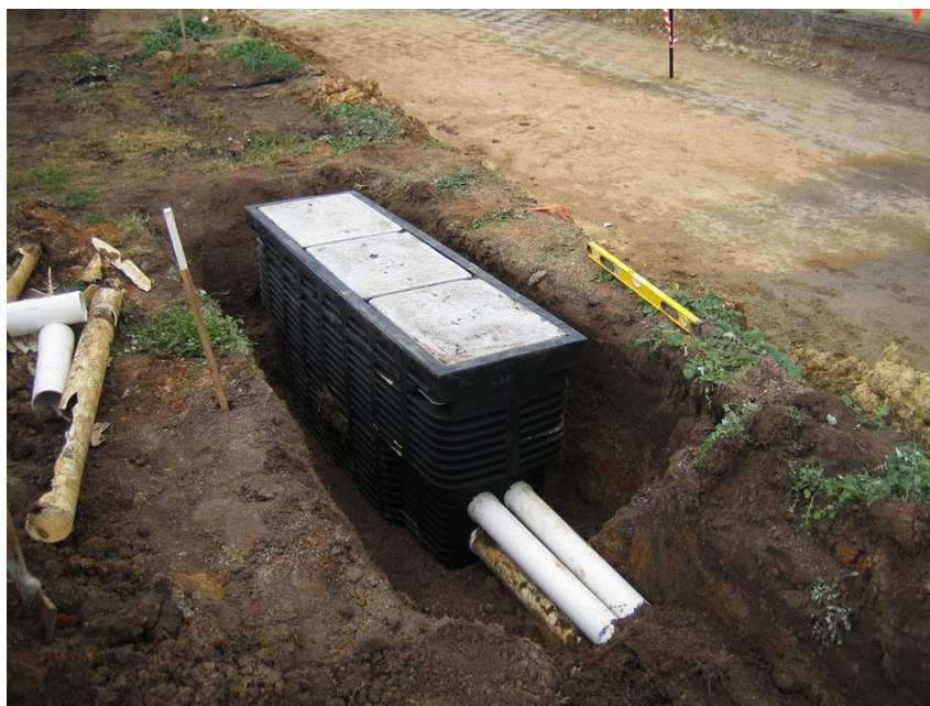
Figure 5-5| "9 Pit" with multiple P100 conduits being installed
