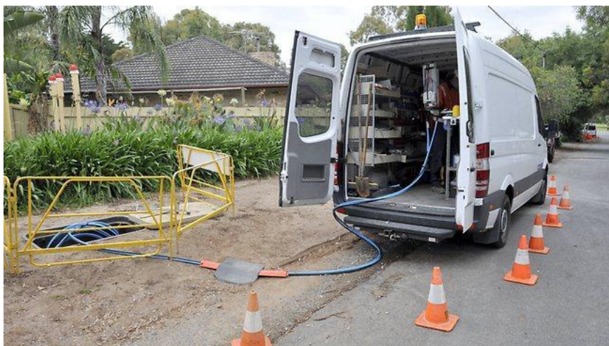
Figure 5-6 | Splicing Van Accessing a roadside pit
