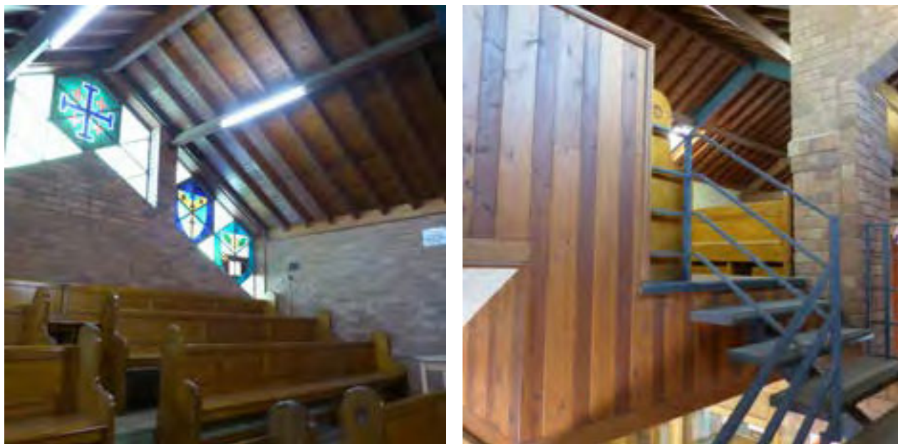
Figures 31 and 32 | Rear section of the early 1960s gallery (left); detail of stair providing access to the gallery (right).
