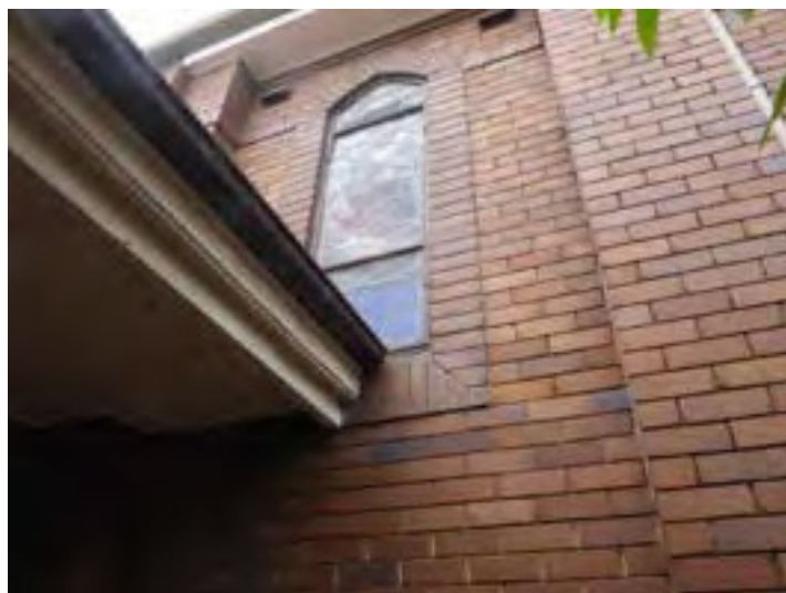
Awkward junction between the Rectory roof and the Church chancel
