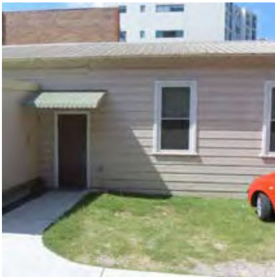
Figures 44 and 45 | Rusticated timber weatherboards and recent windows on the northern side of the Hall (left); skillion roofed northern section of the Hall. The difference in roof level between the original section of the Hall (circa 1926) and the later eastern addition is clearly apparent, as is the differing condition of roof linings.
