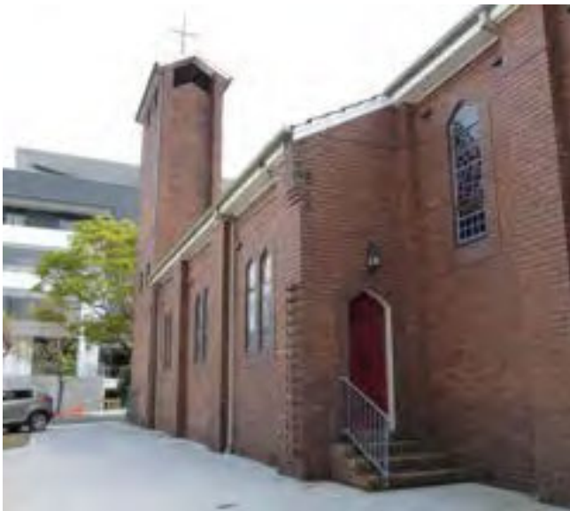
Figures 18 and 19 | Left: Simplified elements along the sides of St Paul's reflect the lingering influence of Gothic architecture, here suggested by the shallow pointed arches of window and door openings and the regularly spaced brick piers, which recall buttresses. The early 1960s tower takes the simplification of Gothic architecture even further. Corbelling at gable ends is also visible. The projecting bricks await the construction of screens that formed part of McPherson's original scheme. Right: the polygonal apse of St Paul's framed by the Vestry and the Rectory. The high band of windows is emphasised by the soldier course below the fascia board and projecting string courses above and below it.
