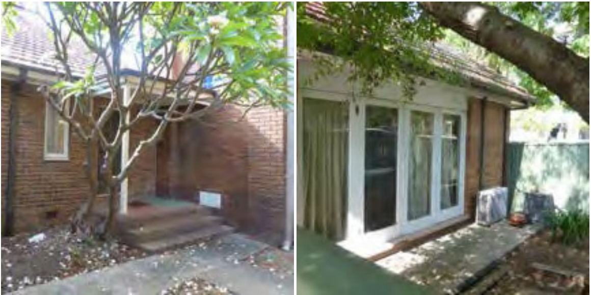
Figures 37 and 38 | The main entrance to the Rectory is on its western side, adjacent to St Paul's Church and distinguished by a relatively generous porch with a simple flat roof supported off a timber post (left); French doors on the north side of the Rectory (right).
