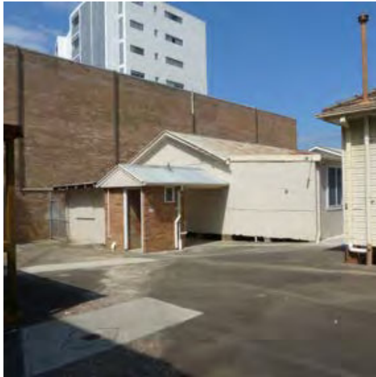
Figure 46 | Circa 1960s toilet and storeroom at the eastern end of the Hall. The toilet block is connected to the Hall by an extension of its metal clad gabled roof.
