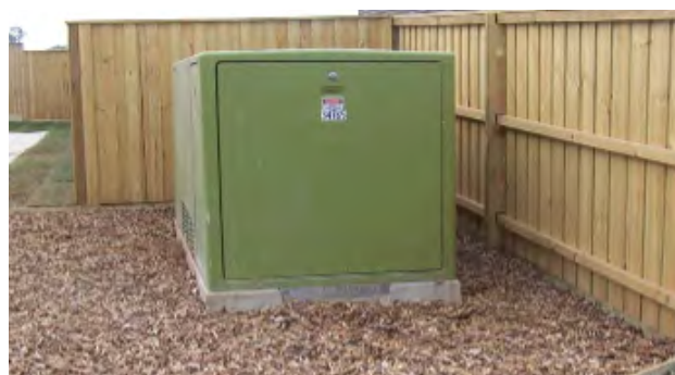
Correctly maintained padmount surrounding area
