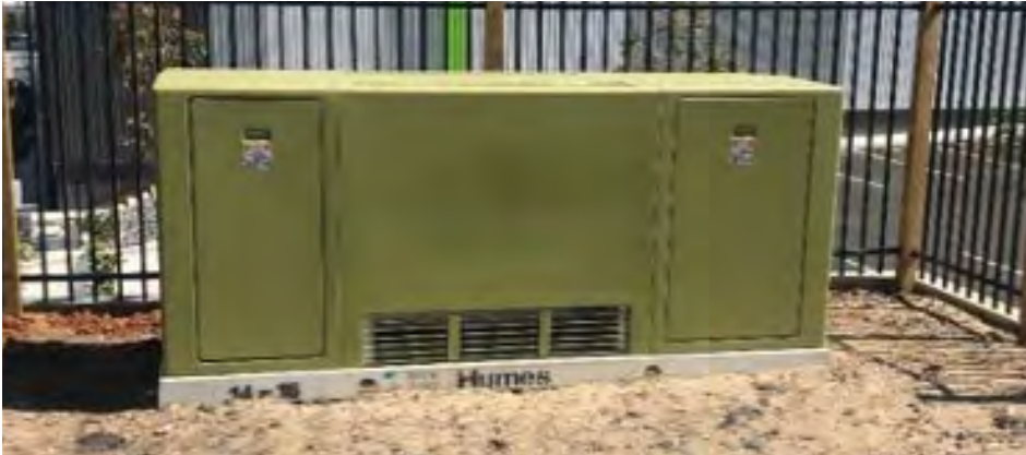
Example of a padmount substation
