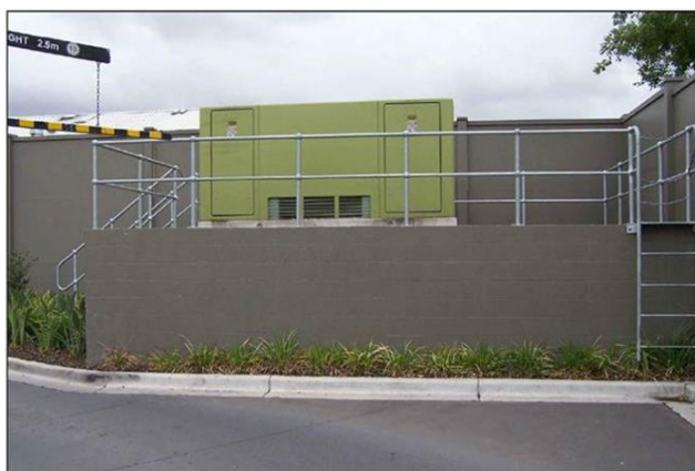
Figure 51 - Example substation raised above 1:100 flood level
