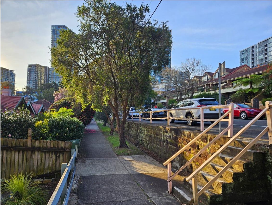
Figure 2 The Nicholson Street Site looking north towards St Leonards
