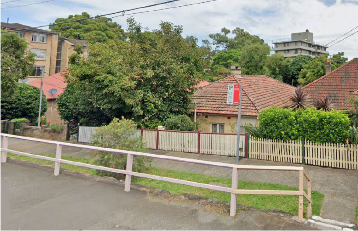
Figure 9 10-storey tower to the west of the site
