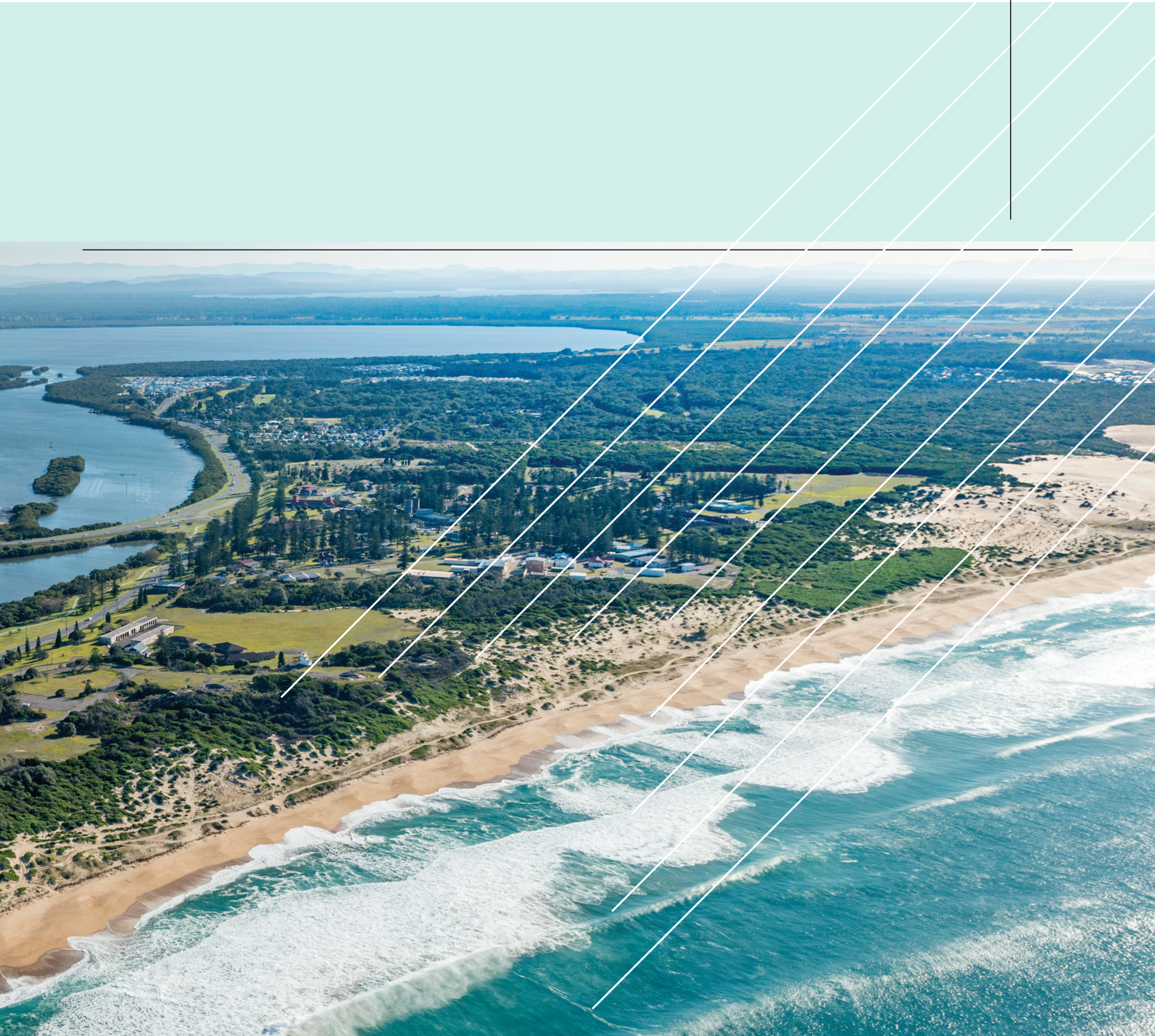
Stockton Bridge looking north towards Fullerton Cover. Credit: Defence Housing Australia.
