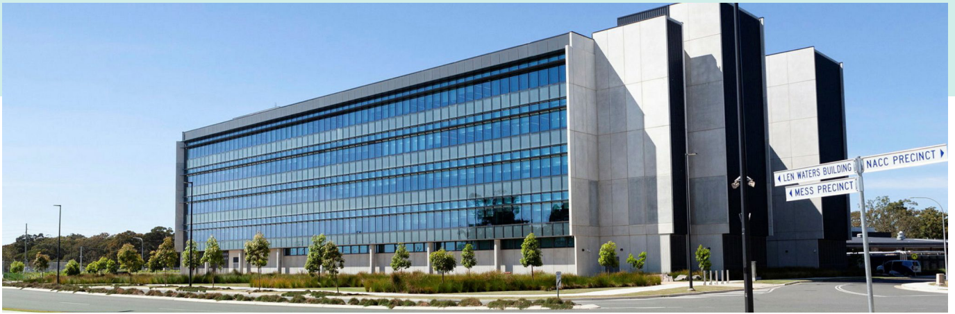
Figure 26: Len Waters Building at RAAF Base Williamtown. Credit: Department of Defence
