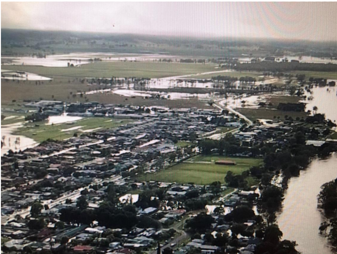
Figure 7.2 Casino Primex site (middle left) and Bruxner Highway (middle right) February 2022 flood
