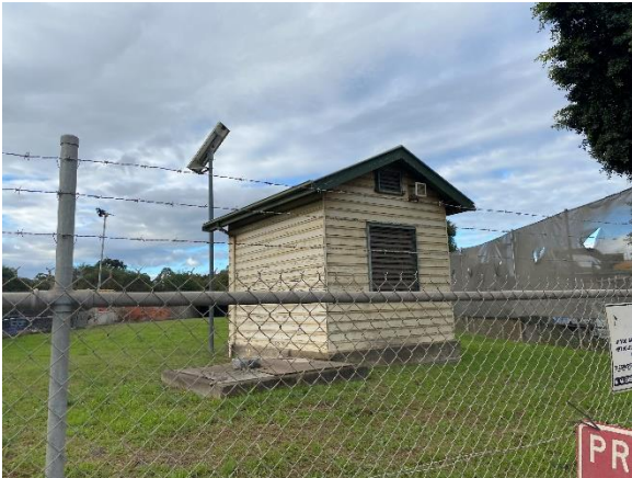
Figure 5 Valve house at 41 Grand Ave
