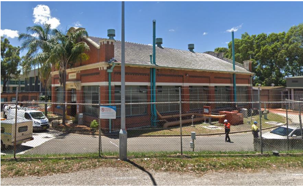
Figure 8 SP0067 Sydney Water Pump Station
