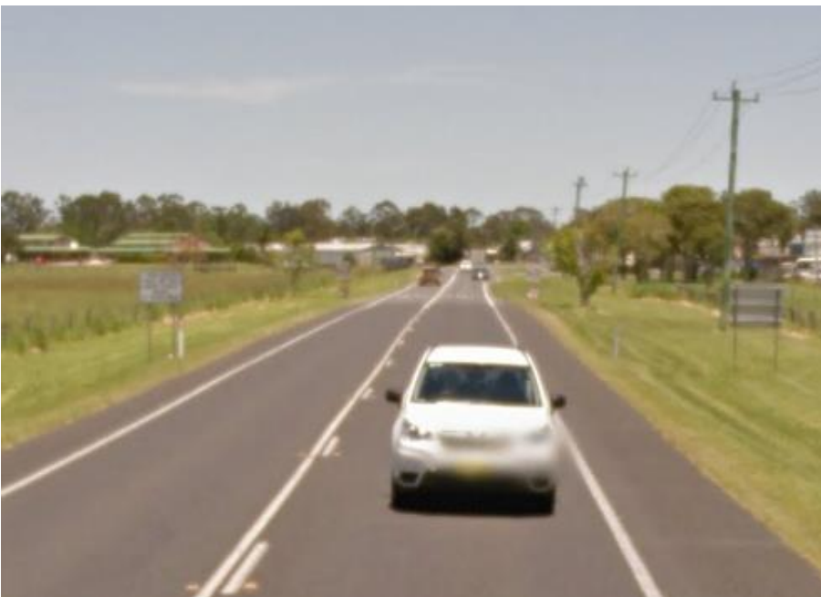
Figure 2.4 Bruxner Highway in proximity to the Johnston Street industrial area
