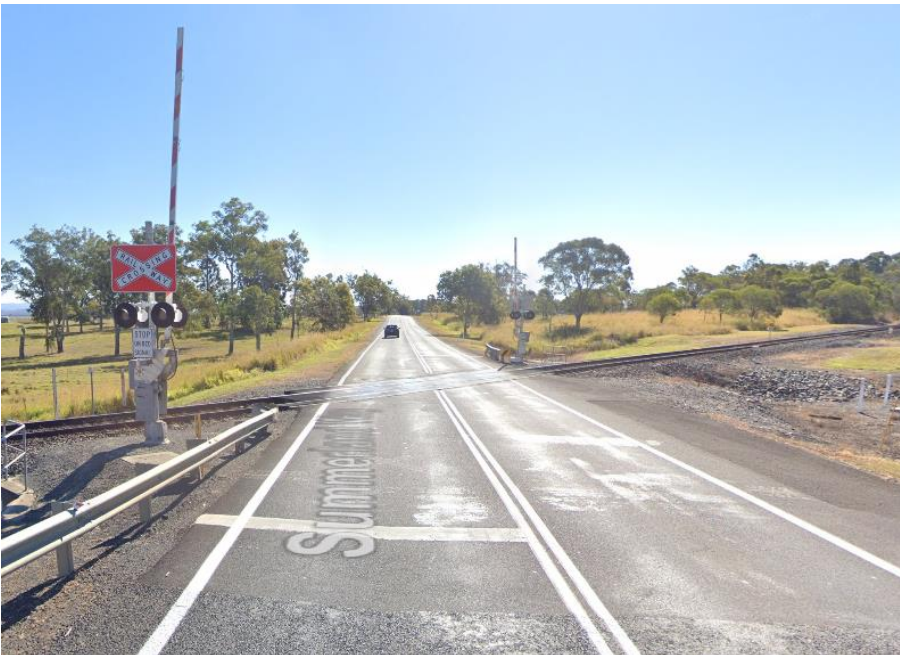
Figure 2.3 Rail level crossing at Summerland Way
