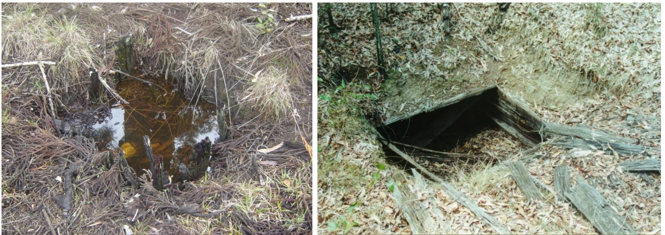
Figure I-16.3 Examples of timber lined wells
