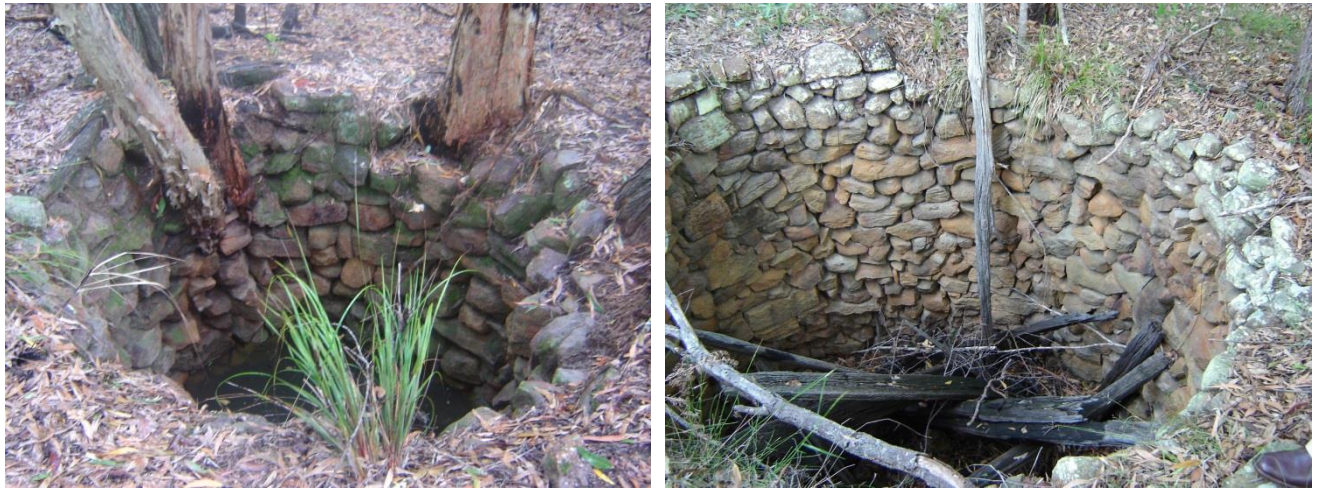
Figure I-16.2 Examples of stone lined wells
