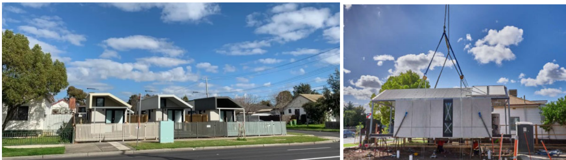
Figures 5 & 6: Photographs of Launch Housing tiny homes development on VicRoads sites – relocatable tiny homes as TSA. Fitting with low-density character of existing suburb. https://www.launchhousing.org.au/harris-transportable-housing-project
