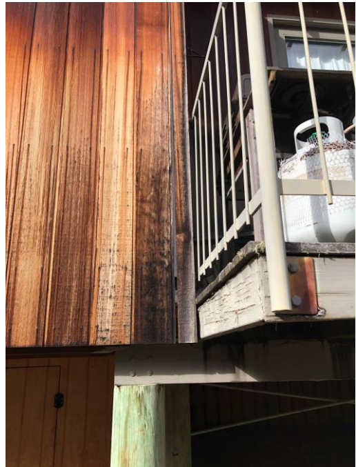
Figure 4: Photo showing the deteriorated cladding, decking boards and decking fascia requiring replacement
