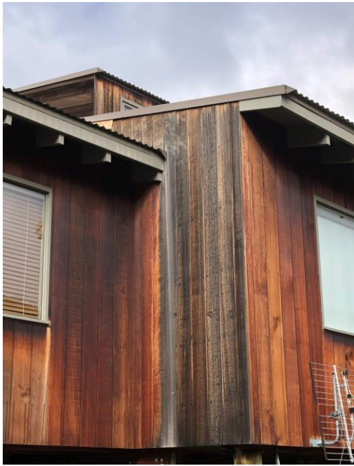
Figure 3: Photo showing the deteriorated cladding requiring replacement
