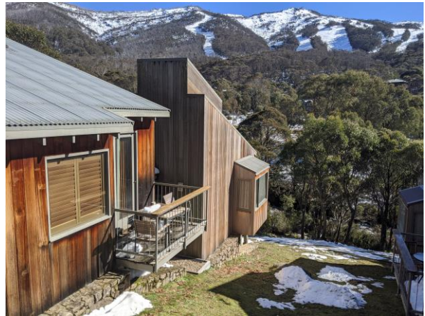
Figure 8: Photo of a cabin with the original cladding requiring replacement and further back a cabin recently re-cladded
