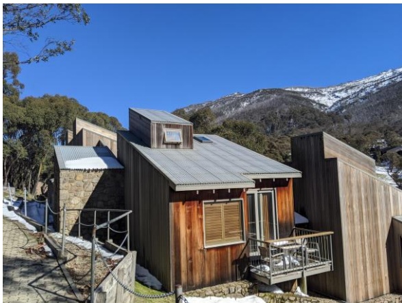
Figure 5: Photo of the lantern façade cladding requiring replacement
