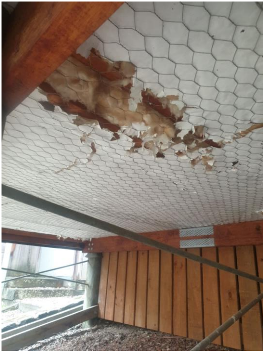
Figure 7: Photo of the underside of the cabins to be lined with metal soffit lining
