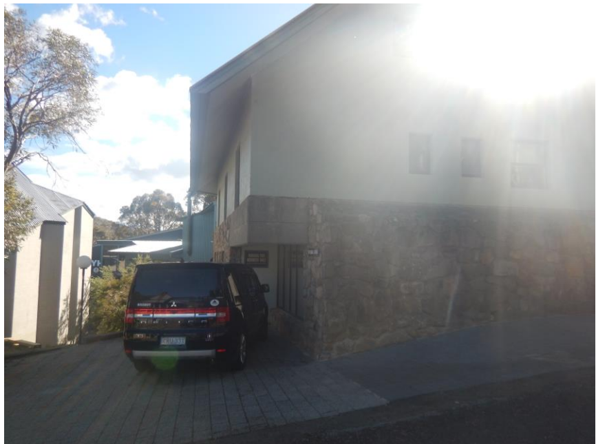
Figure 2: Photo of the southwest elevation and western lower carpark
