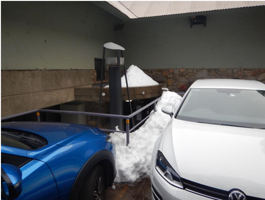
Figure 12: Snow deposition from the roof valley onto the main entrance area
