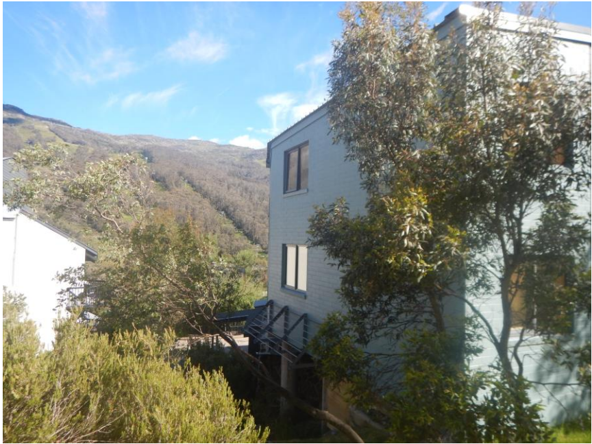
Figure 5: Photo of Kiama Lodge to the north-east
