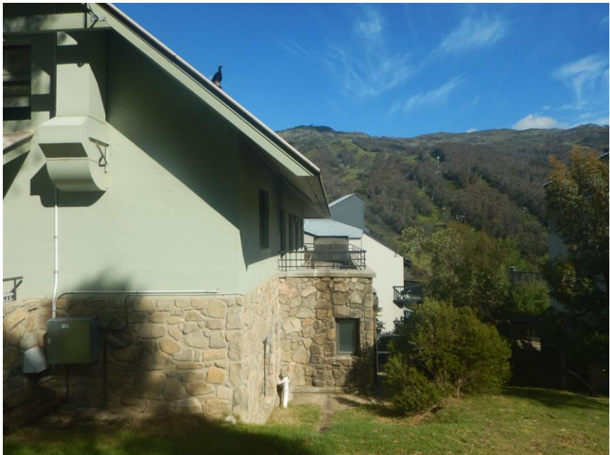
Figure 4: Photo of the south-east elevation of the lodge
