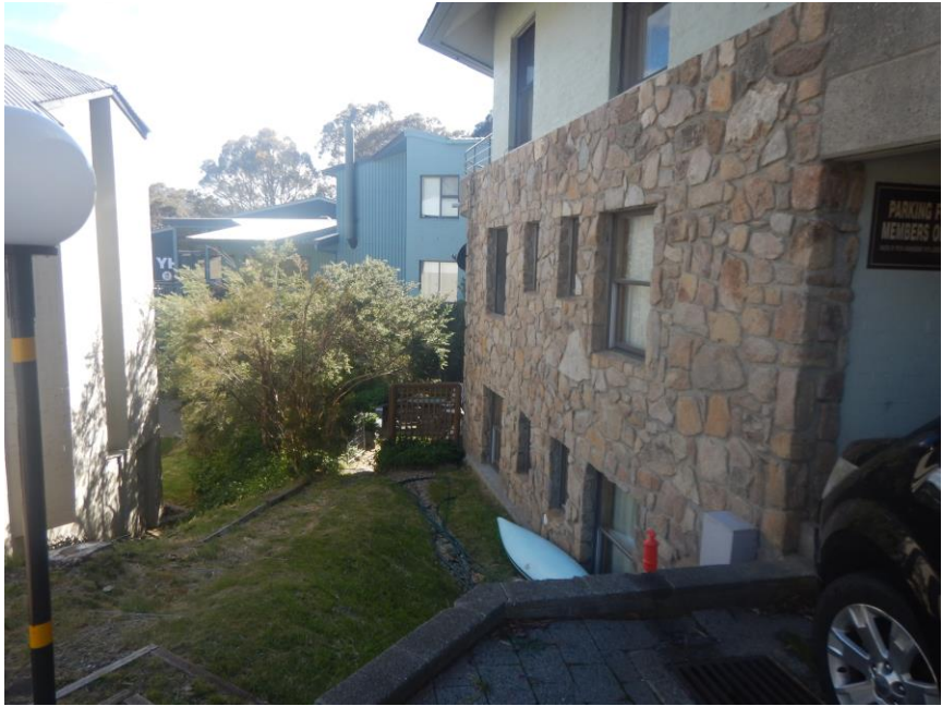
Figure 3: Photo of the north-west elevation of the lodge
