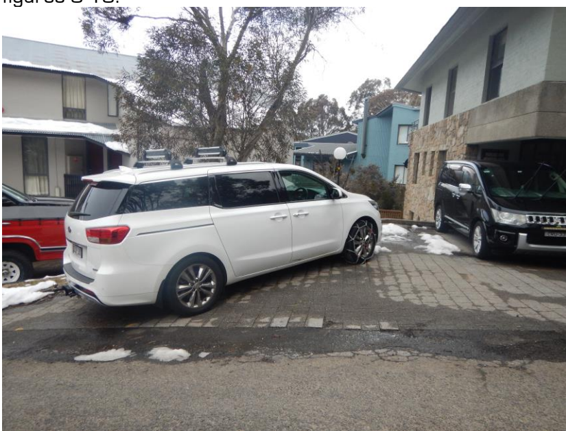
Figure 9: Car park at the western side of the building is subject to snow deposition from the roof above
