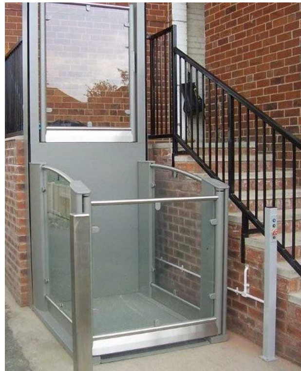
IMAGE OF TYPICAL EXTERNAL PLATFORM LIFT INSTALLATION
