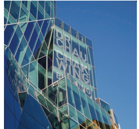
Figure 1.6.5 / Dr Chau Chak Wing Building
