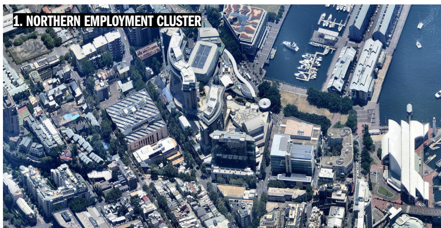
88 / Aerial view of the northern employment cluster within the peninsula, Nearmap 2020
