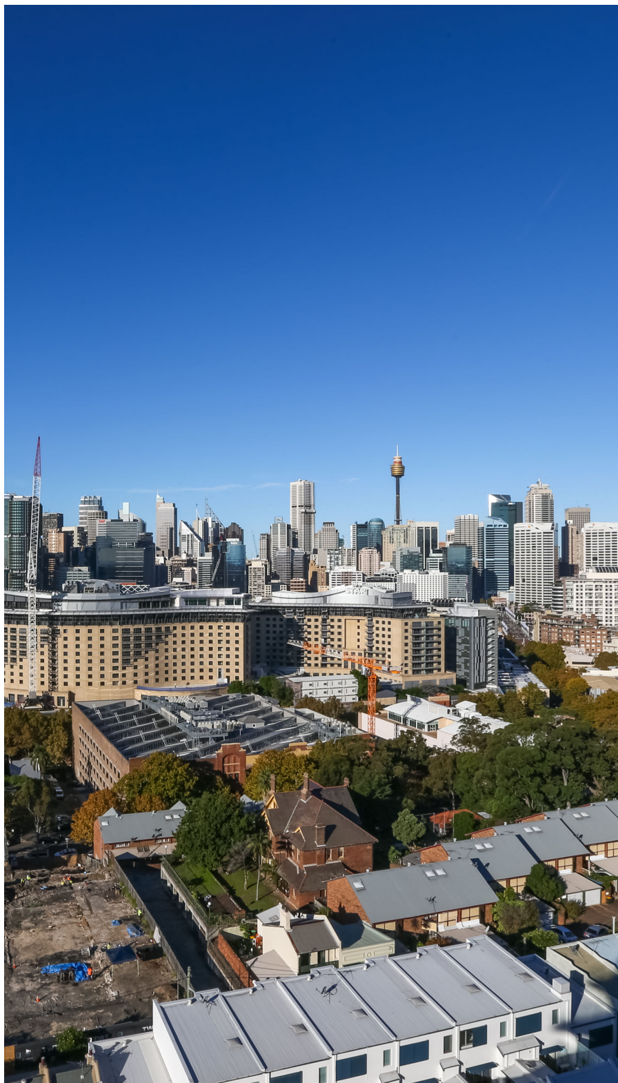
92 / View looking over Pyrmont Peninsula towards Sydney CBD showing a variety of building typologies on varying lot sizes, City of Sydney 2019
