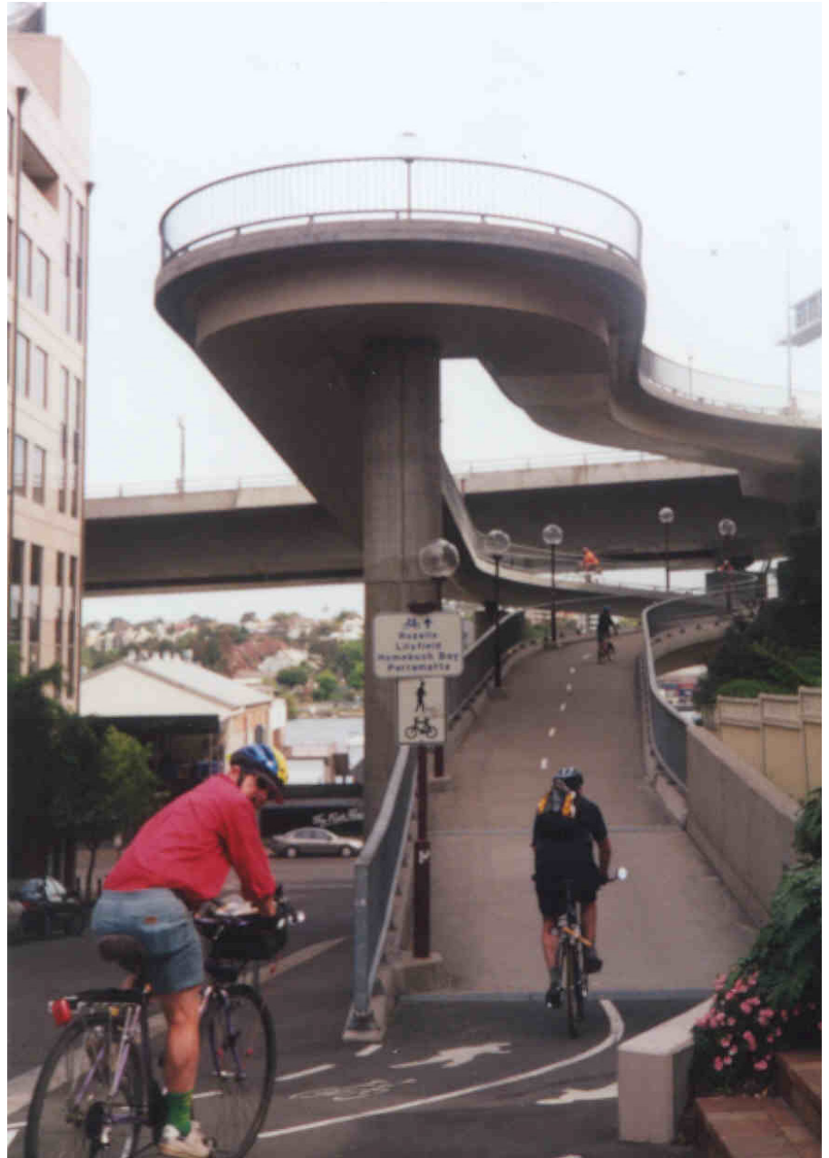
84 / View of pedestrian and cycle access ramp to Anzac Bridge on Quarry Master Drive
