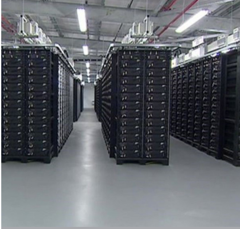
An example of grid scale battery storage
