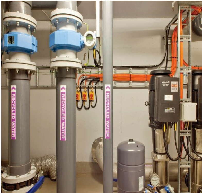
Recycled water infrastructure
