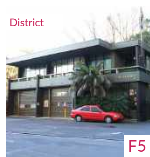
NSW Fire Brigade Station - The Rocks
