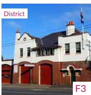
NSW Fire Brigade Station - Glebe
