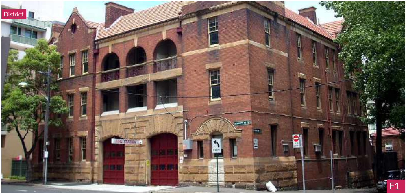
NSW fire brigade station - Pymont
