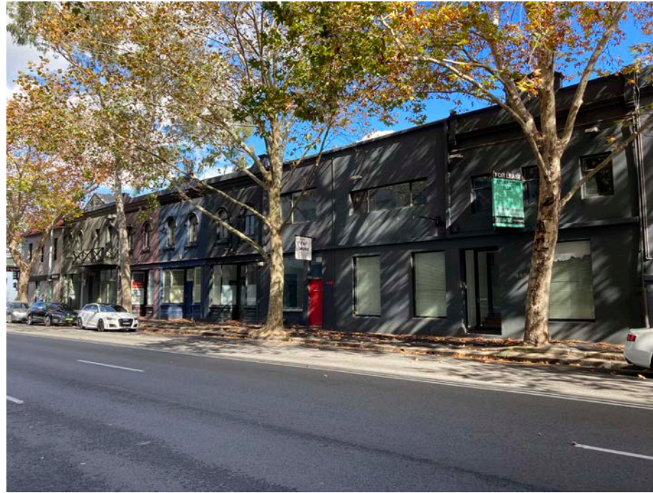
View of western side of Harris Street.
