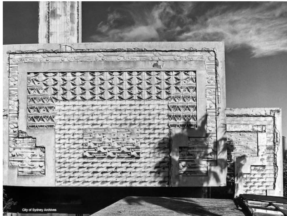
Griffin Incinerator stack detail. (Source: City of Sydney Archives)
