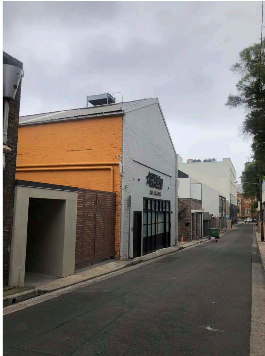
View of rear of properties fronting Harris Street from Hackett Street facing south.
