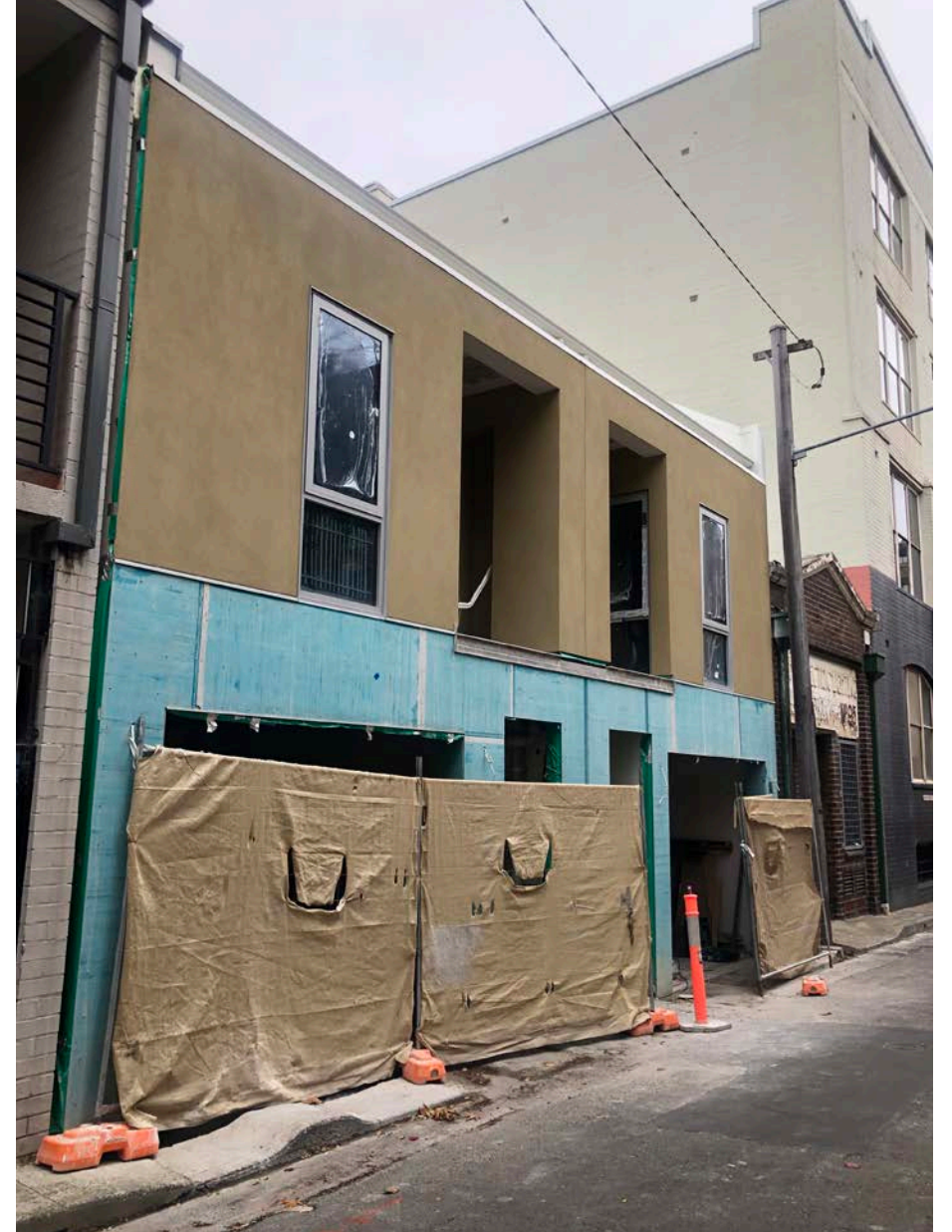
View south of Hackett Street showing new development adjacent to a s170 listed substation.
