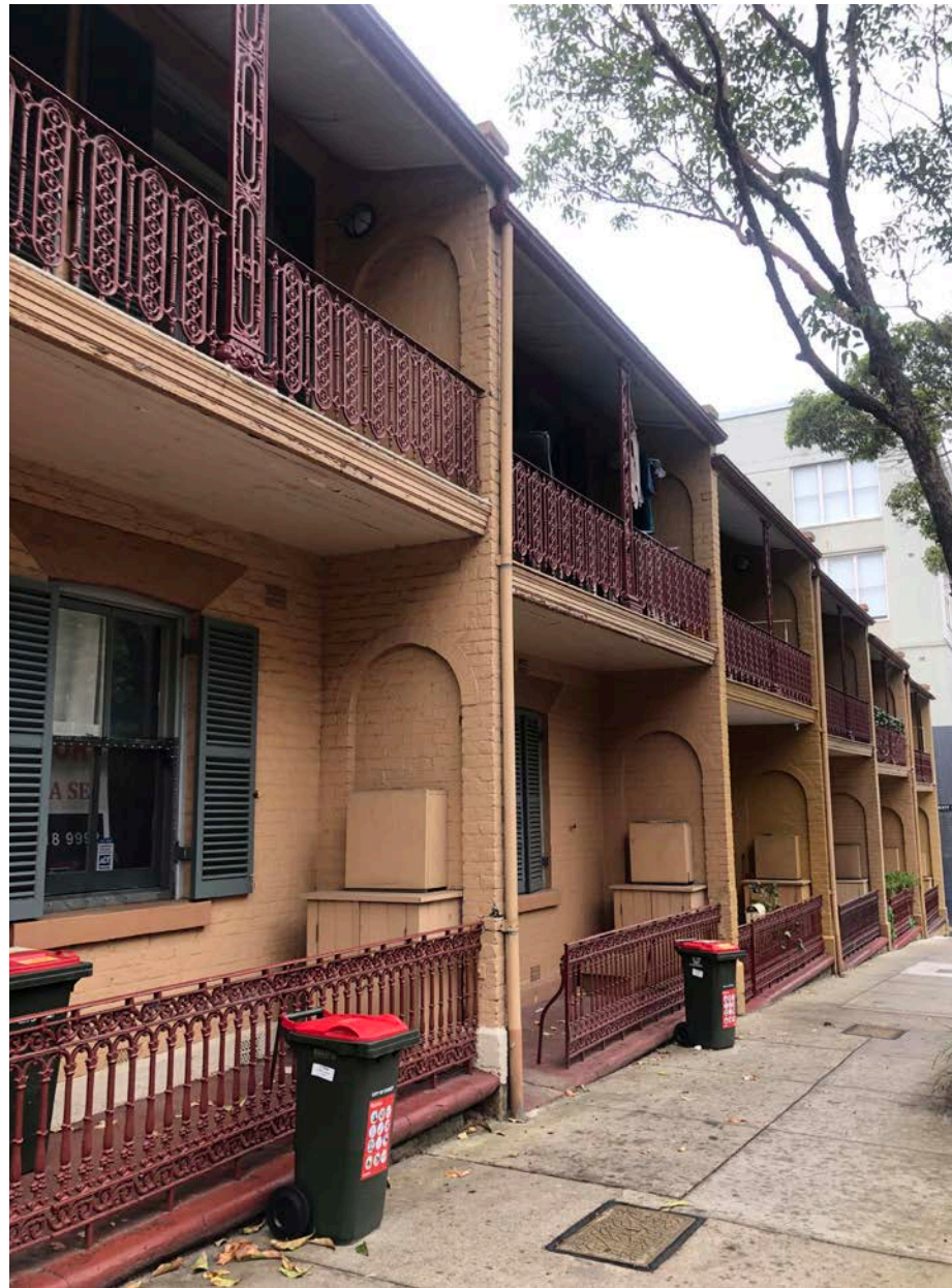
View of terrace houses fronting Mary Ann Street.
