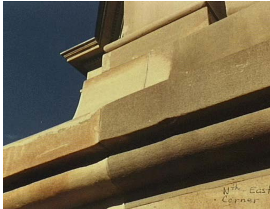
Restoration of the Sydney Town Hall clock tower, 1982. (Source: City of Sydney Archive)
