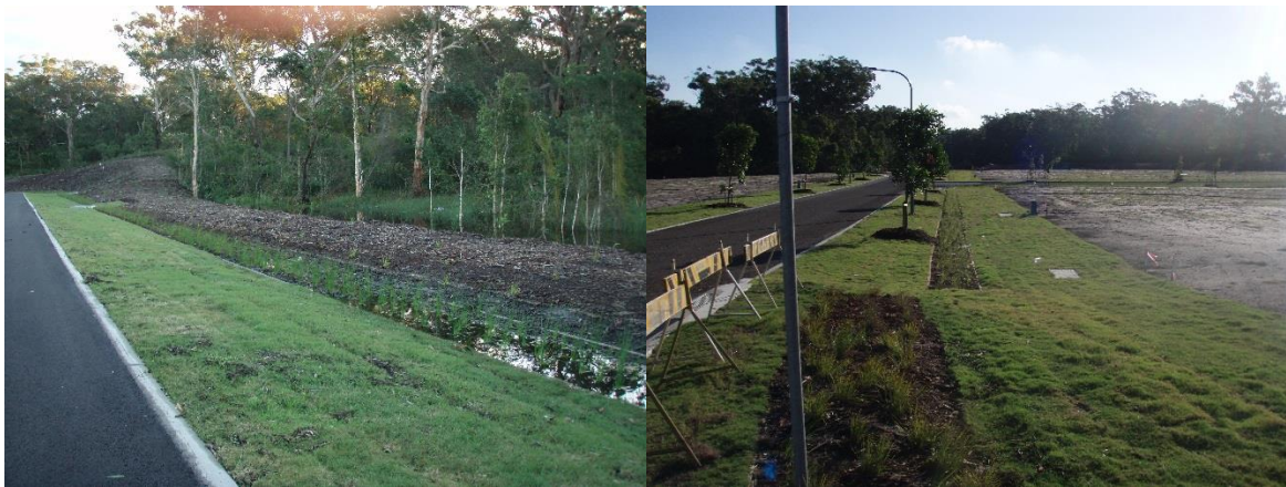
Figure 7-5 Grassed roadside filter strips
