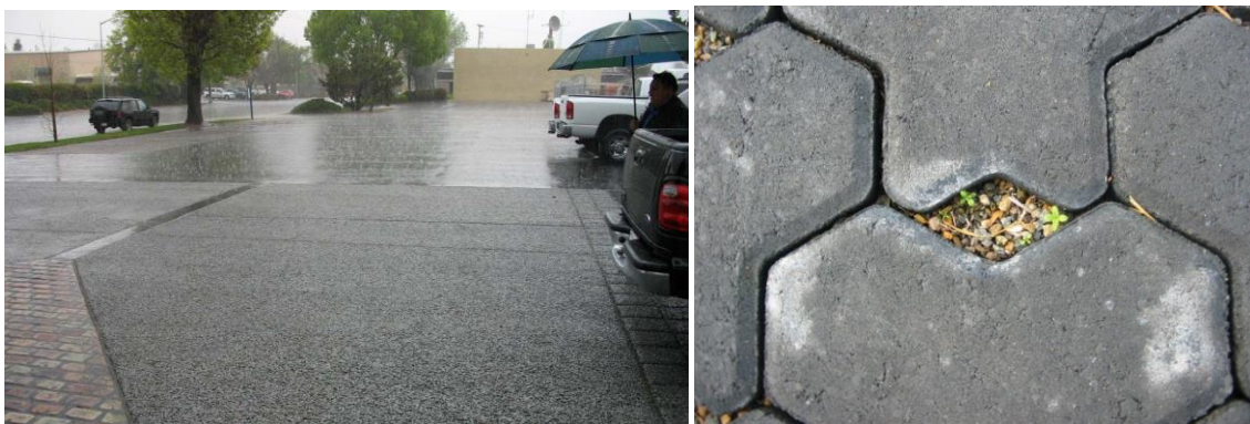
Figure 7-4 Pervious concrete (LHS) and permeable pavers (RHS)
