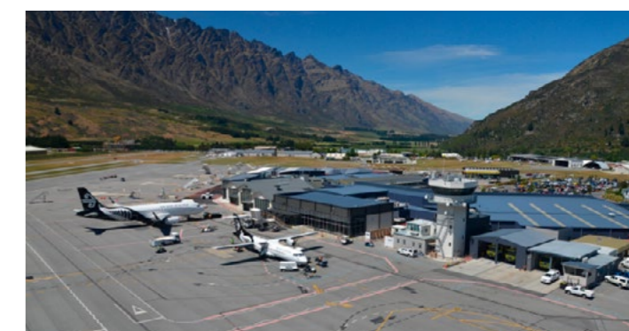
International Airport at Queenstown
