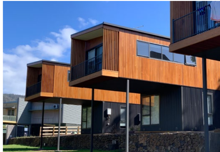
Contemporary accommodation is of high quality Source: Michael McKeown, 2021
