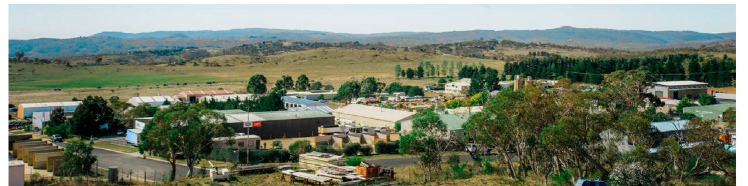
Leesville industrial area, South Jindabyne, about 4km by road from the town centre and away from other built up areas
