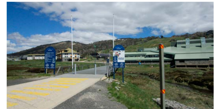
Bridge across river at Perisher Village
