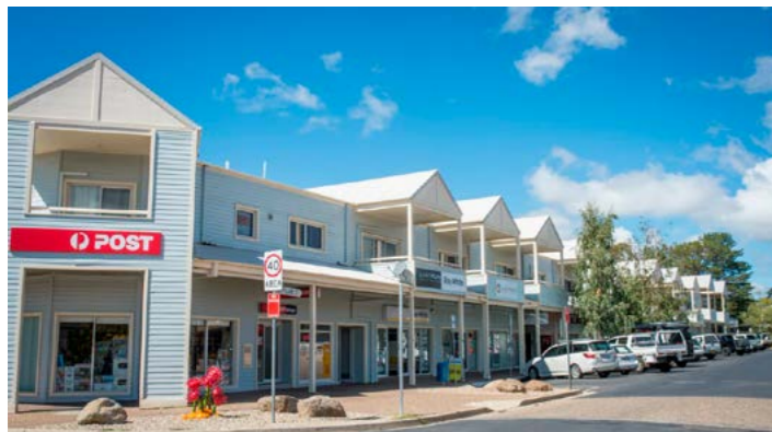
Well-scaled development with positive street interfaces in Gippsland Street
