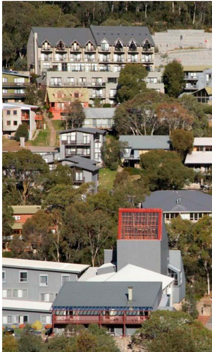
Thredbo Centre (West) with many opportunities for renewal and redevelopment of older tourist accommodation over time
