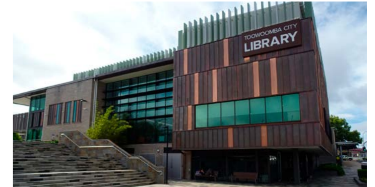
Example of a contemporary library / civic building
