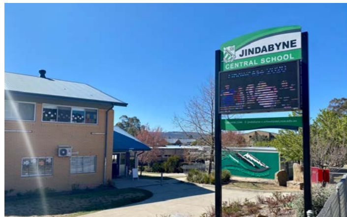
Jindabyne Central School. Some buildings are recently built and may be worthy of adaptive re-use
