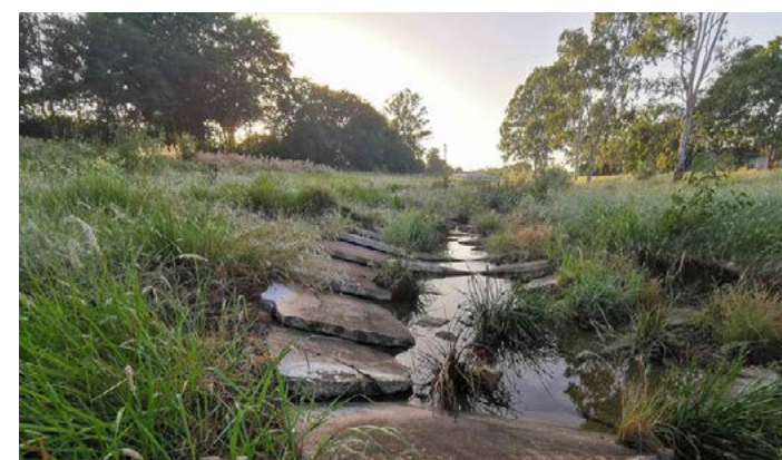
Reusing the former concrete lined drain
