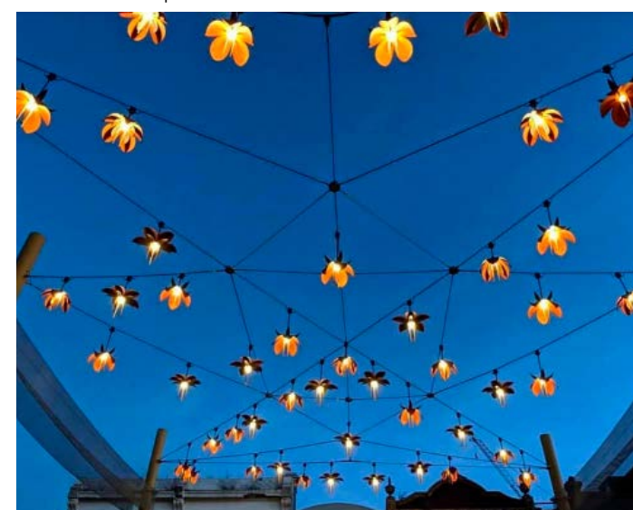
Bespoke catenary lighting assembled with tension cabling and post construction suitable for the new town square and other smaller spaces.
