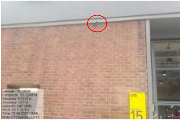
Photograph 5: Showing the potential breather vent pipe associated with the potential UST.
