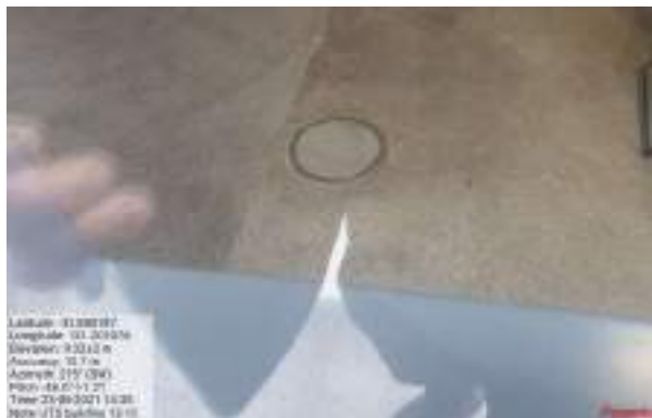
Photograph 3: Showing what appeared to be a former UST fill point, which appeared to have had the metal gatic cover removed and filled with concrete. The approximate UST location is shown on Figure 2.
