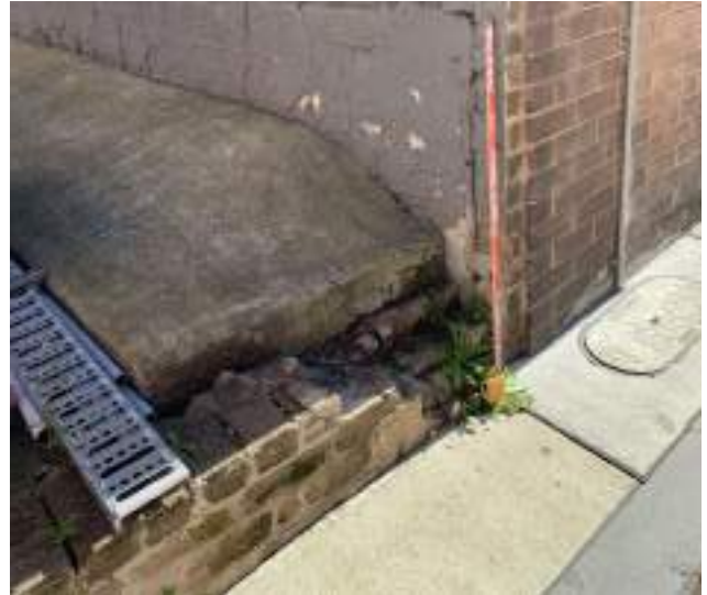
Figure 26 – Brick foundations of the former commercial building abutting the shopfront at 644-644A Harris Street. Note the concrete slab as evidence of the surface level of this former structure, which is approximately 50cm above the existing carpark level.
