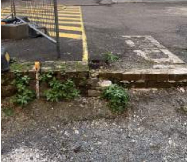
Figure 25 – Brick foundations of the mid-20 th century commercial building which occupied 634-642 Harris Street.
