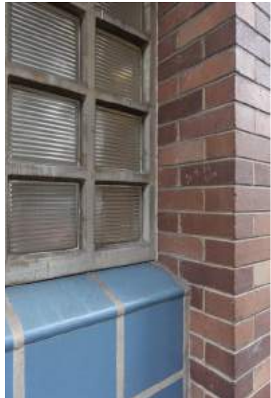
Figure 2.3.22: View of the 'Plummer Crete' windows atop tiled infill walls.
