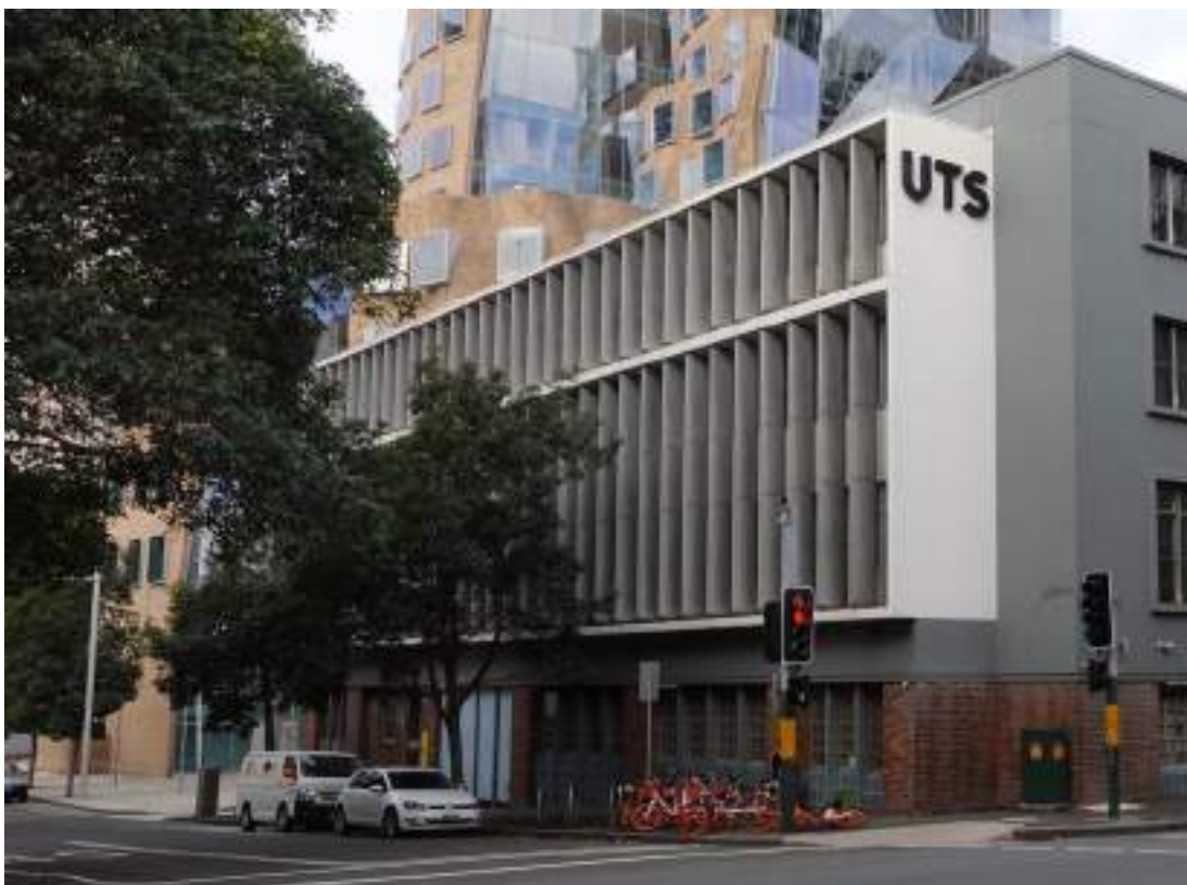
Figure 2.3.17: Mary Ann Street Elevation showing the cantilevered framed concrete box with aluminium louvers.
