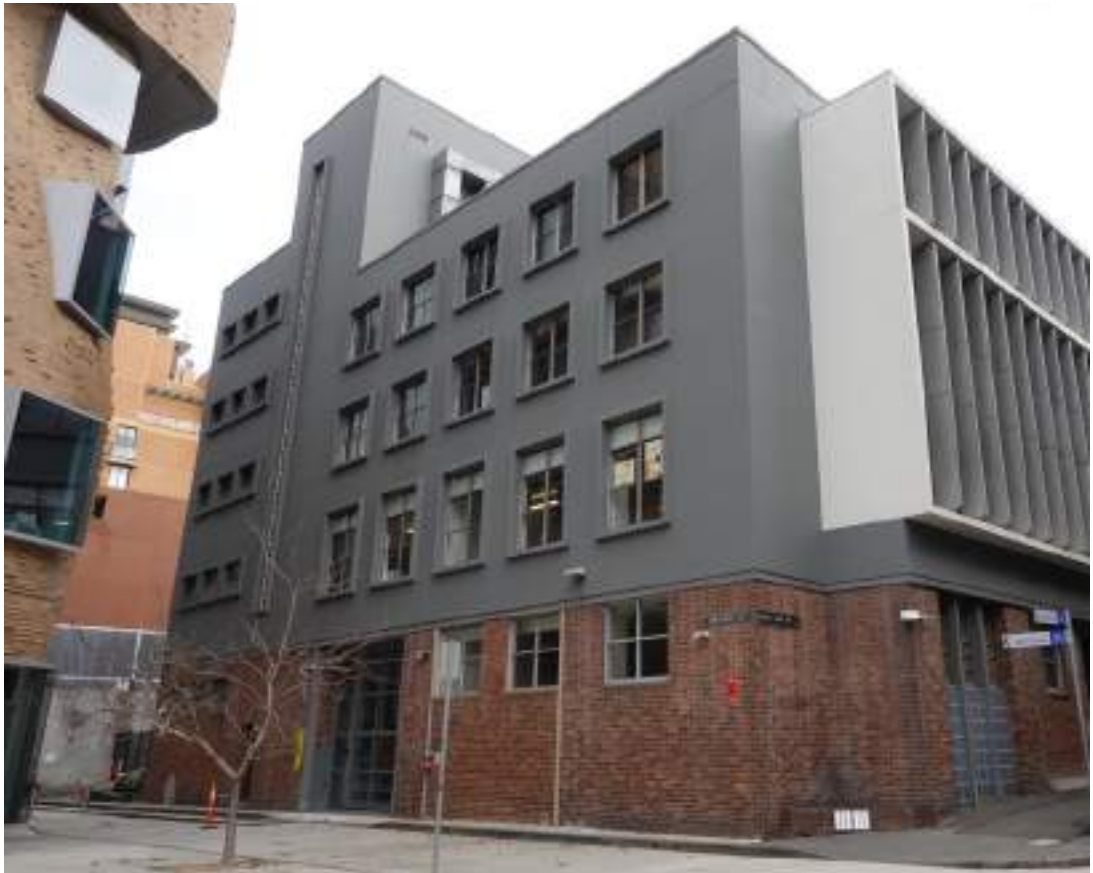
Figure 2.3.23: Omnibus Lane elevation showing the former entry bays to the loading dock. One of the bays is seen with an aluminium framed sectional glass and the bay to its right has been filled in with rendered brick wall with clerestory windows.
