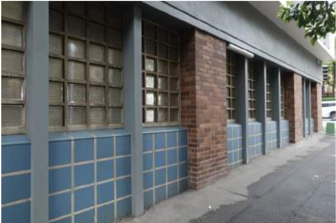
Figure 2.3.20: View looking south west along Mary Ann Street Elevation showing the recessed bays with the 'Plummer Crete' windows (with glass blocks).
