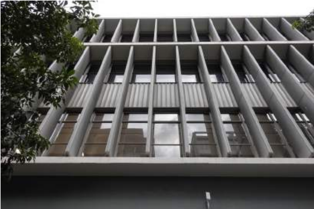
Figure 2.3.19: The concrete framed box with profiled aluminium spandrels and aluminium windows behind the aluminium louvers.
