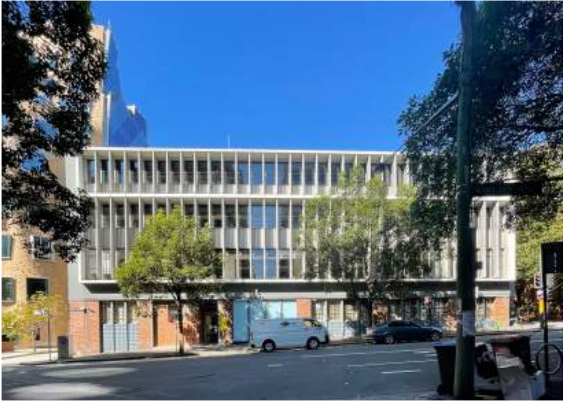
Figure 2.3.18: The Mary Ann Street Elevation showing the cantilevered framed concrete box with aluminium louvers.
