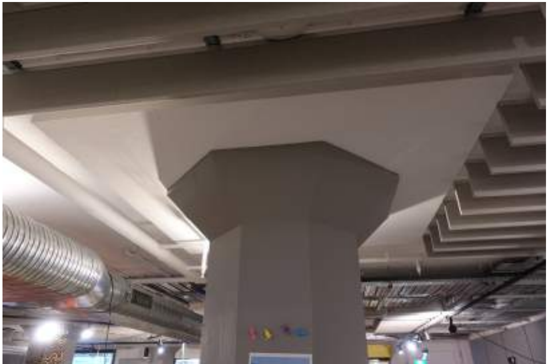
Figure 2.3.42: A concrete column with mushroom head supporting splayed beam and exposed concrete ceilings.
