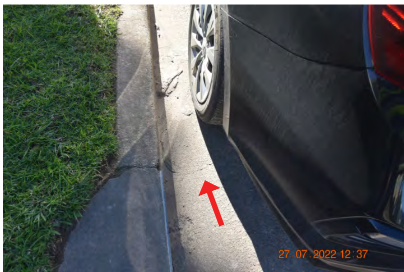
Figure: 0464 Fine cracking in the gutter. | CHANGE: None
