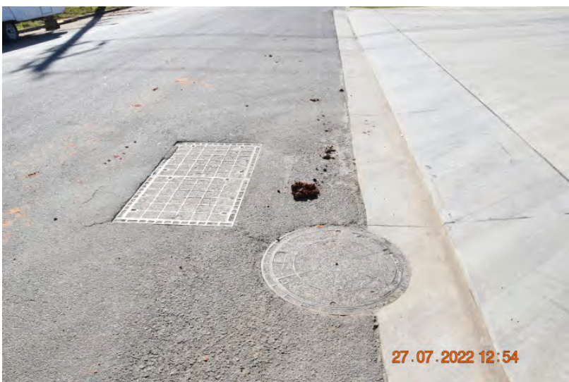
Figure: 0524 Slight cracking in the paving. | CHANGE: None
