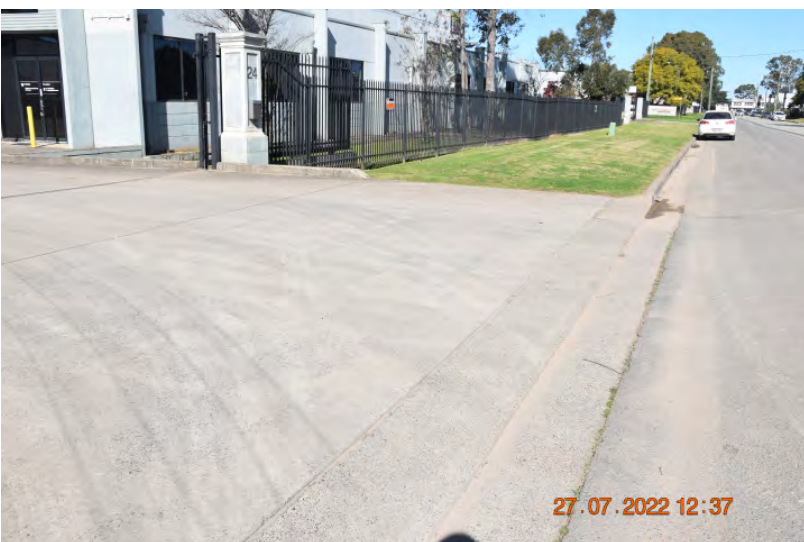
Figure: 0467 Scoring in the paving. | CHANGE: None
