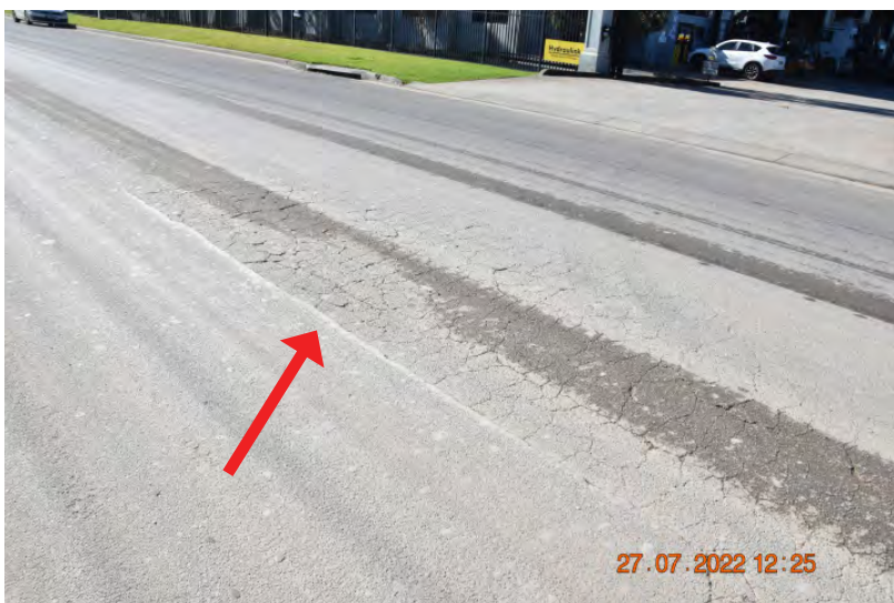
Figure: 0425 Fine alligator cracking in the paving. | CHANGE: None
