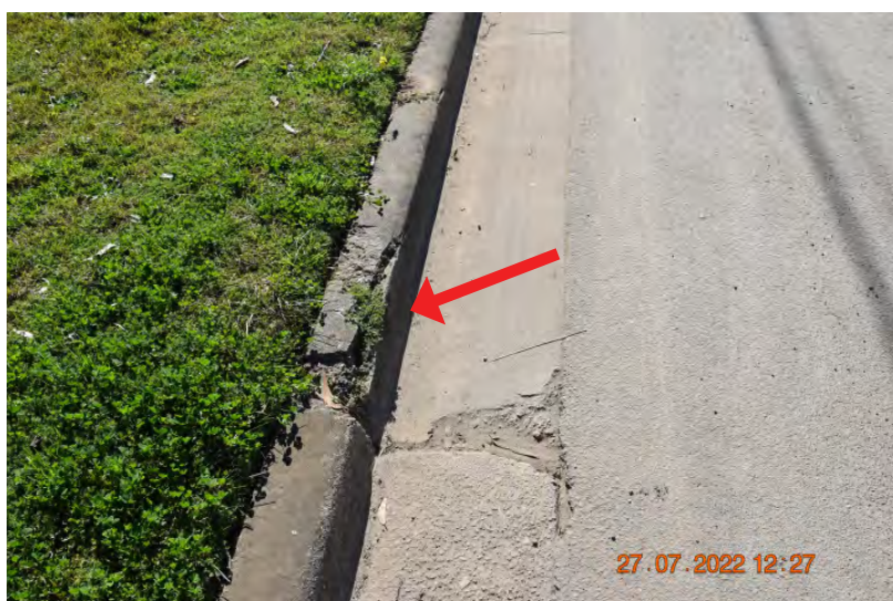
Figure: 0431 Chipping in the kerb and gutter. | CHANGE: None
