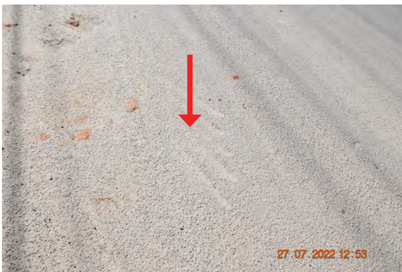
Figure: 0518 Scoring in the paving, looking to the north. | CHANGE: None
