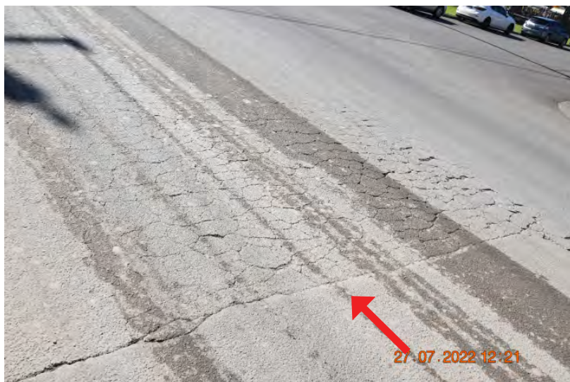
Figure: 0403 Slight cracking in the paving. | CHANGE: None
