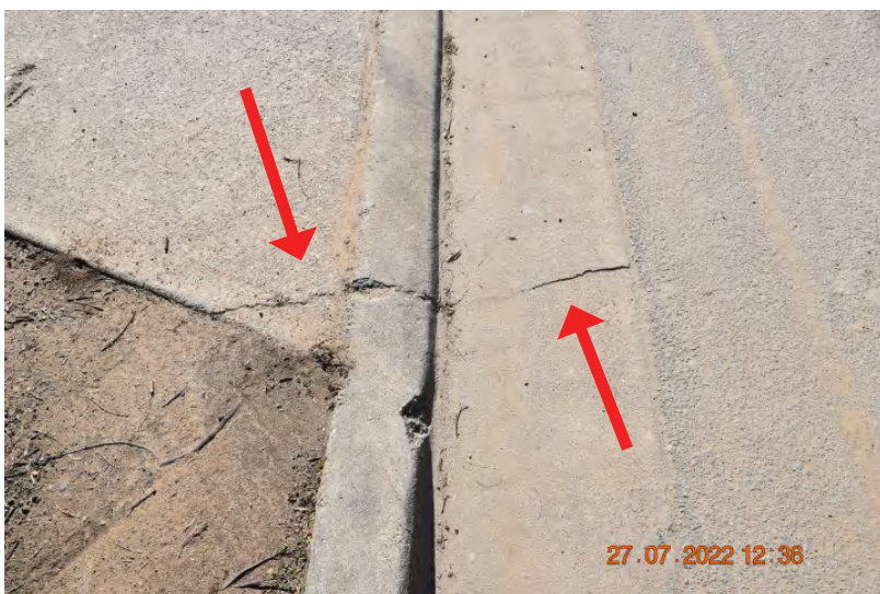
Figure: 0461 Fine cracking in the crossover. (462-463) | CHANGE: None
