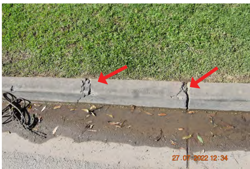
Figure: 0449 Slight cracking in the kerb and gutter. | CHANGE: None
