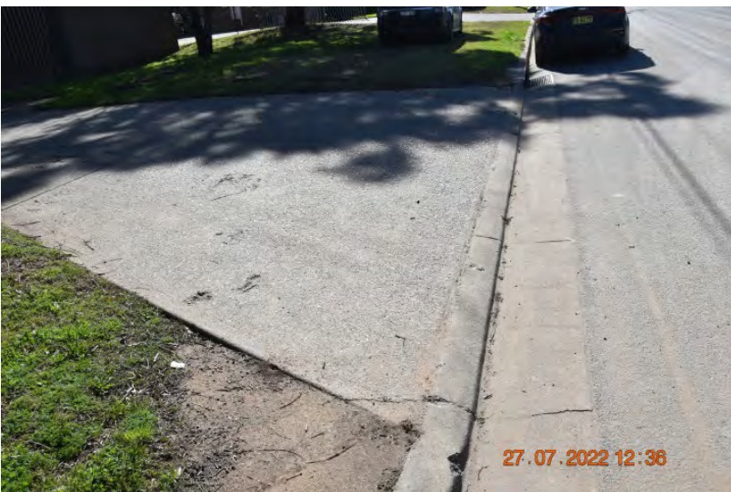
Figure: 0461 Fine cracking in the crossover. (462-463) | CHANGE: None
