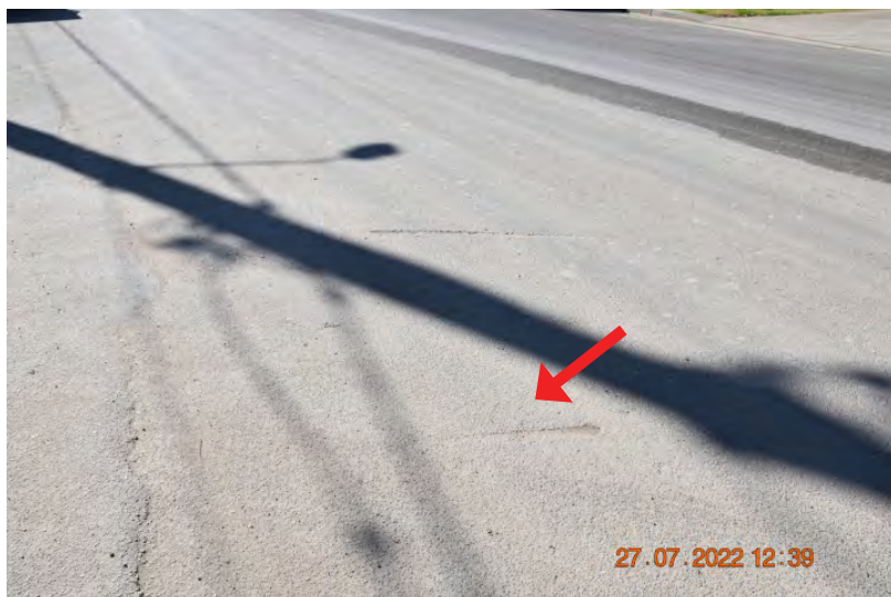
Figure: 0475 Slight cracking in the paving and the crossover. | CHANGE: None
