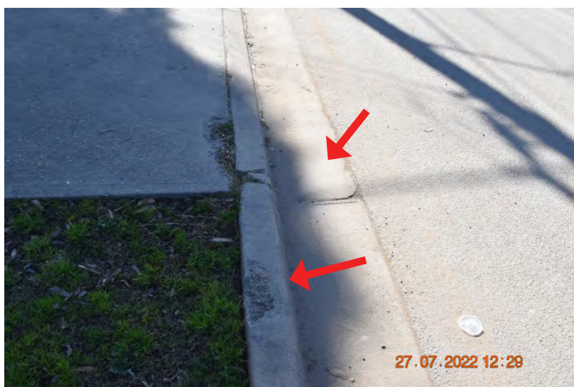
Figure: 0440 Chipping and slight cracking in the crossover. | CHANGE: None
