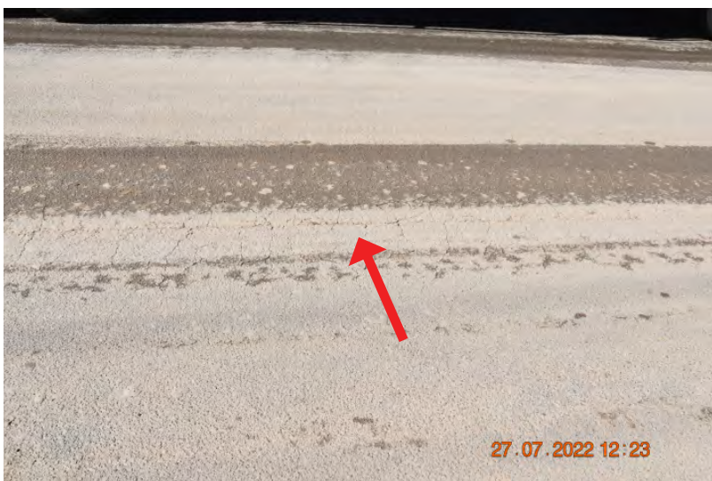
Figure: 0410 Slight separation in the roadway. (RPT FOR FIGURES 411-412) | CHANGE: None
