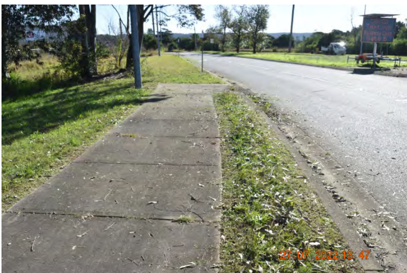
Figure: 0548 Slight cracking in the kerb and gutter. | CHANGE: None
