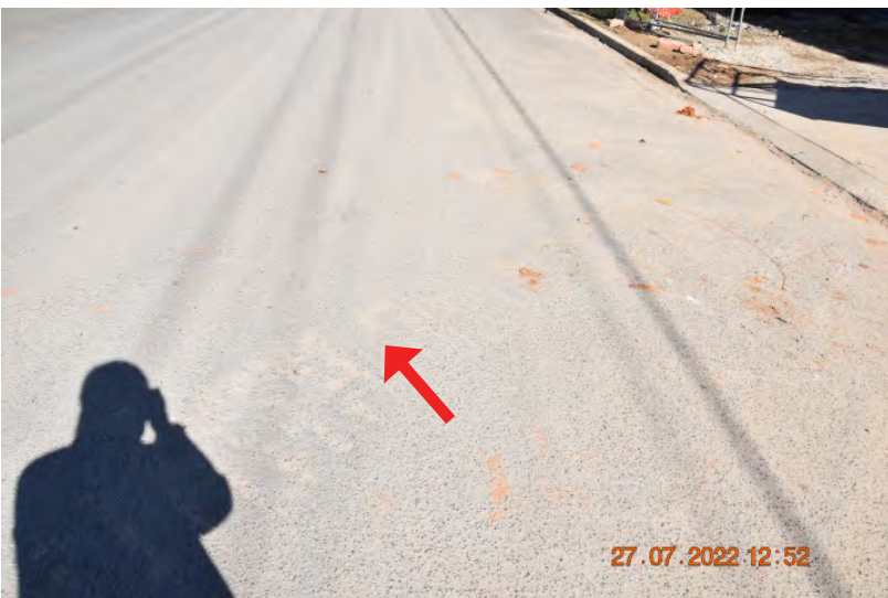
Figure: 0518 Scoring in the paving, looking to the north. | CHANGE: None
