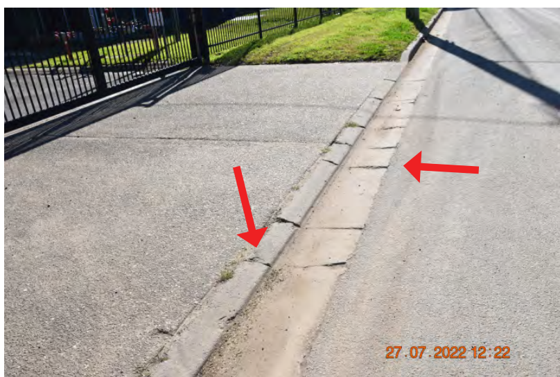
Figure: 0404 Chipping and slight cracking in the crossover. (RPT FOR FIGURES 405-406) | CHANGE: None
