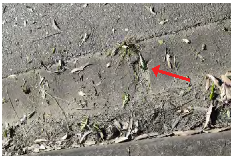
Figure: 0548 Slight cracking in the kerb and gutter. | CHANGE: None
