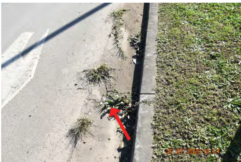
Figure: 0590 Slight cracking and chipping in the kerb and gutter. | CHANGE: None
