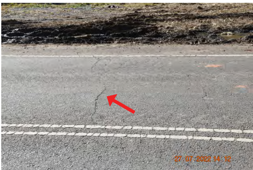
Figure: 0641 Slight cracking in the paving. (RPT FOR FIGURES 642-643) | CHANGE: None
