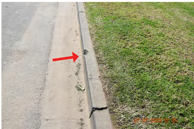
Figure: 0454 Fine cracking in the kerb and gutter. (RPT FOR FIGURES 455-456) | CHANGE: None
