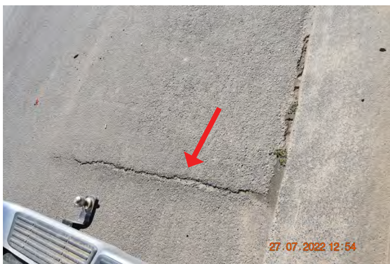
Figure: 0524 Slight cracking in the paving. | CHANGE: None
