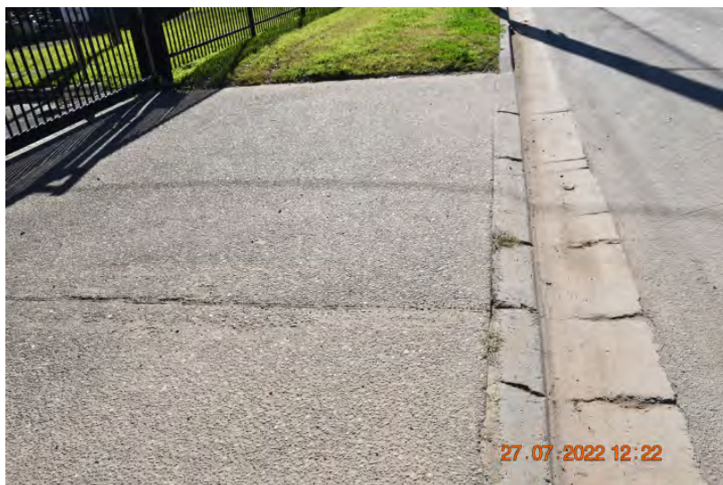
Figure: 0406 Fine cracking in the kerb and gutter. | CHANGE: None
