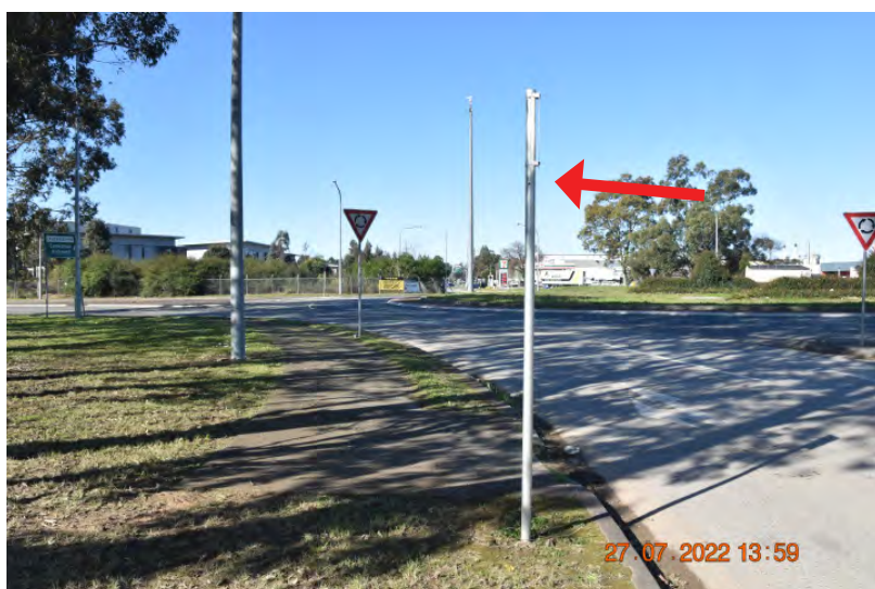
Figure: 0566 Leaning street sign. | CHANGE: None
