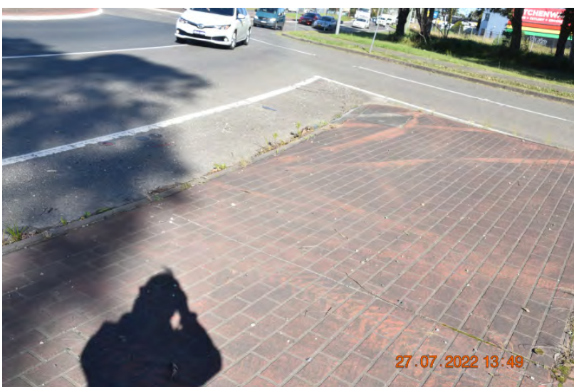
Figure: 0554 Slight cracking in the median strip. | CHANGE: None
