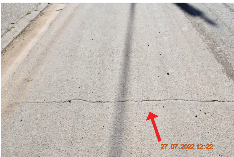
Figure: 0404 Chipping and slight cracking in the crossover. (RPT FOR FIGURES 405-406) | CHANGE: None
