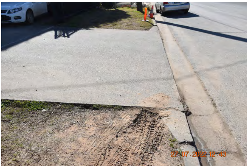
Figure: 0496 Slight cracking and chipping in the kerb and gutter. | CHANGE: None
