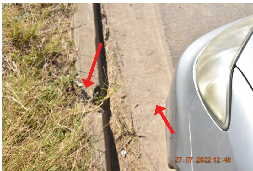
Figure: 0506 Chipping in the kerb. Also showing fine cracking in the gutter. | CHANGE: None
