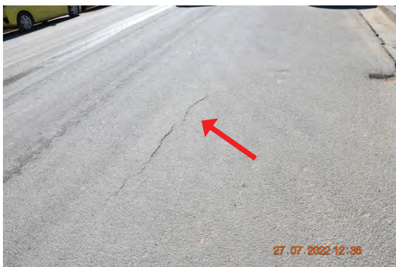
Figure: 0458 Fine cracking in the paving. | CHANGE: None
