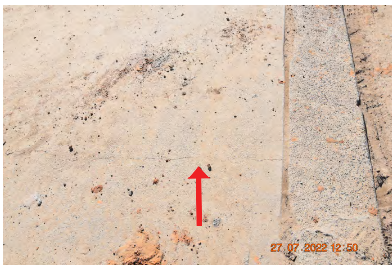
Figure: 0515 Fine cracking in the crossover, looking to the west. | CHANGE: None
