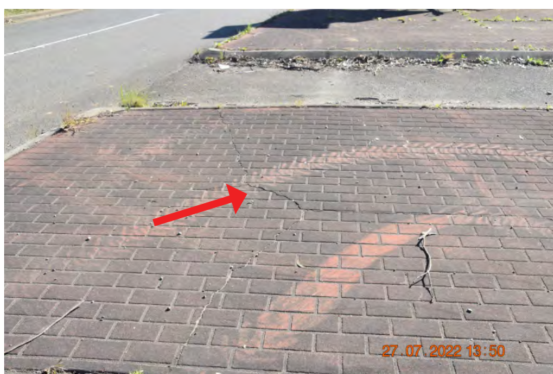
Figure: 0554 Slight cracking in the median strip. | CHANGE: None
