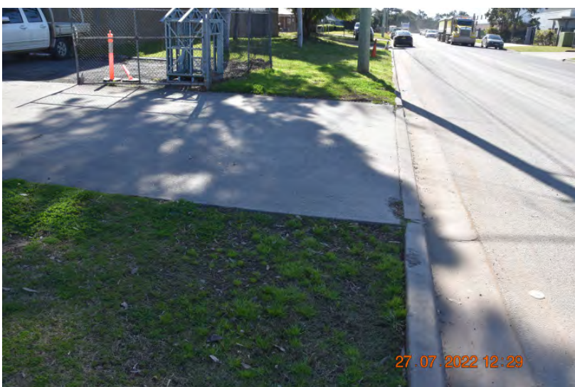
Figure: 0440 Chipping and slight cracking in the crossover. | CHANGE: None
