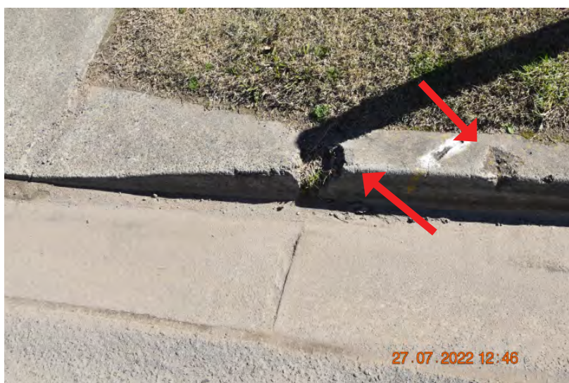
Figure: 0503 Chipping in the kerb. | CHANGE: None
