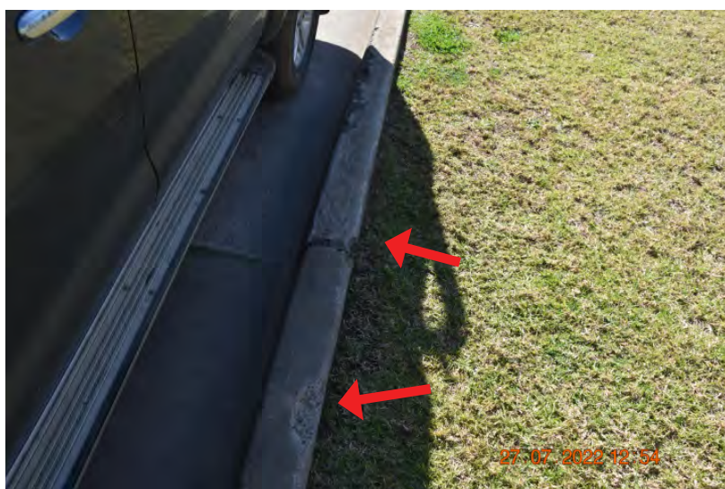
Figure: 0521 Chipping in the kerb. | CHANGE: None
