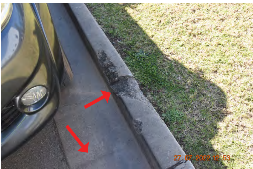
Figure: 0521 Chipping in the kerb. | CHANGE: None
