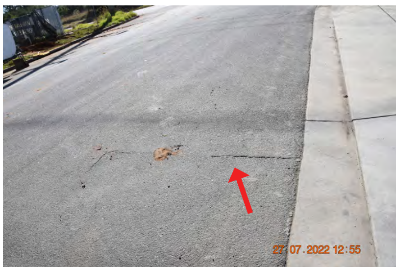
Figure: 0527 Slight cracking in the roadway. | CHANGE: None
