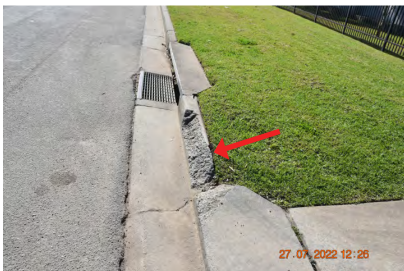
Figure: 0431 Chipping in the kerb and gutter. | CHANGE: None
