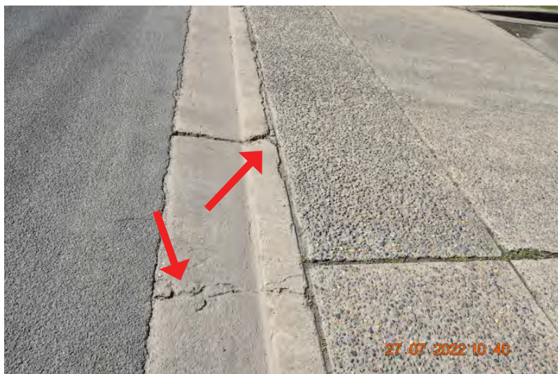
Figure: 0143 Fine cracking and chipping in the crossover. | CHANGE: None
