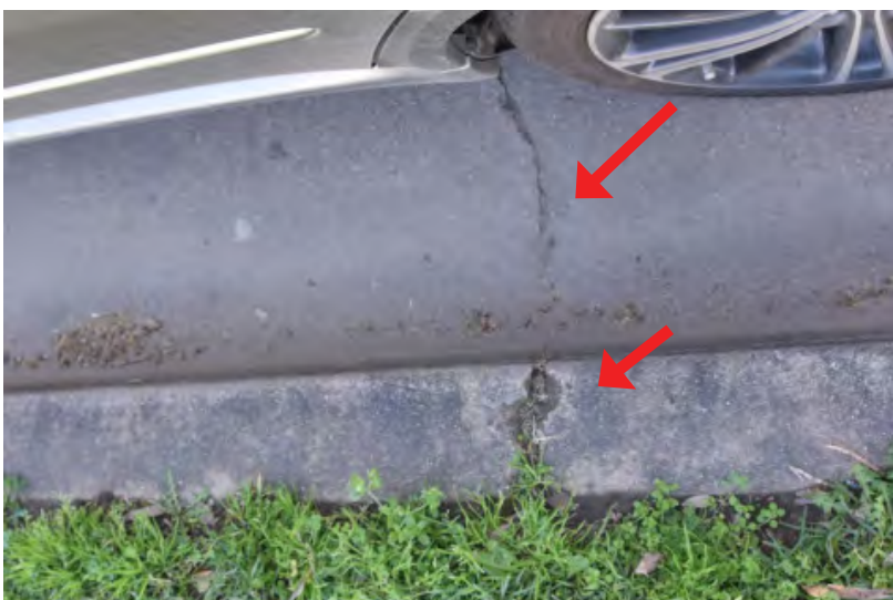
Figure: 0197 Slight cracking in the kerb and gutter. | CHANGE: None
