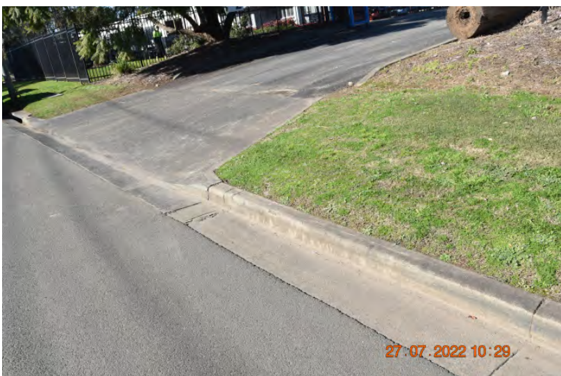
Figure: 0102 Slight cracking and chipping in the kerb and gutter. | CHANGE: None
