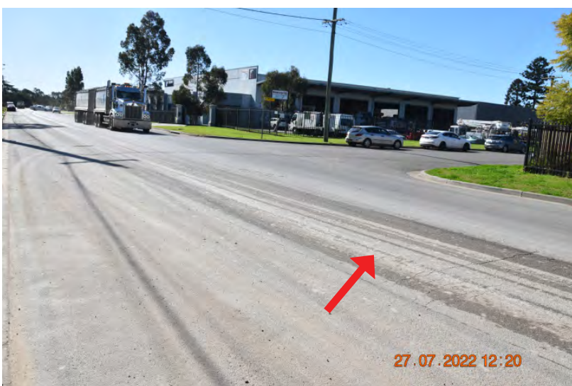
Figure: 0392 Alligator cracking in the paving. | CHANGE: None
