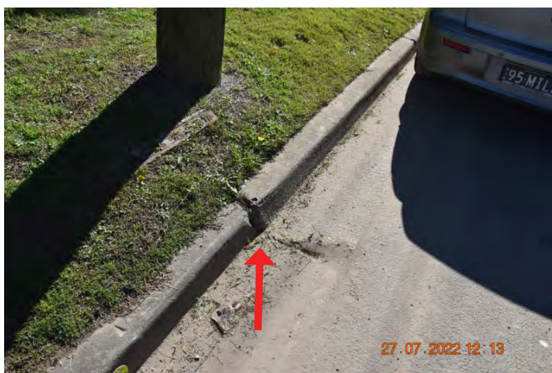
Figure: 0359 Slight cracking in the kerb and gutter. | CHANGE: None
