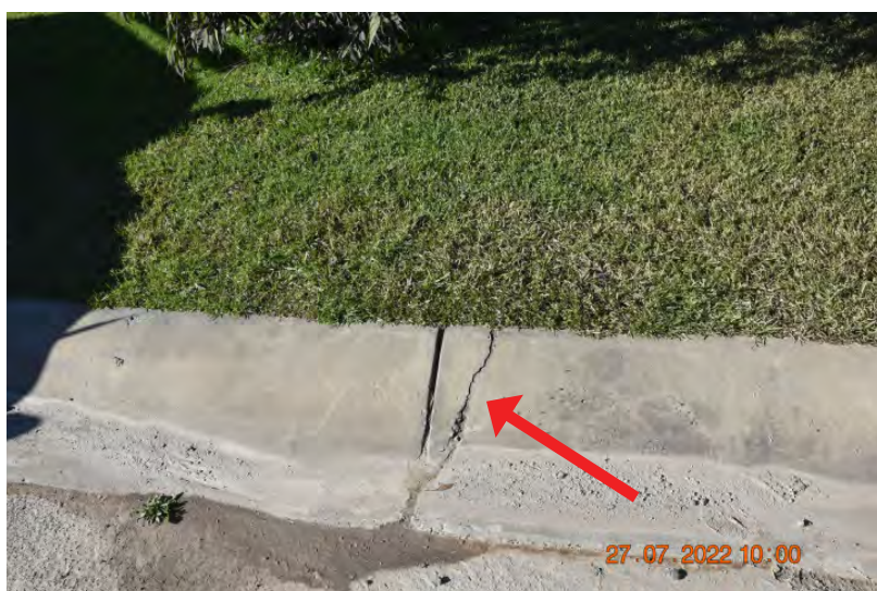
Figure: 0012 Slight cracking in the kerb and gutter. | CHANGE: None
