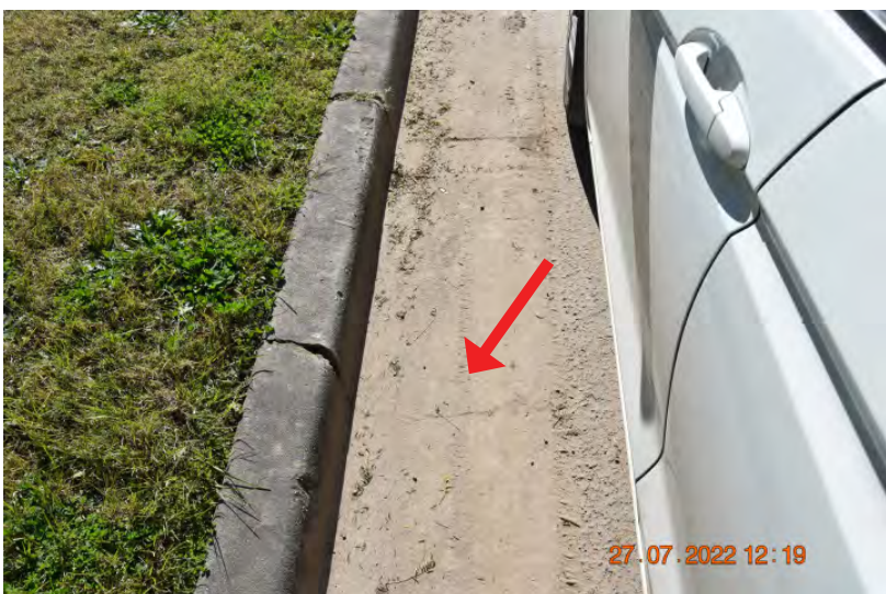
Figure: 0389 Fine cracking in the kerb and gutter. | CHANGE: None
