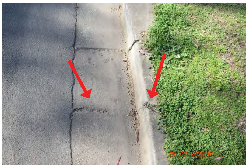
Figure: 0192 Slight cracking in the kerb and gutter. | CHANGE: None
