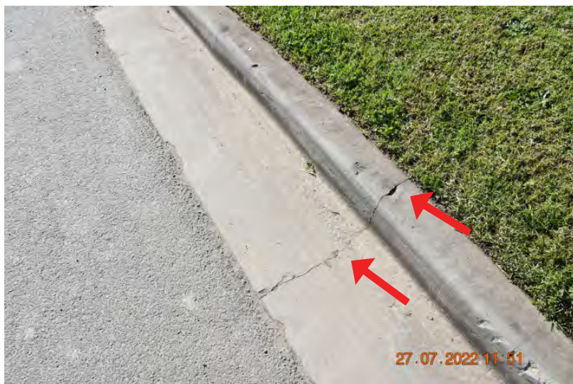
Figure: 0255 Fine cracking in the kerb and gutter, looking to the east. (RPT FOR FIGURES 256-257) | CHANGE: None
