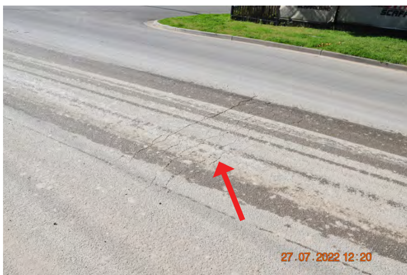
Figure: 0392 Alligator cracking in the paving. | CHANGE: None
