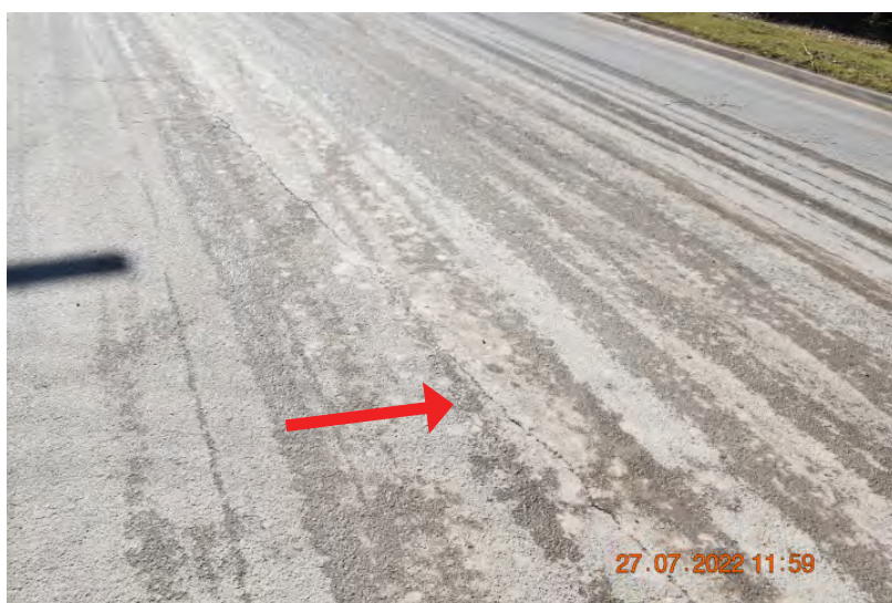
Figure: 0293 Slight cracking in the paving. (RPT FOR FIGURES 294-296) | CHANGE: None
