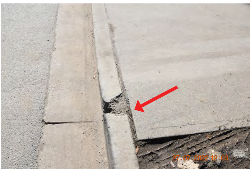
Figure: 0314 Chipping in the crossover. | CHANGE: None
