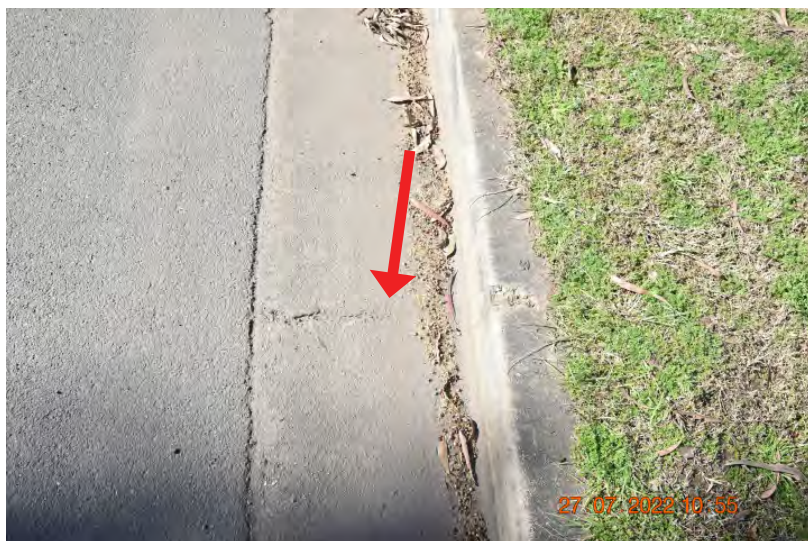
Figure: 0191 Chipping and fine cracking in the kerb and gutter. | CHANGE: None
