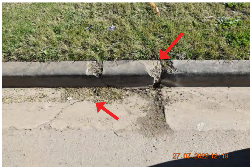
Figure: 0388 Fine cracking in the kerb. | CHANGE: None
