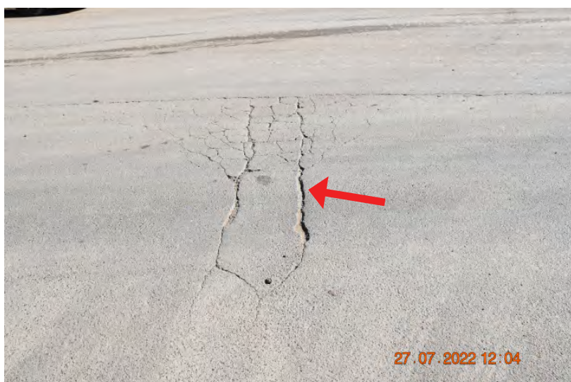
Figure: 0320 Slight cracking in the kerb and gutter. | CHANGE: Showing new condition.
