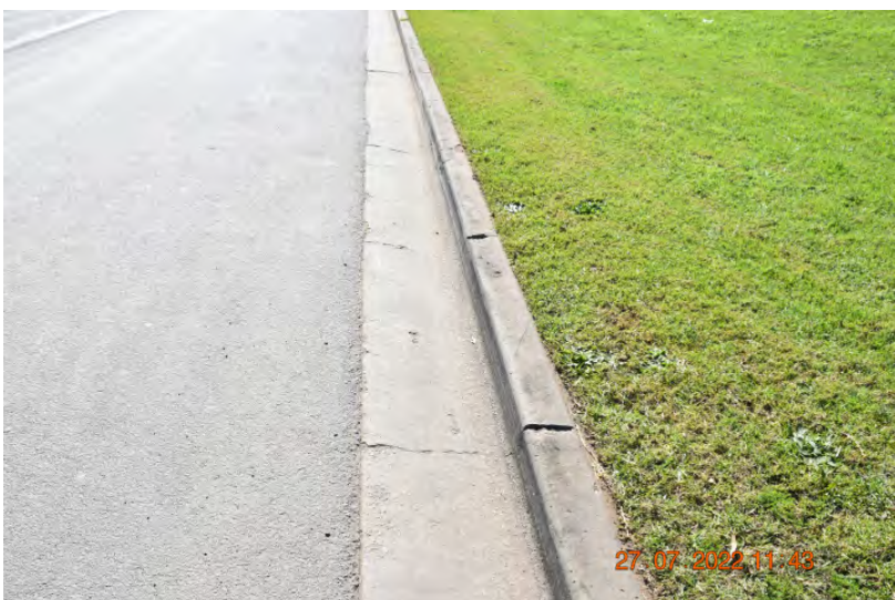
Figure: 0245 Chipping and cracking to the kerb and gutter. | CHANGE: None
