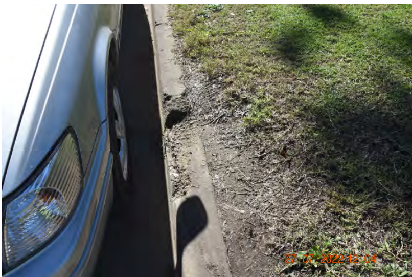
Figure: 0319 Slight cracking in the roadway, looking to the west. | CHANGE: None
