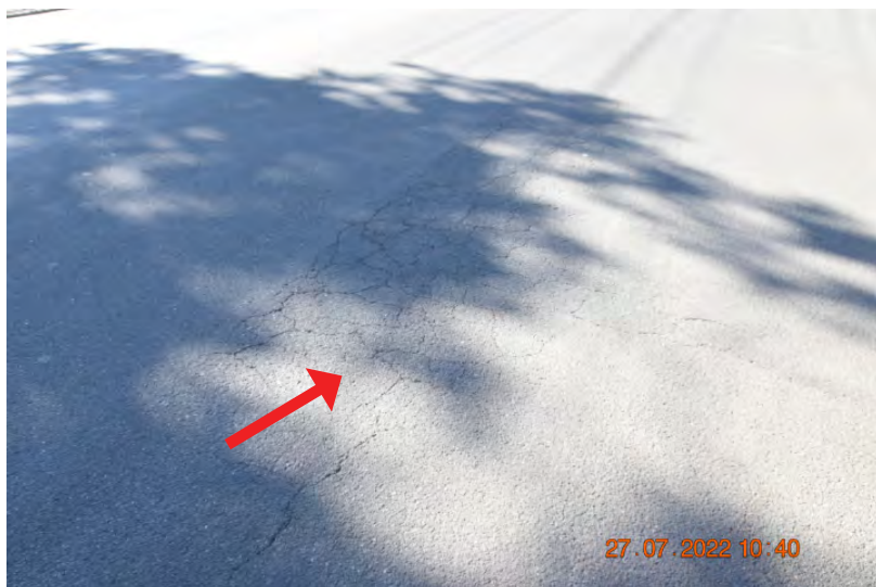
Figure: 0140 Cracking and scoring in the crossover. | CHANGE: None
