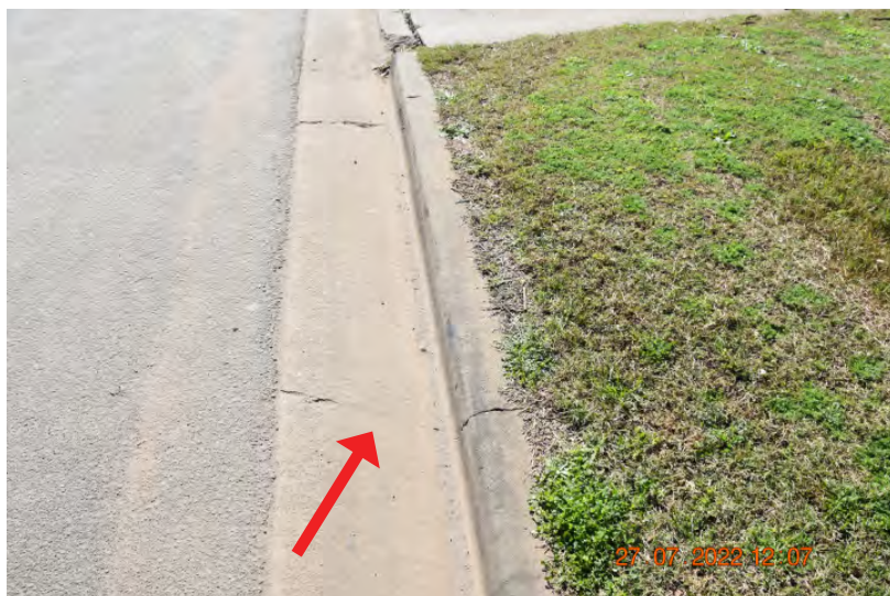
Figure: 0334 Slight cracking in the kerb and gutter. | CHANGE: None
