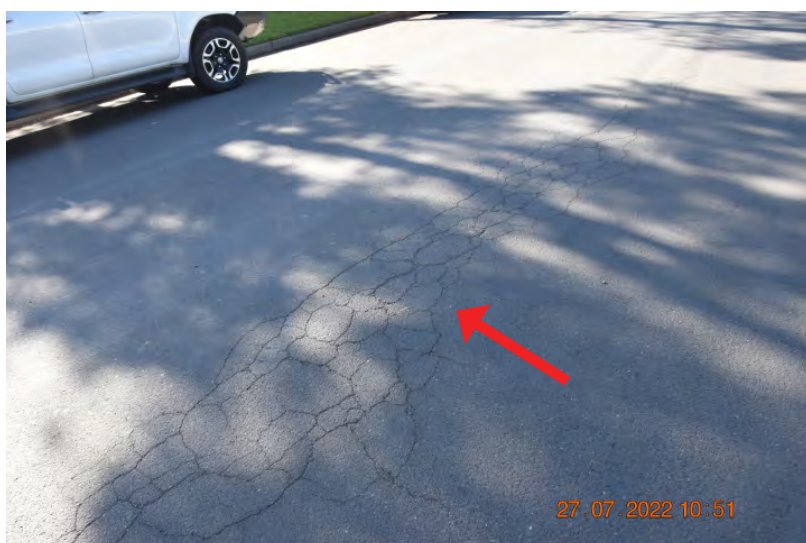
Figure: 0183 Fine cracking in the paving, looking to the north. (RPT FOR FIGURES 183-185) | CHANGE: None
