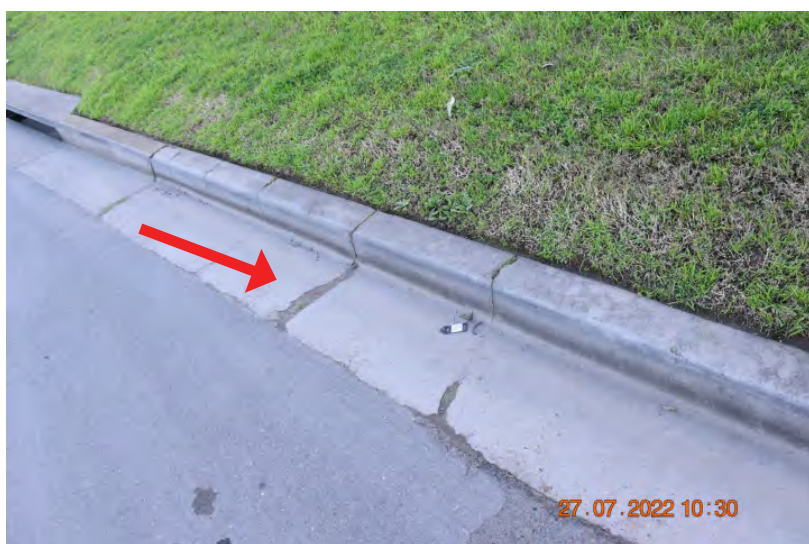
Figure: 0105 Slight cracking and chipping in the kerb and gutter. | CHANGE: None
