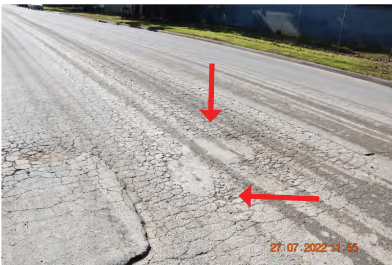
Figure: 0275 Slight alligator cracking in the paving. Also showing subsidence. | CHANGE: None
