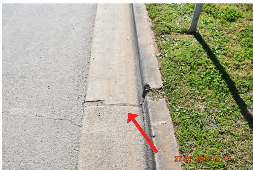
Figure: 0242 Slight cracking in the kerb and gutter. (RPT FOR FIGURES 243-245) | CHANGE: None
