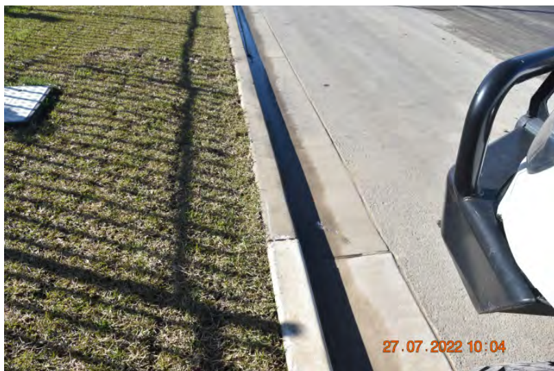
Figure: 0029 Chipping in the kerb. | CHANGE: None
