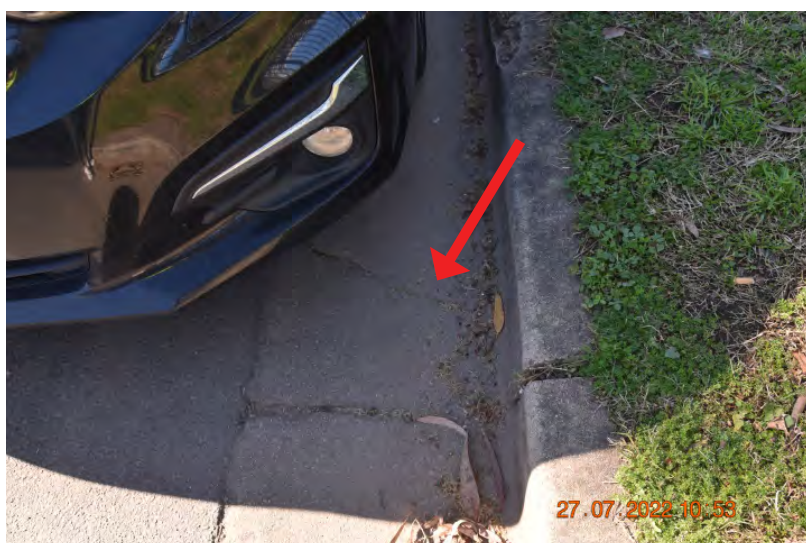
Figure: 0189 Chipping in the kerb. | CHANGE: None
