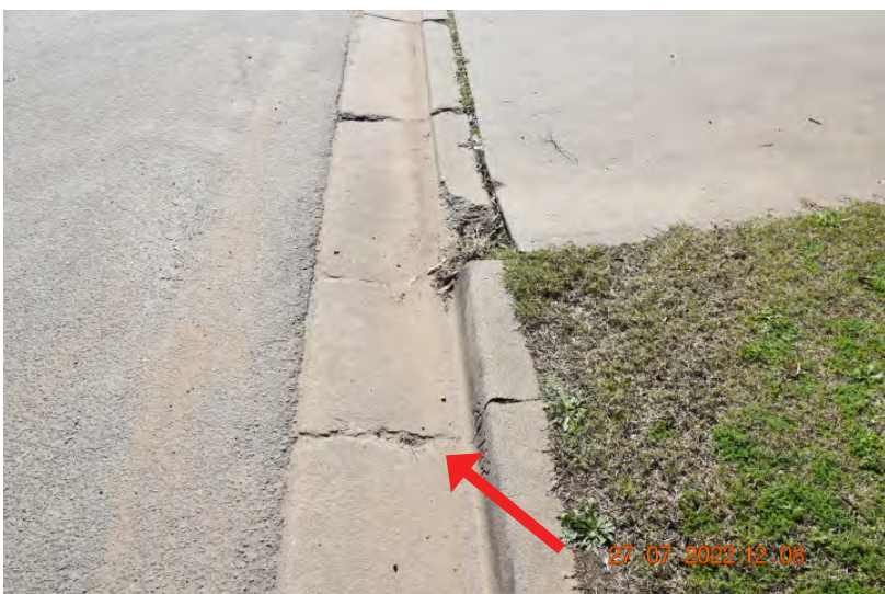
Figure: 0335 Chipping and slight cracking in the crossover. | CHANGE: None
