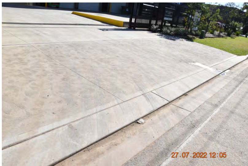
Figure: 0322 Slight alligator cracking in the paving. (RPT FOR FIGURES 323-324) | CHANGE: None
