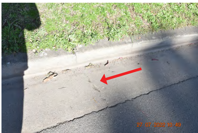
Figure: 0171 Slight cracking in the kerb and gutter, looking to the west. | CHANGE: None
