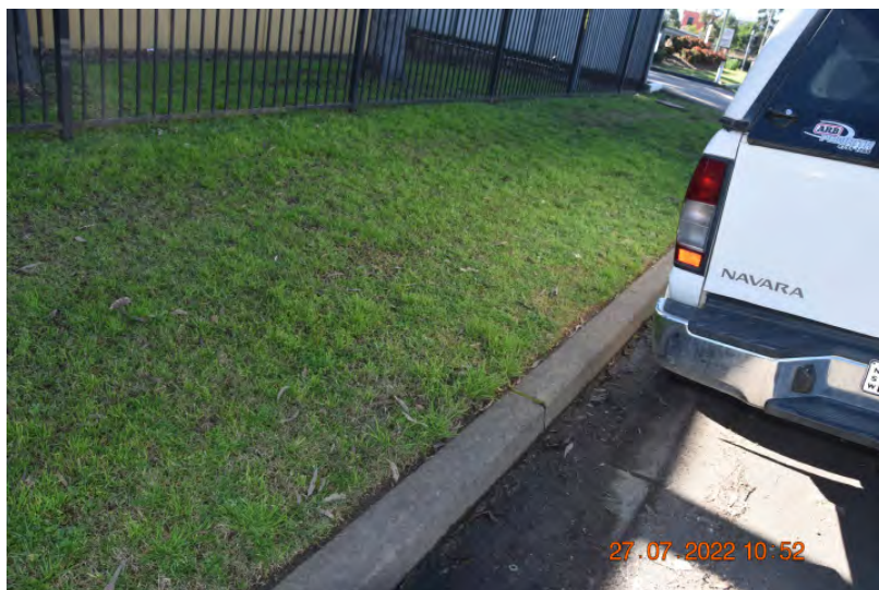
Figure: 0188 Chipping in the kerb. | CHANGE: None
