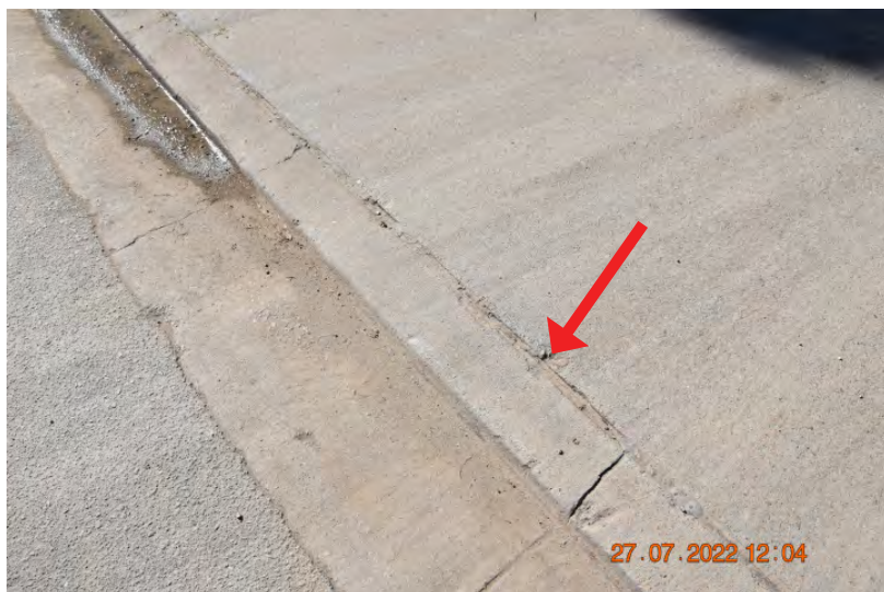
Figure: 0316 Chipping in the kerb. (RPT FOR FIGURES 317-319) | CHANGE: None
