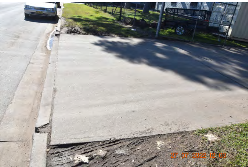
Figure: 0314 Chipping in the crossover. | CHANGE: None
