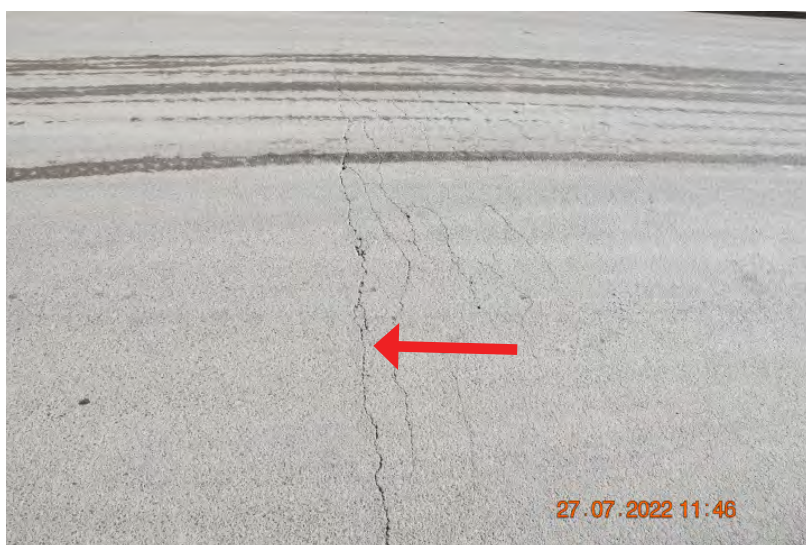
Figure: 0251 Fine cracking in the paving. | CHANGE: None
