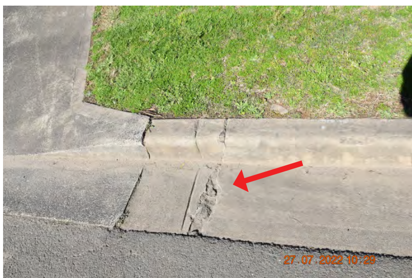
Figure: 0102 Slight cracking and chipping in the kerb and gutter. | CHANGE: None
