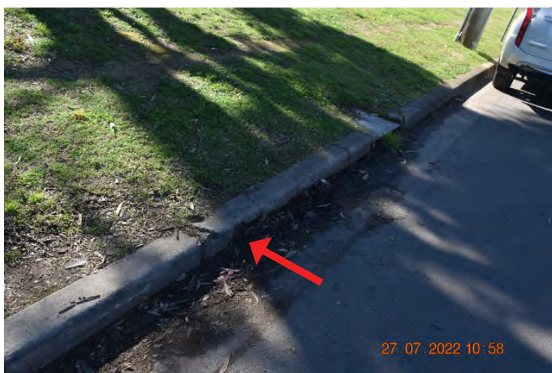
Figure: 0203 Chipping in the kerb, looking to the north. | CHANGE: None
