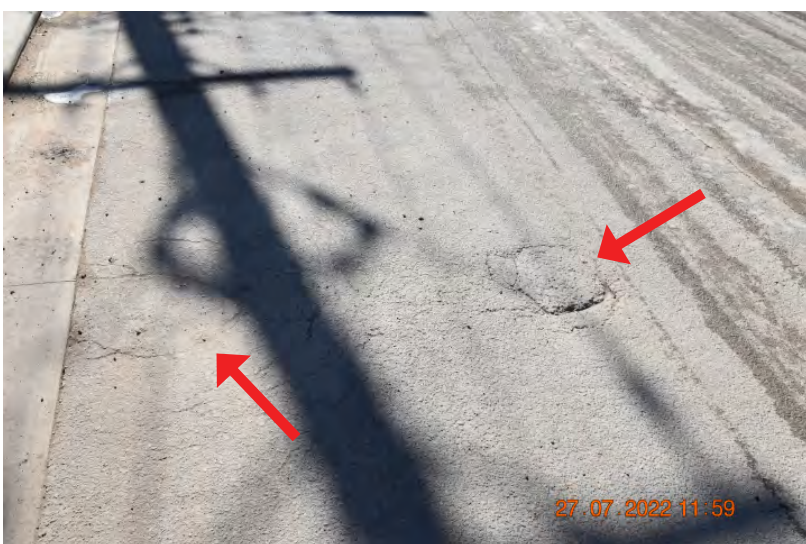
Figure: 0293 Slight cracking in the paving. (RPT FOR FIGURES 294-296) | CHANGE: None
