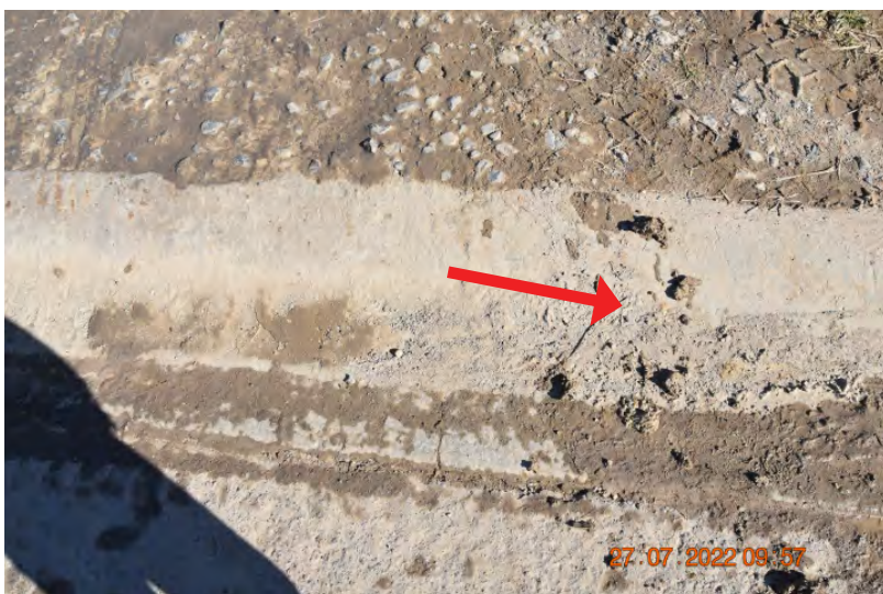
Figure: 0006 Fine cracking in the kerb and gutter, looking to the west. | CHANGE: None
