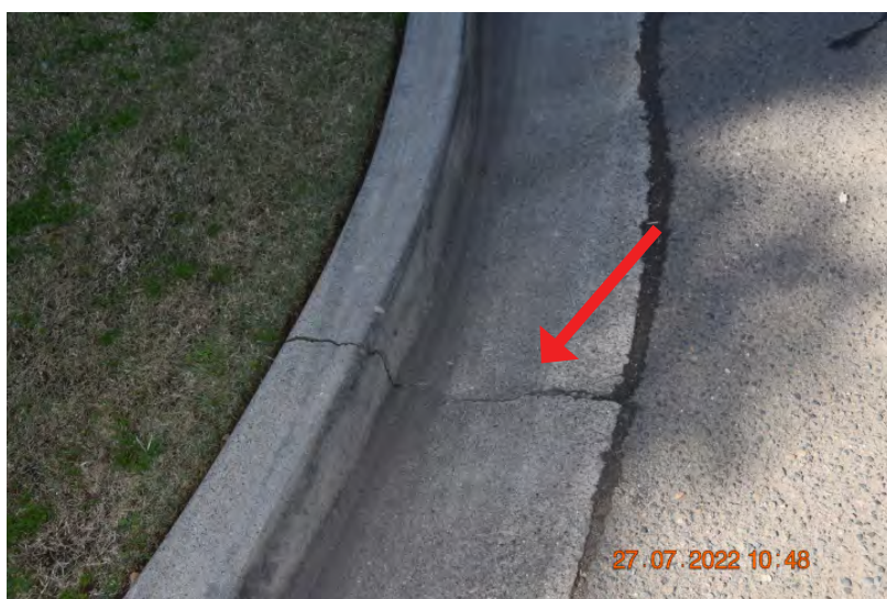
Figure: 0168 Fine cracking in the kerb and gutter. | CHANGE: Showing exacerbated cracking. | CHANGE: None
