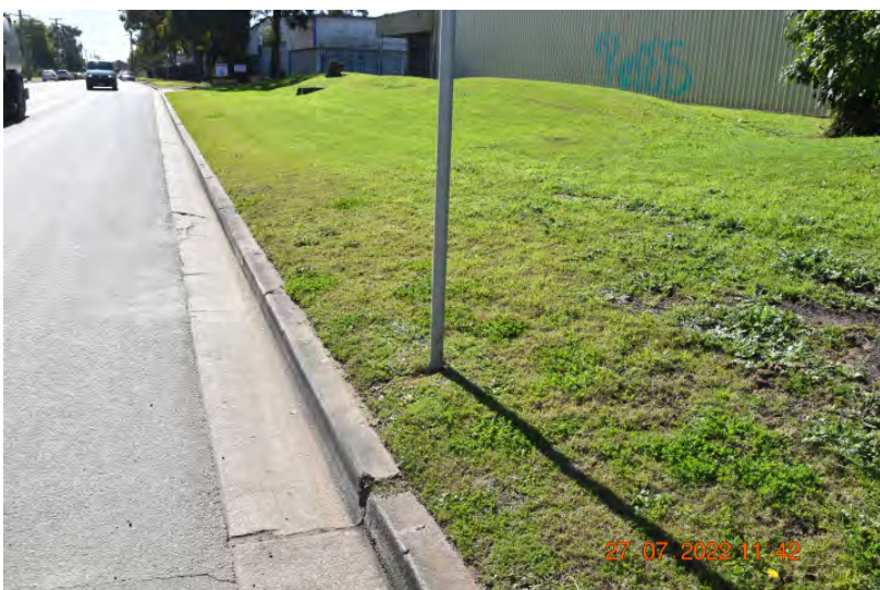
Figure: 0242 Slight cracking in the kerb and gutter. (RPT FOR FIGURES 243-245) | CHANGE: None
