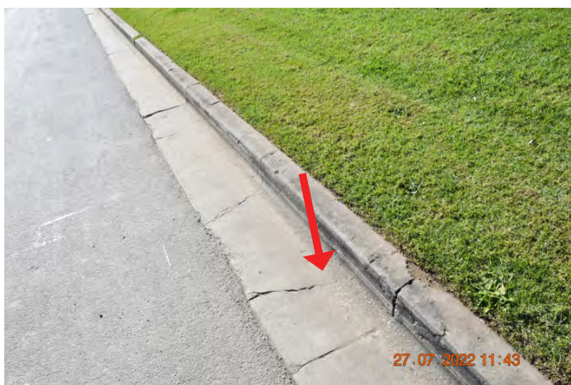
Figure: 0245 Chipping and cracking to the kerb and gutter. | CHANGE: None
