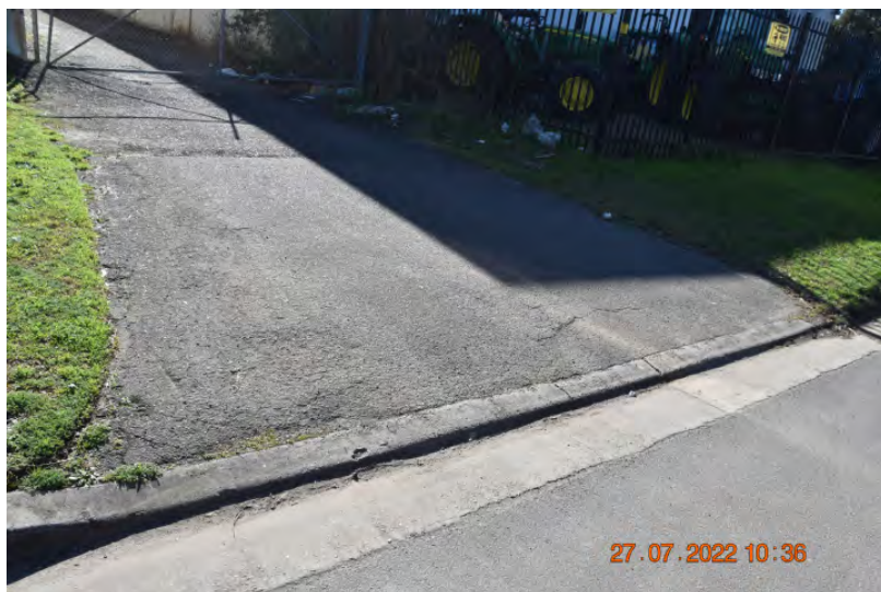
Figure: 0122 Fine cracking in the crossover, looking to the south. (RPT FOR FIGURES 122-123) | CHANGE: None
