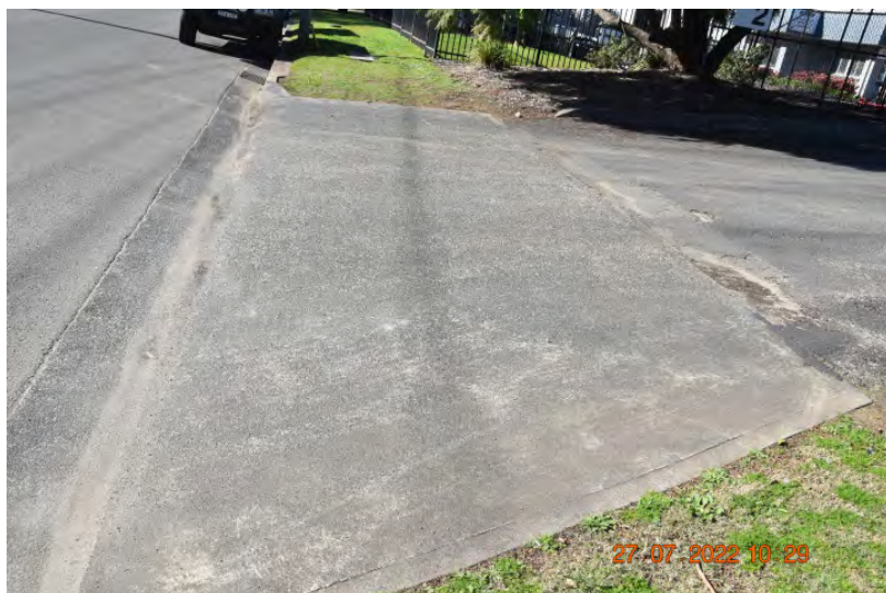
Figure: 0104 Cracking and chipping in the kerb and gutter, looking to the north. | CHANGE: None
