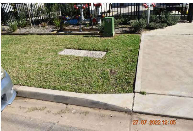
Figure: 0320 Slight cracking in the kerb and gutter. | CHANGE: Showing new condition.
