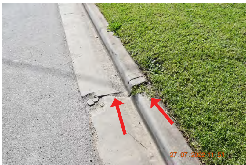
Figure: 0254 Chipping in the kerb and gutter. | CHANGE: None
