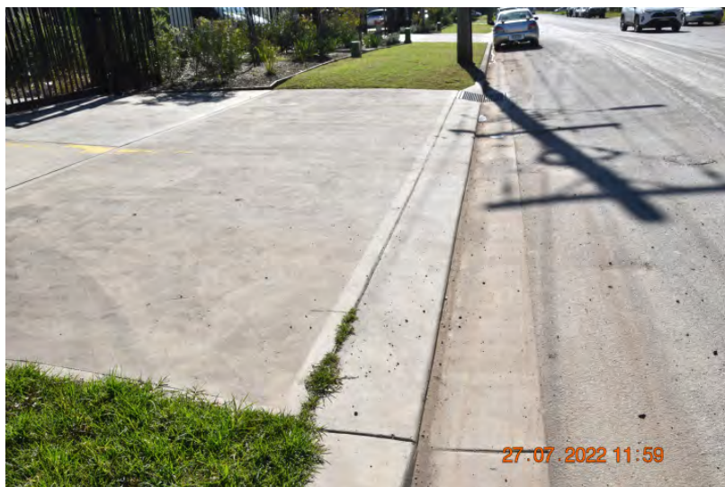
Figure: 0292 Subsidence in the paving. | CHANGE: None
