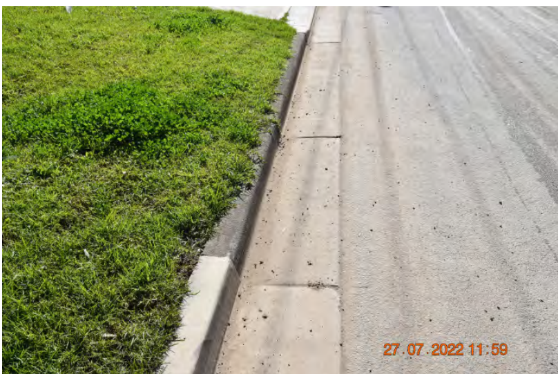
Figure: 0290 Fine cracking in the kerb and gutter. | CHANGE: None
