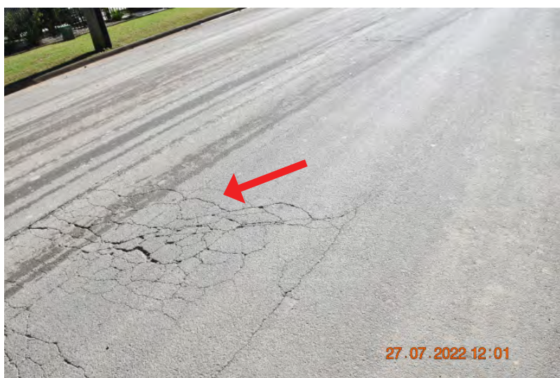
Figure: 0299 Slight cracking in the paving. (RPT FOR FIGURES 300-301) | CHANGE: None
