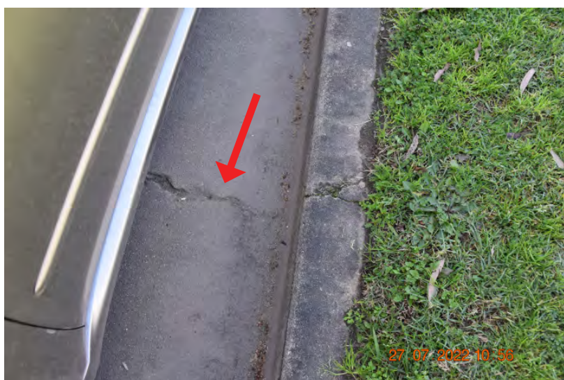
Figure: 0195 Fine cracking in the kerb and gutter. (RPT FOR FIGURES 195-197) | CHANGE: None
