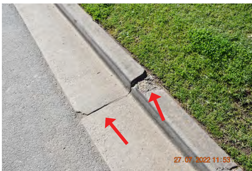
Figure: 0266 Fine cracking and chipping in the kerb and gutter, looking to the east. (RPT FOR FIGURES 267-269) | CHANGE: None
