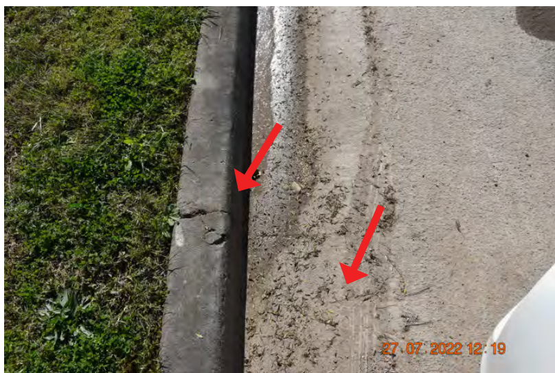
Figure: 0389 Fine cracking in the kerb and gutter. | CHANGE: None
