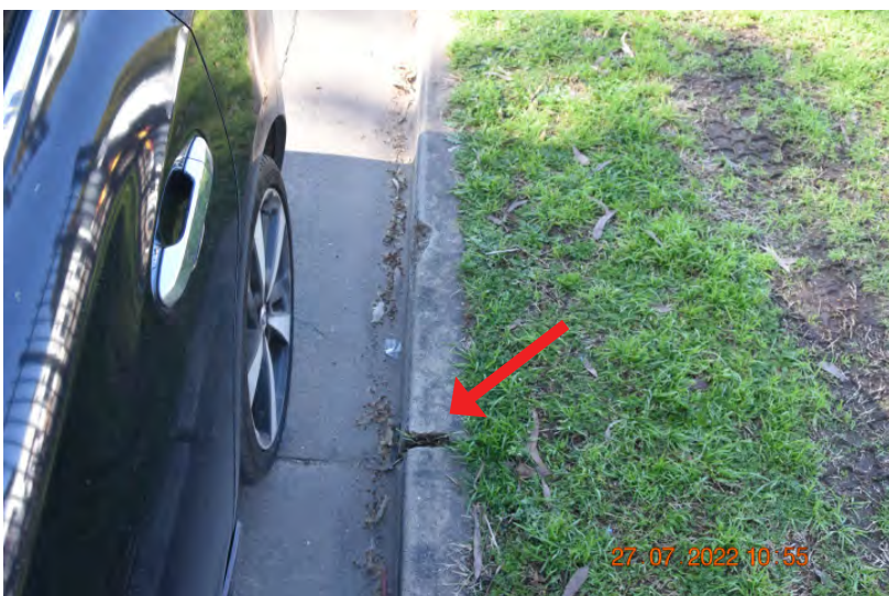
Figure: 0192 Slight cracking in the kerb and gutter. | CHANGE: None
