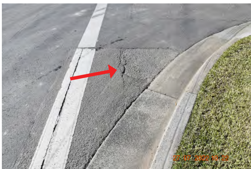
Figure: 0072 Slight cracking in the paving. | CHANGE: None
