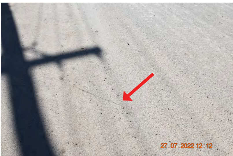
Figure: 0353 Fine cracking in the paving. (RPT FOR FIGURES 354-356) | CHANGE: None
