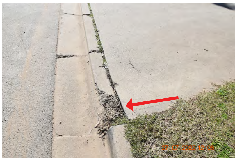
Figure: 0335 Chipping and slight cracking in the crossover. | CHANGE: None
