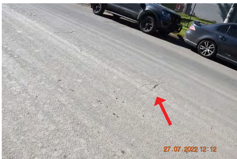
Figure: 0353 Fine cracking in the paving. (RPT FOR FIGURES 354-356) | CHANGE: None
