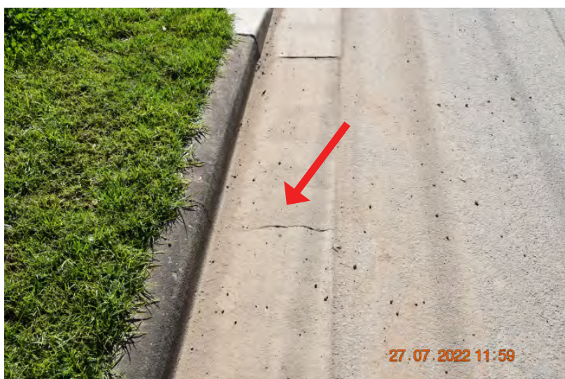
Figure: 0290 Fine cracking in the kerb and gutter. | CHANGE: None
