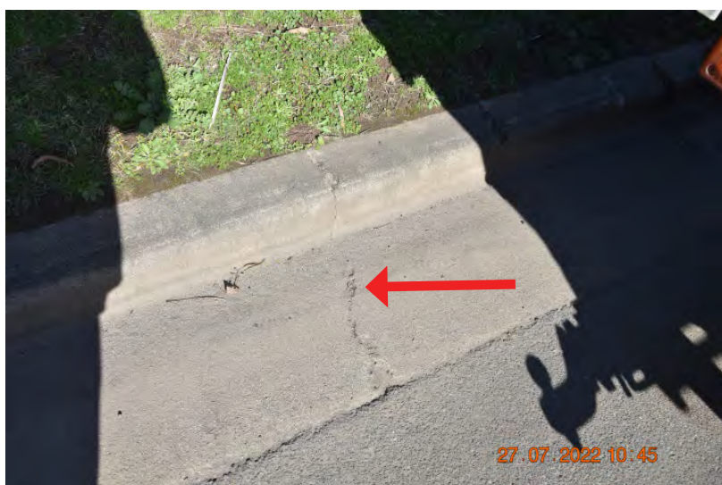
Figure: 0156 Substantial cracking in the kerb and gutter. | CHANGE: None
