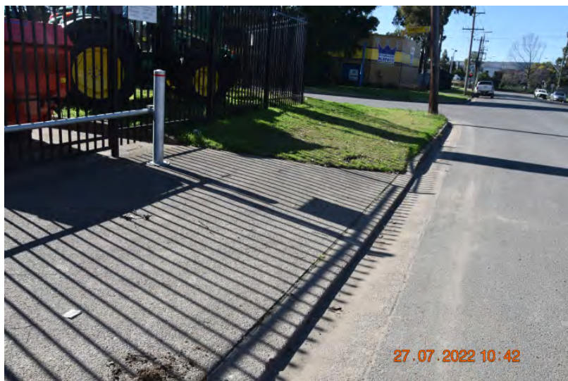
Figure: 0146 Slight cracking in the crossover. (RPT FOR FIGURES 146-148) | CHANGE: None
