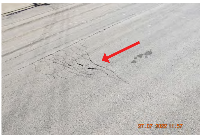
Figure: 0284 Slight cracking in the paving. (RPT FOR FIGURES 285-288) | CHANGE: None
