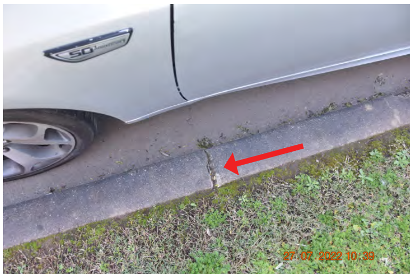
Figure: 0137 Slight cracking and chipping in the kerb and gutter, looking to the south. | CHANGE: None
