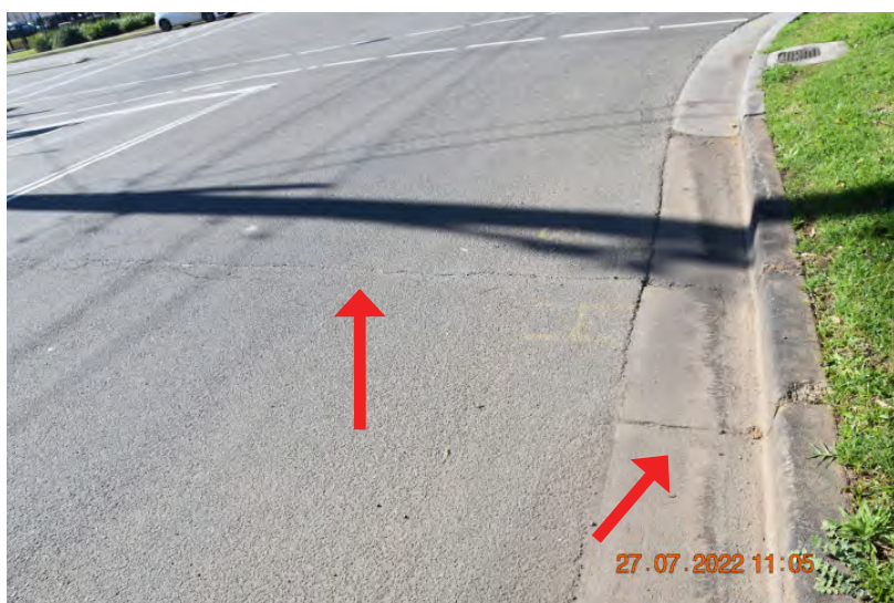
Figure: 0227 Slight cracking to the paving and the kerb and gutter. | CHANGE: None
