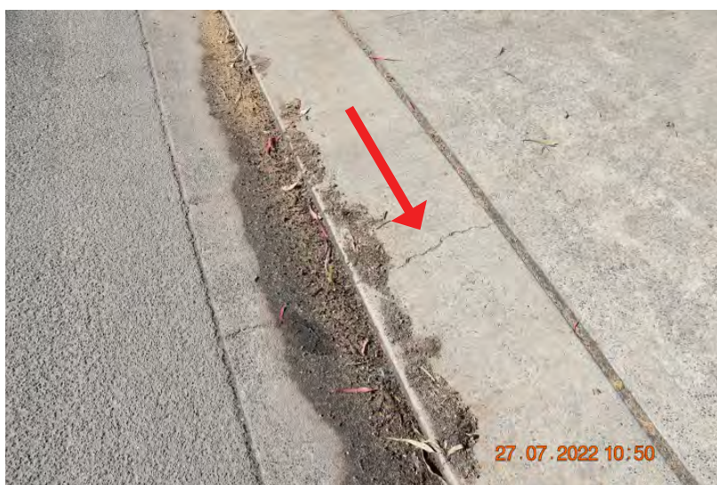
Figure: 0177 Slight cracking in the crossover. (RPT FOR FIGURES 177-178) | CHANGE: None
