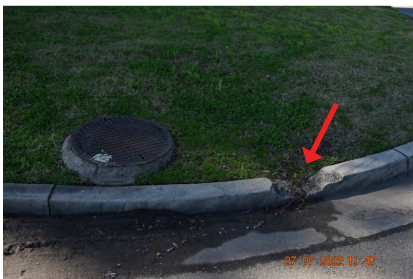
Figure: 0165 Chipping in the kerb and gutter. | CHANGE: None
