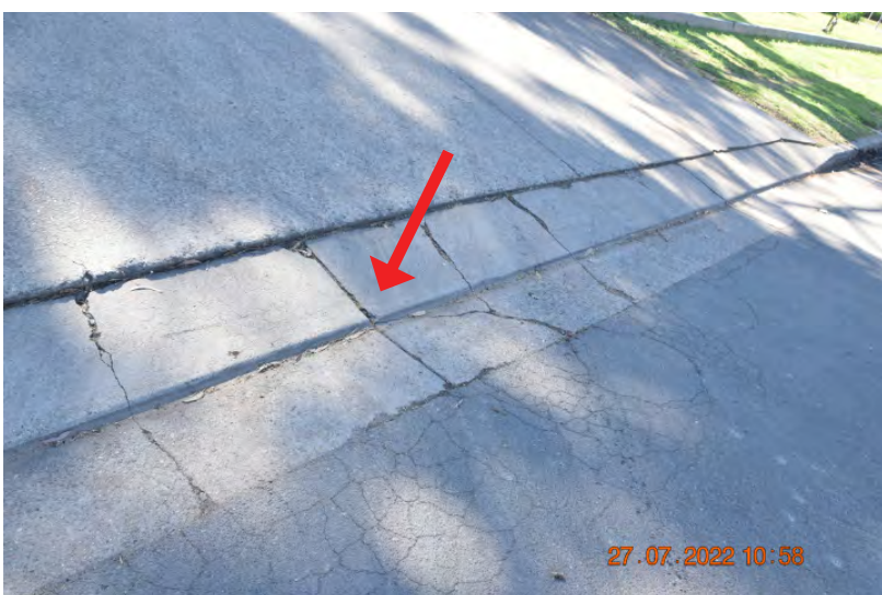
Figure: 0203 Chipping in the kerb, looking to the north. | CHANGE: None
