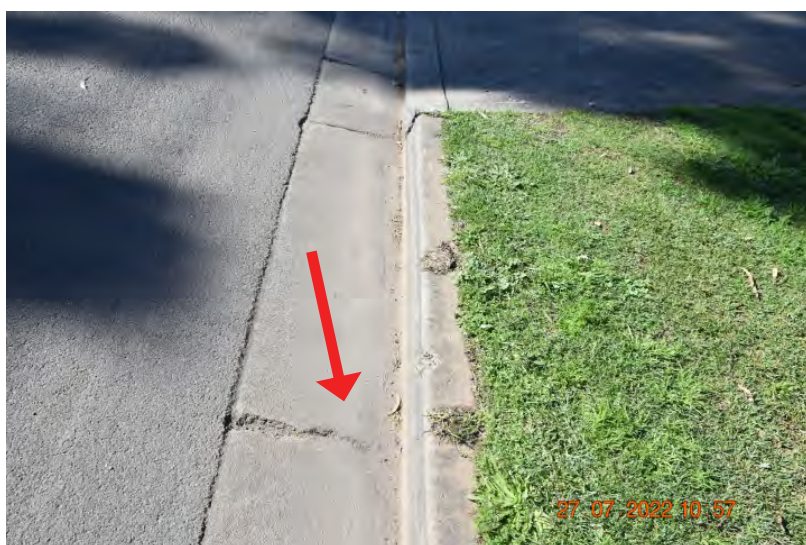
Figure: 0197 Slight cracking in the kerb and gutter. | CHANGE: None
