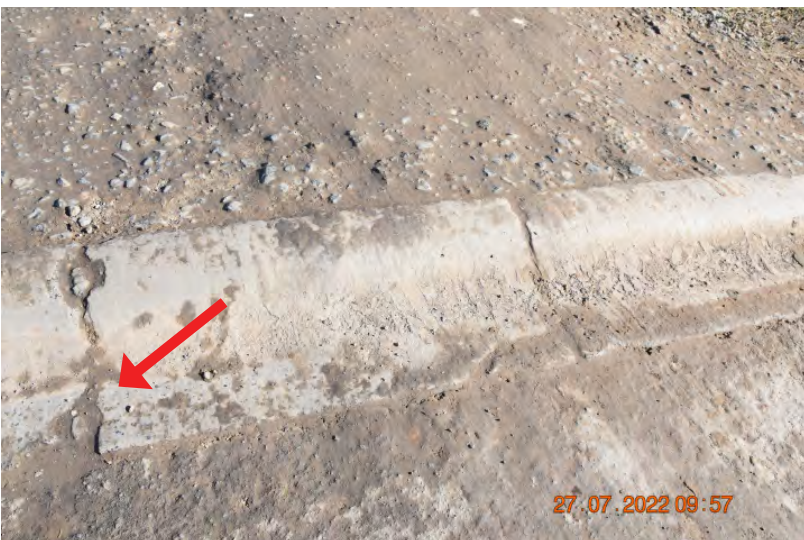
Figure: 0006 Fine cracking in the kerb and gutter, looking to the west. | CHANGE: None
