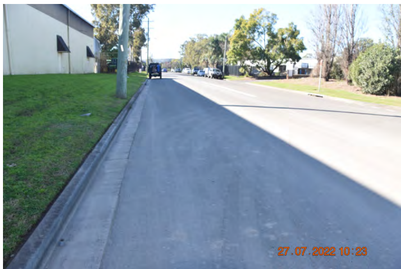
Figure: 0080 Slight alligator cracking in the paving. (RPT FOR FIGURES 80-85) | CHANGE: None
