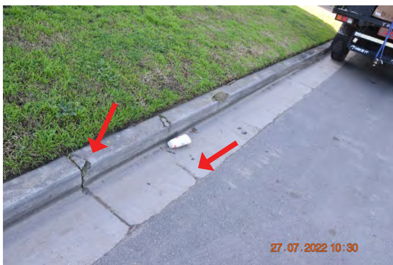
Figure: 0105 Slight cracking and chipping in the kerb and gutter. | CHANGE: None
