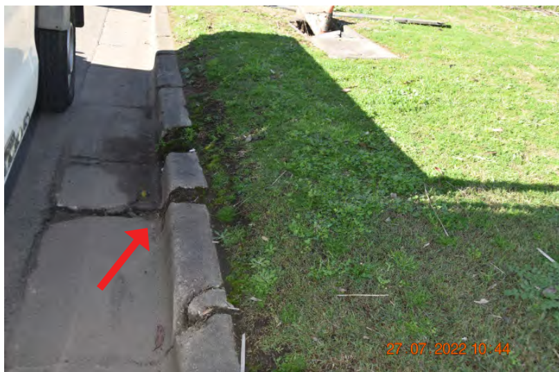
Figure: 0155 Missing pit lid. | CHANGE: None
