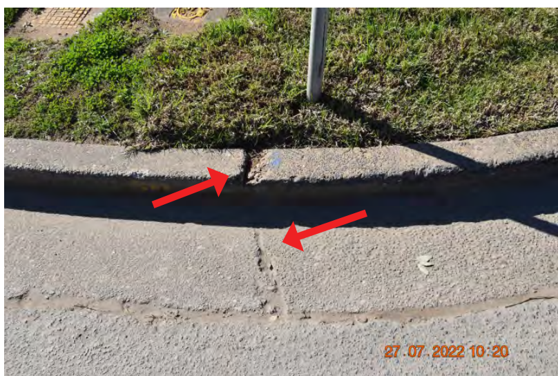
Figure: 0063 Slight cracking and chipping in the kerb and gutter. | CHANGE: None
