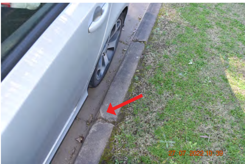
Figure: 0138 Slight cracking in the kerb and gutter, looking to the south. | CHANGE: None
