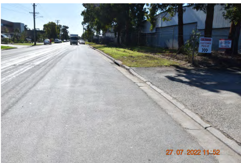
Figure: 0266 Fine cracking and chipping in the kerb and gutter, looking to the east. (RPT FOR FIGURES 267-269) | CHANGE: None
