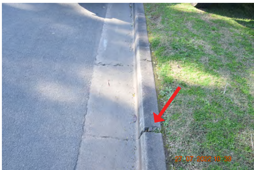
Figure: 0138 Slight cracking in the kerb and gutter, looking to the south. | CHANGE: None
