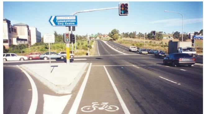
**Figure 7.1: Provision for bicycle operating space at intersections: the Six Intersection Elements.**
