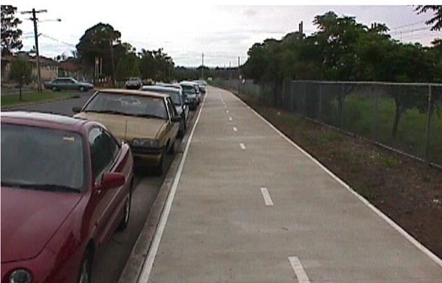
**Photo 8.1 (Left top):** Example of a reinforced concrete path with an asphalt wearing course. Running track adjacent to compressed granite with concrete edging. The Bay Run Cycleway, King Georges Park, Rozelle.
