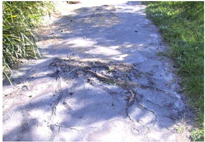
**Photo 8.8** Example tree root damage to an off-road path. Near Malabar Rd, Malabar.
