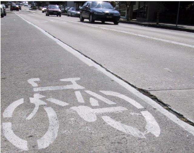
**Photo 8.4: Example of concrete road jointing and bicycle shoulder lanes. Edgecliff Rd, Bondi Junction.**
