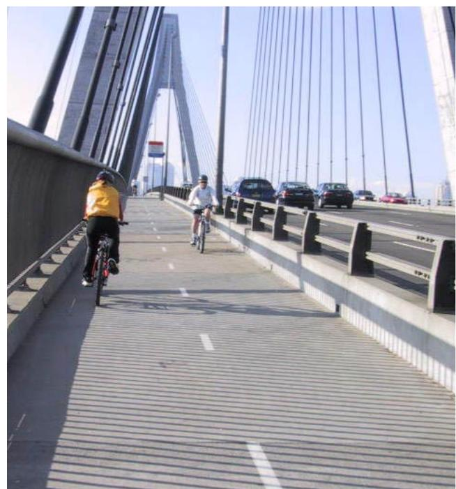
**Figure 8.3: Linemarking and pavement symbols.**
