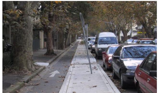
**Photo 5.9 (above): Protected bicycle contraflow lane located to the kerbside of parallel car parking. Bourke St, Surry Hills.**
