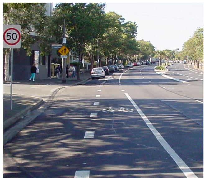
**Figure 5.3: Bicycle shoulder lanes across side streets with alternative marking for parking bays**
