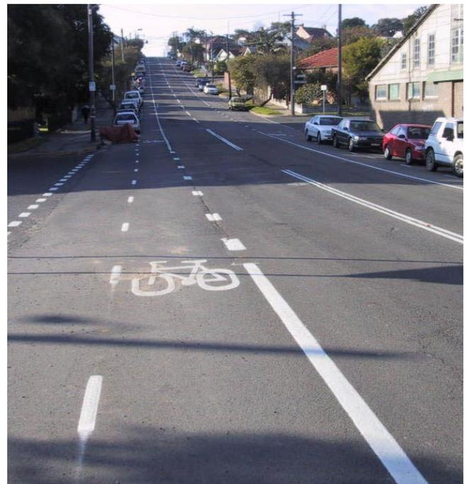
**Photo 7.3: Example of bicycle lanes through an unsignalled intersection. Lilyfield Rd, Lilyfield.**
