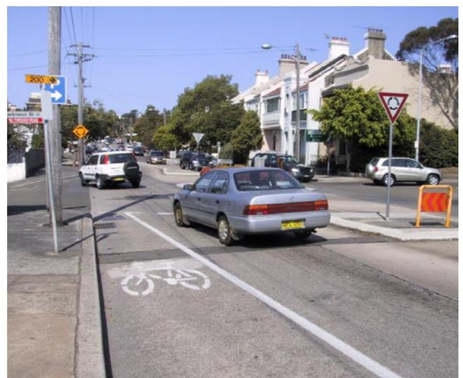
**Figure 7.9: Two bicycle routes crossing at a single-lane roundabout with visually separated bicycle operating space.**
