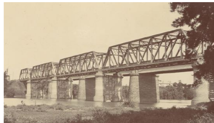
Figure 11: View of the Victoria Bridge over the Nepean River at Penrith, ca. 1900-1929 Source: State Library of NSW, File no: FL1060530
