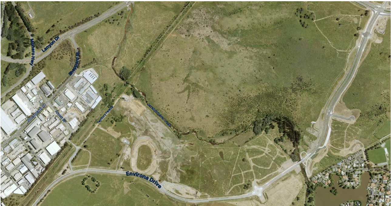
Figure 4-5 | Recently constructed Envirova Dve (Metromaps, 2022)
