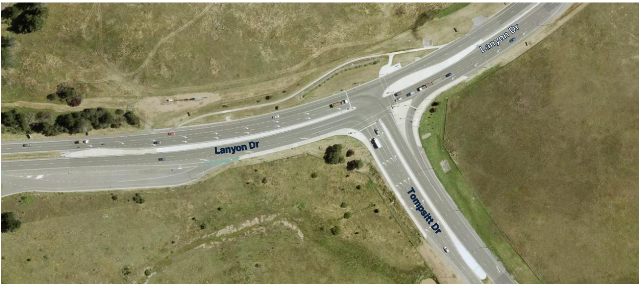
Figure 4-3 | Lanyon Dve intersection with Tomsitt Dve (source: Metromaps, 2022)
