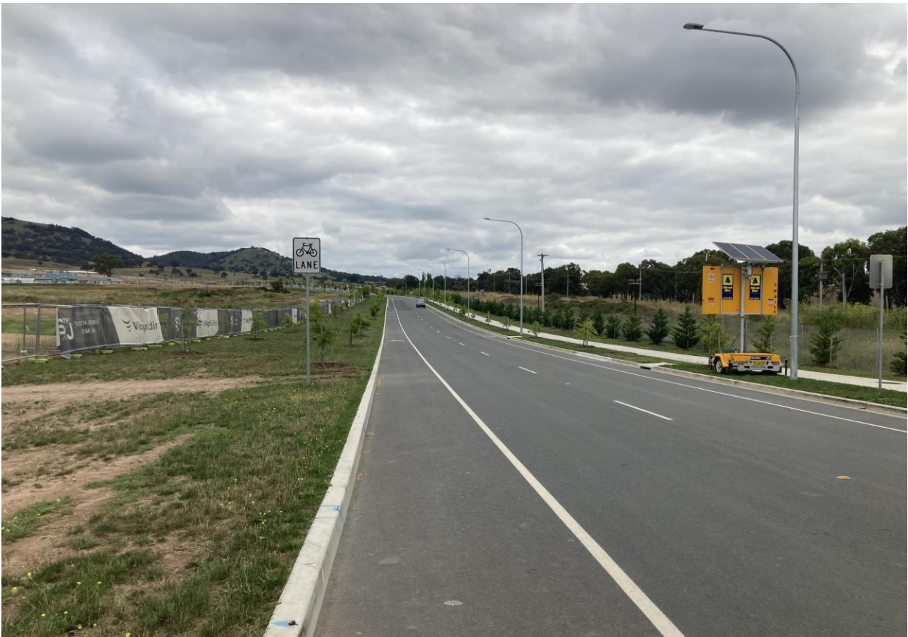
Figure 4-15 | Shared User Path adjacent to future local centre in Tralee and on-road cycle lanes in both directions along the southern portion of Envirova Drive
