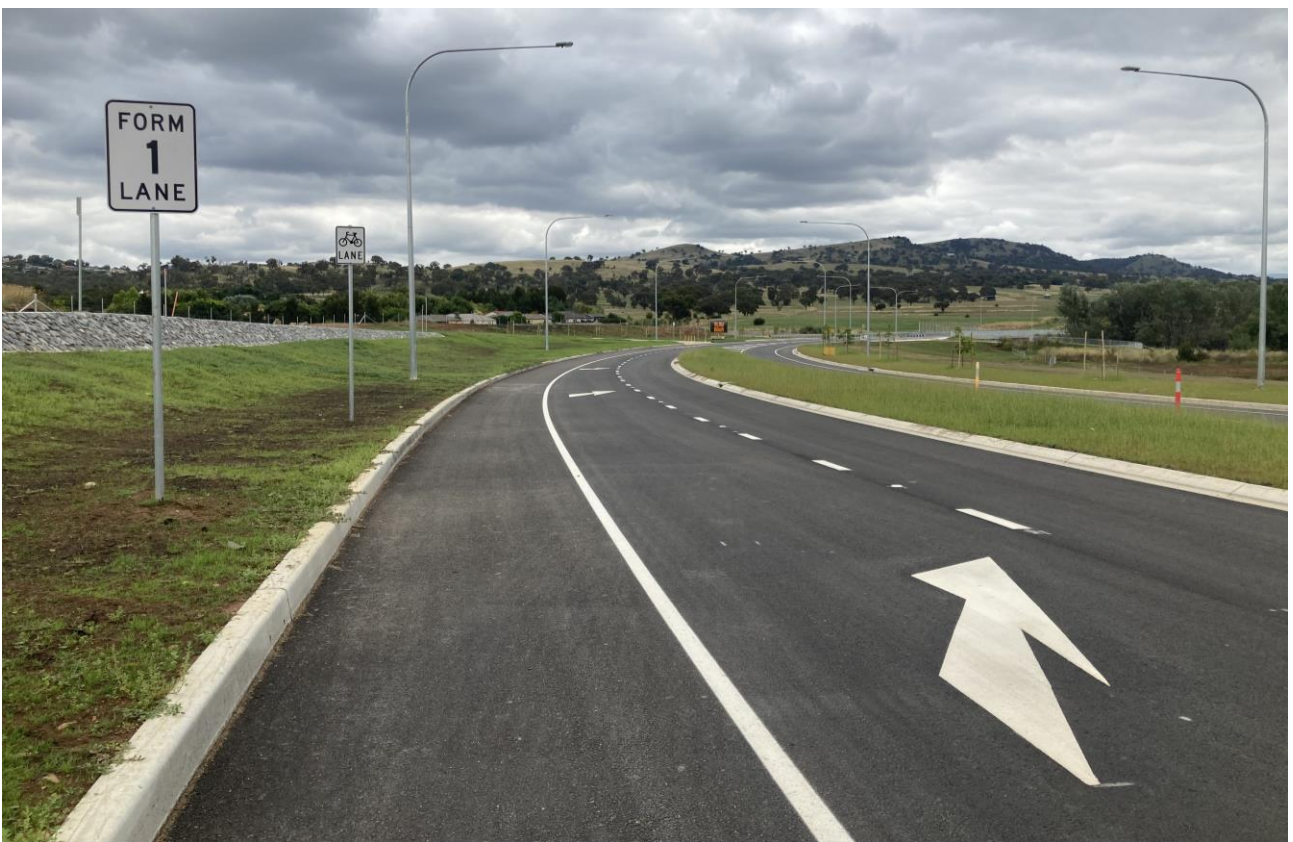
Figure 4-14 | On road cycle path on the southern section of Envirova Drive, to the south of the future high school
