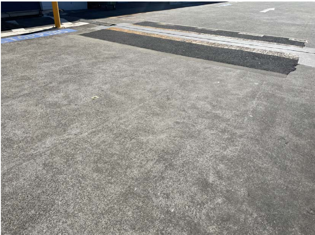
Photograph 6 Bitumen and concrete flooring in the car parking area.
