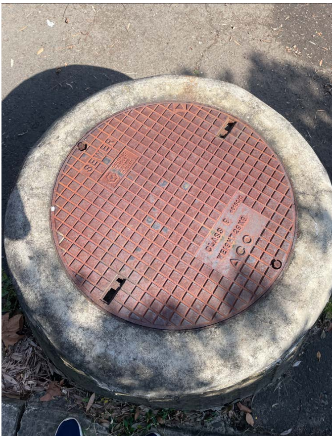
Photograph 16 Sewer pit noted on the eastern boundary.
