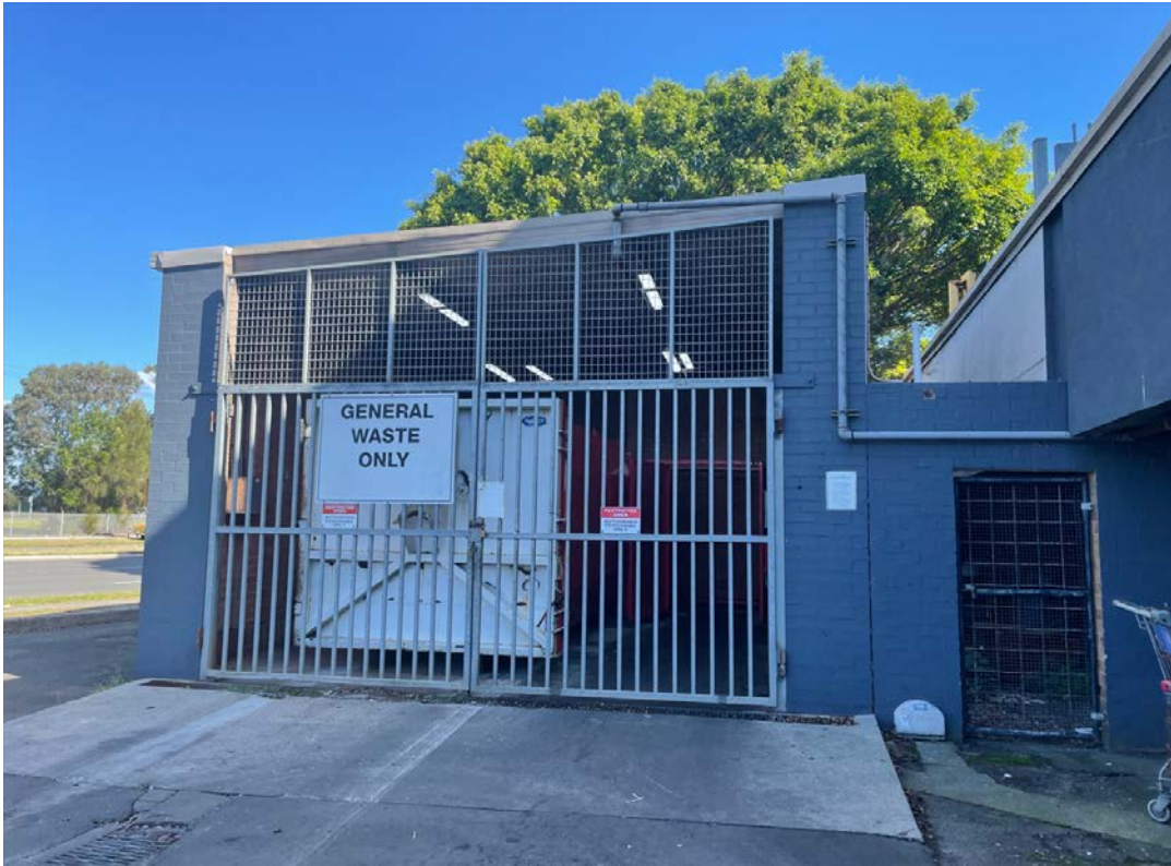
Photograph 7 Waste storage area at the site's southern boundary.
