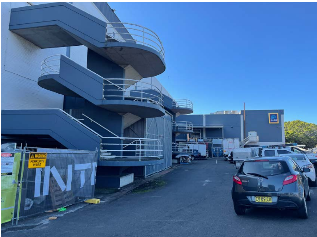
Photograph 10 Loading dock at the site's western boundary.
