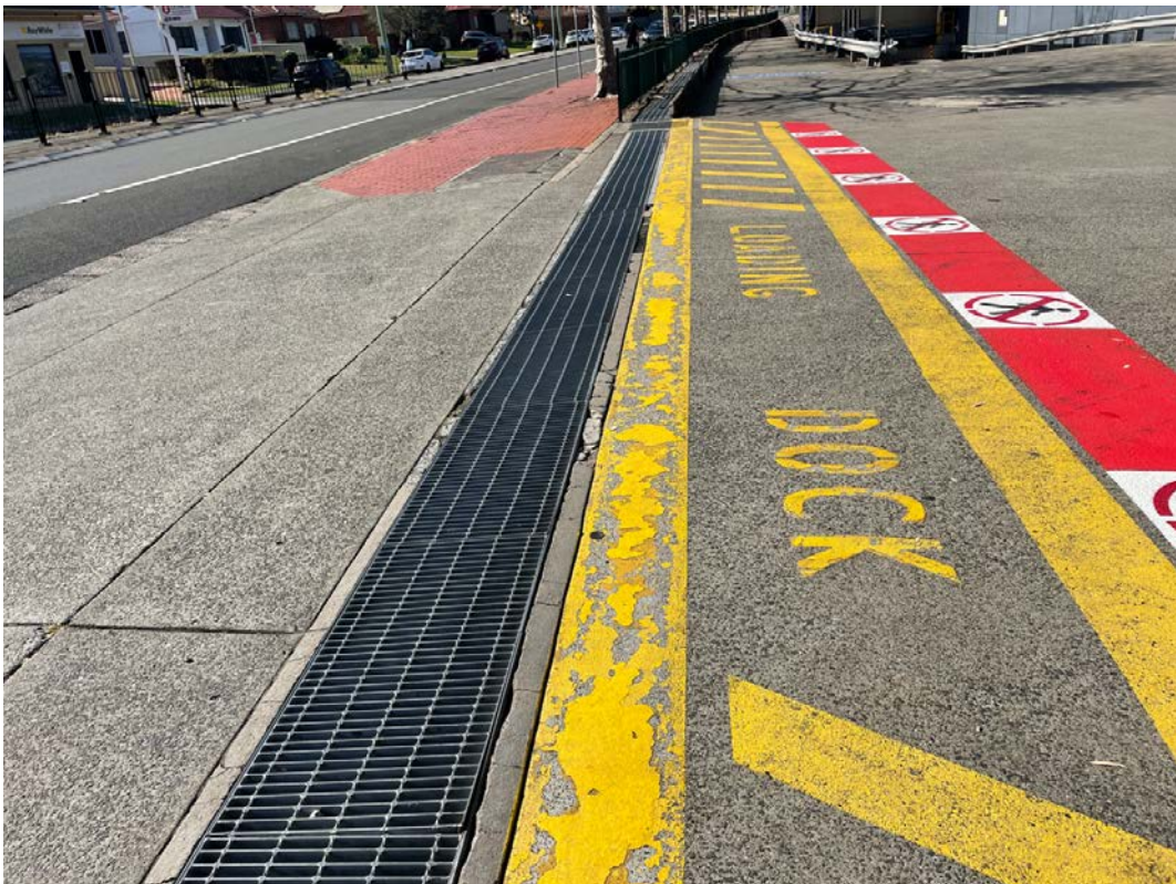
Photograph 18 Strip drains noted on the northern boundary.
