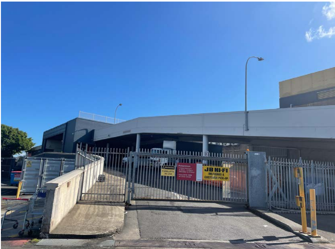
Photograph 8 Loading dock at the site's southern boundary.
