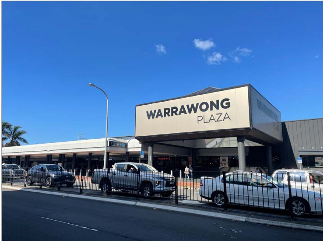
Photograph 1 Warrawong Plaza, looking south from Cowper Street.
