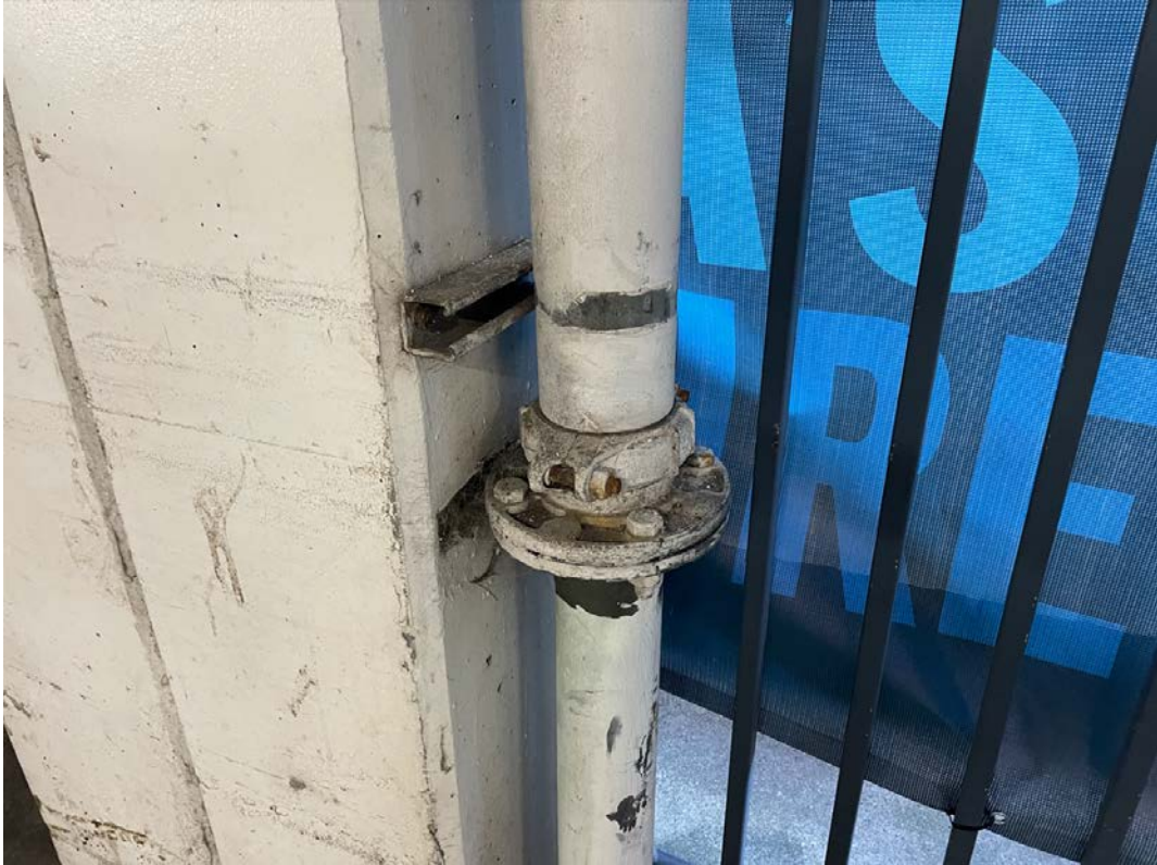
Photograph 5 Cement down pipes noted in the ground-floor car parking area.
