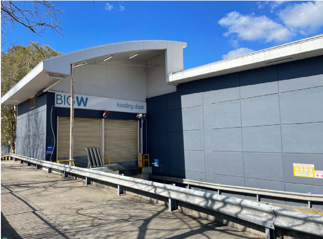
Photograph 9 Loading dock at the site's northern boundary.
