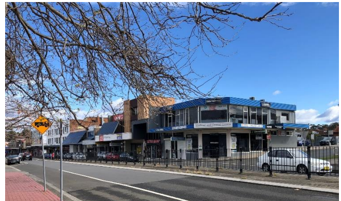
Figure 17 Commercial development on the northern side of Cowper Street looking from the north-eastern corner of the Site
