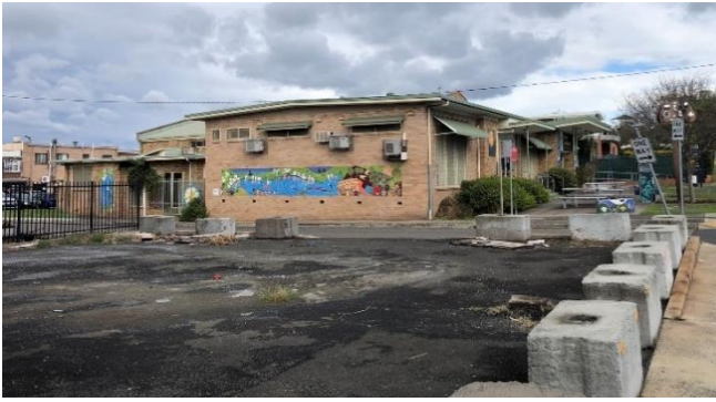
Figure 22 Future Warrawong Library Site and existing Warrawong Community Centre
