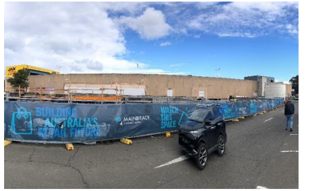
Figure 11 Warrawong Plaza looking from eastern boundary of the Site
