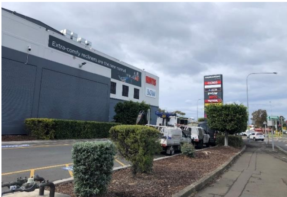
Figure 12 Warrawong Plaza at corner of King Street and Northcliffe Drive
