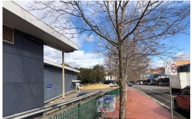
Figure 9 Warrawong Plaza looking west from Cowper Street
