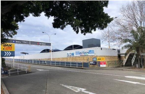
Figure 8 North-eastern corner of Warrawong Plaza Site
