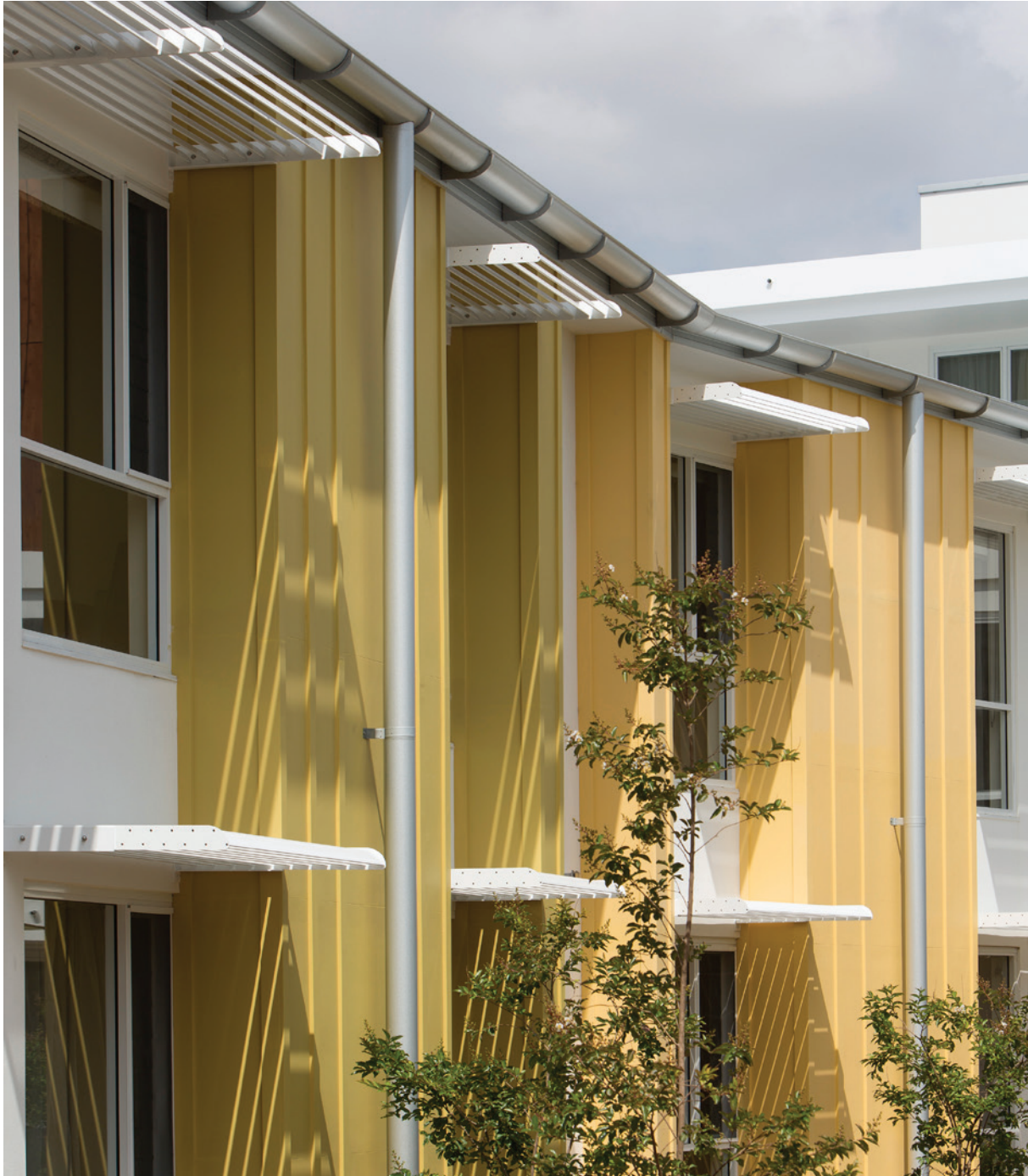
Fig 1.4.B Shading and deeply recessed fenestration articulate the external façade and provide interest with dynamic movement of shadow patterns through the day
