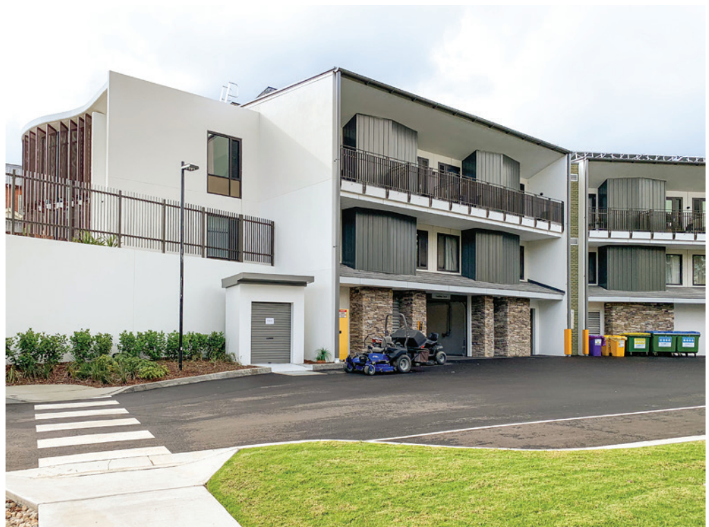
Fig 6.11.A Service driveway showing loading dock area and back-of-house utilities
