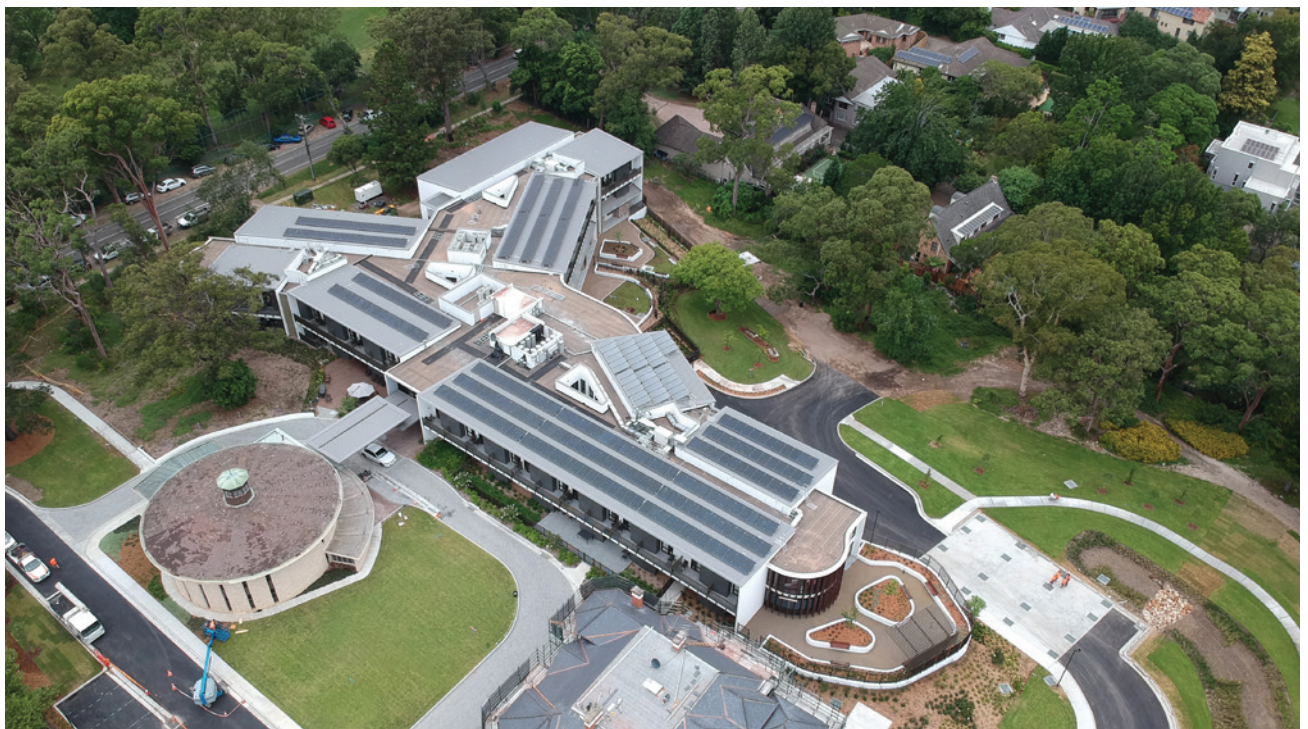
Fig 1.5.A Residential care facility with extensive photovoltaics on the roof
