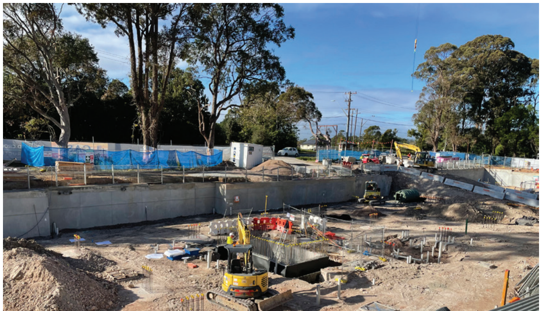
Fig 1.2.A Commencement of construction for a new residential care facility
