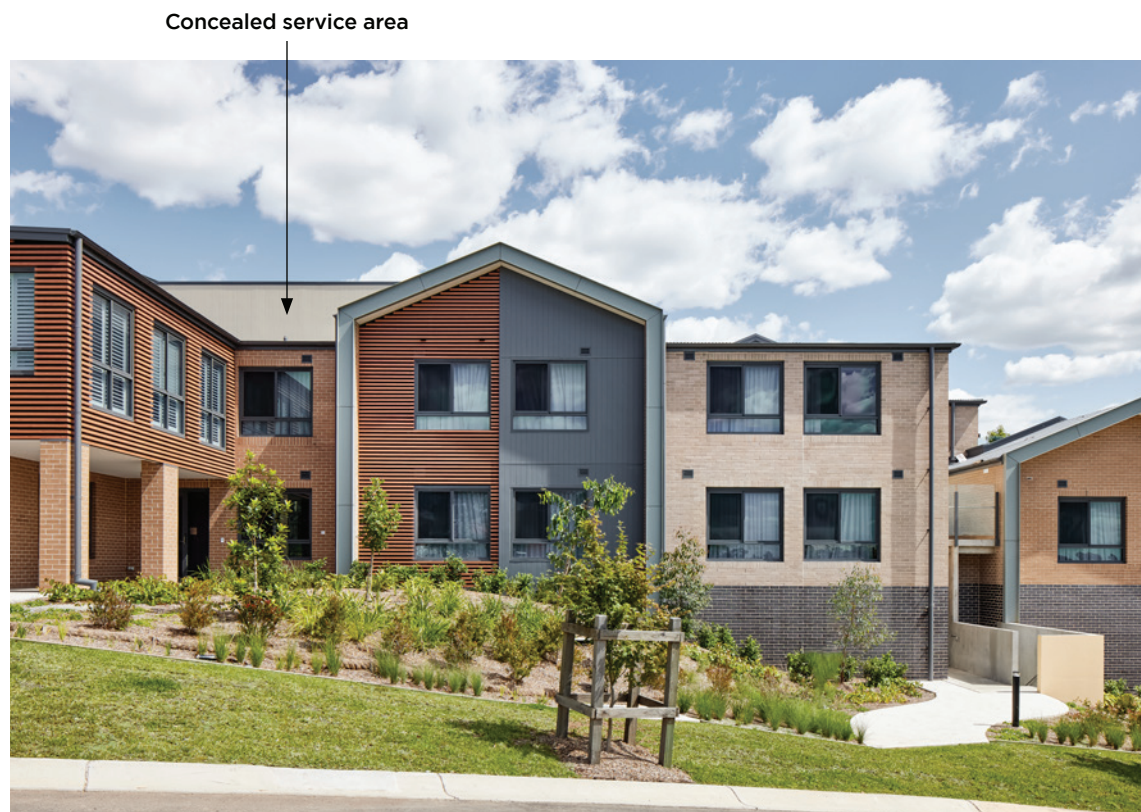
Fig 6.10.D Service plant concealed from view by roof structure
