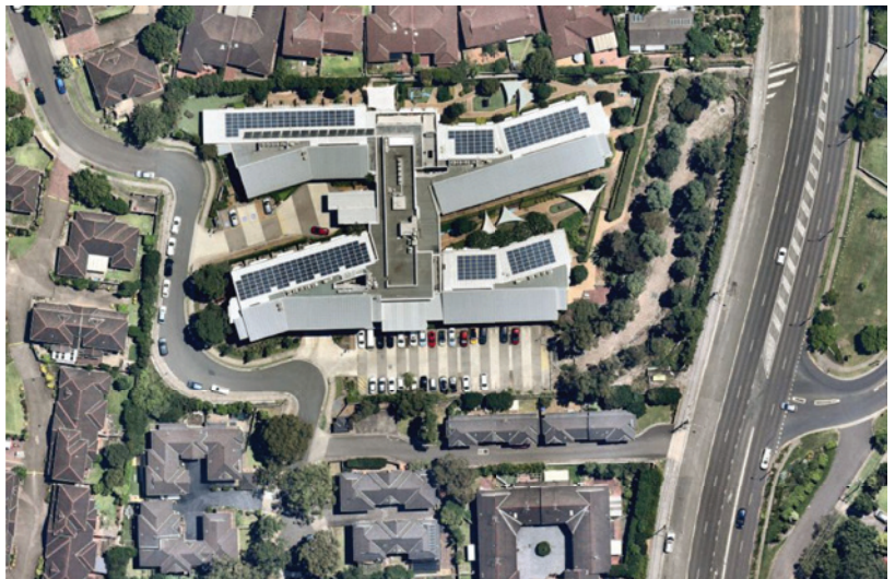
Fig 2.2.D Aerial view of completed development showing dry creek bed to channel stormwater into culvert
