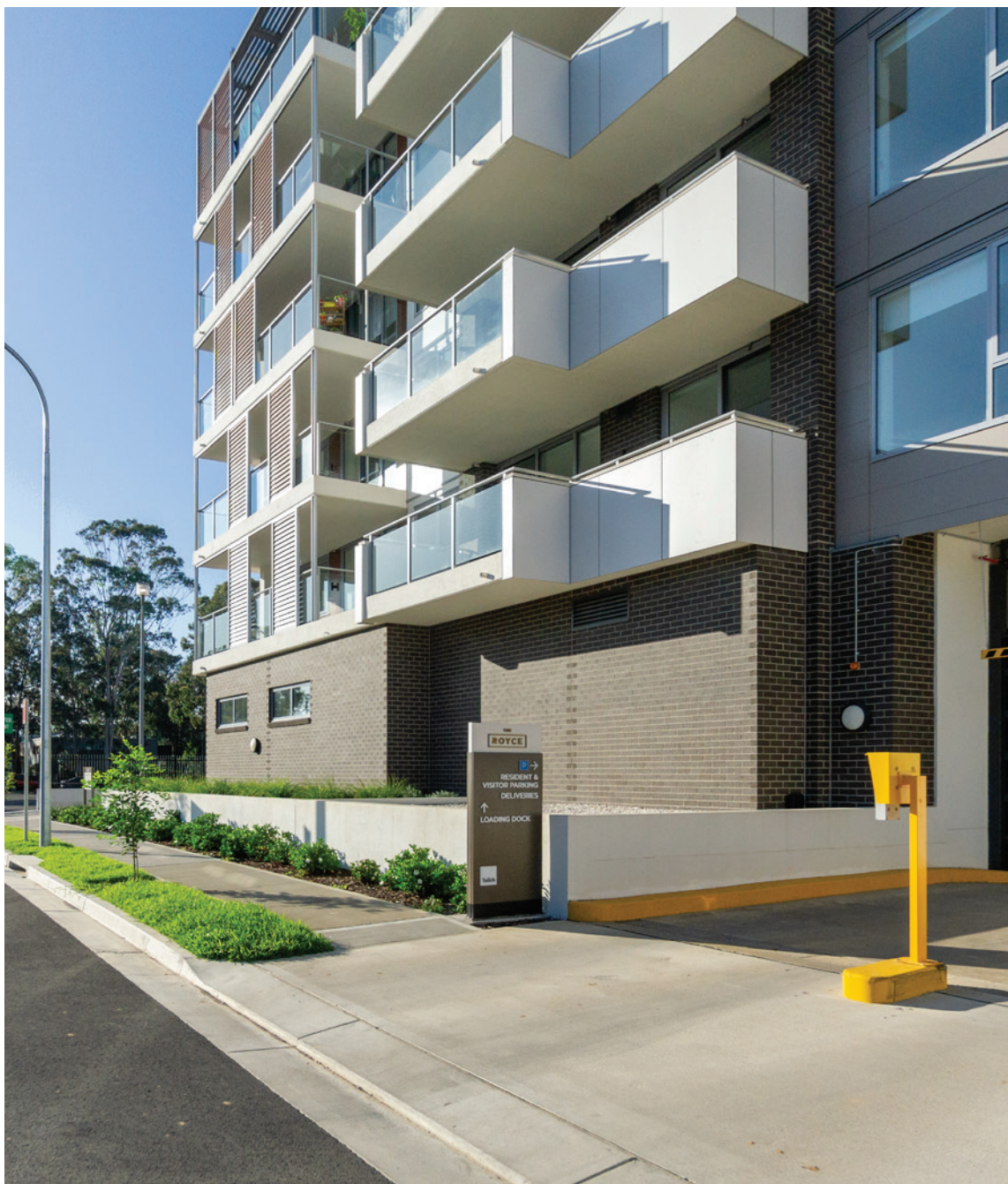
Fig 6.16.C Basement carpark entry with clear signage and level threshold
