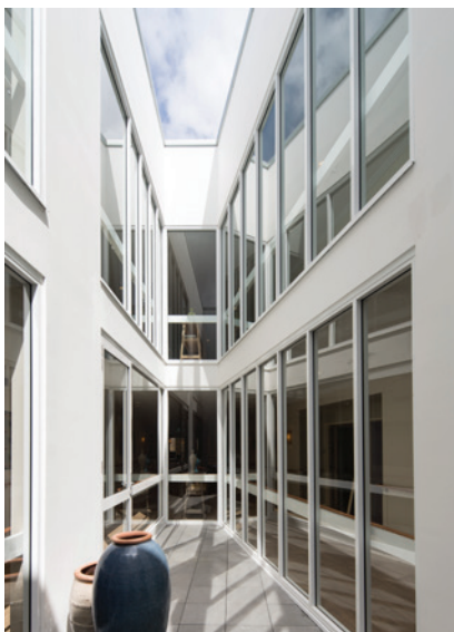
Fig 1.4.A Lightwells bring daylight and variance in light quality through the day into deep parts of the building
