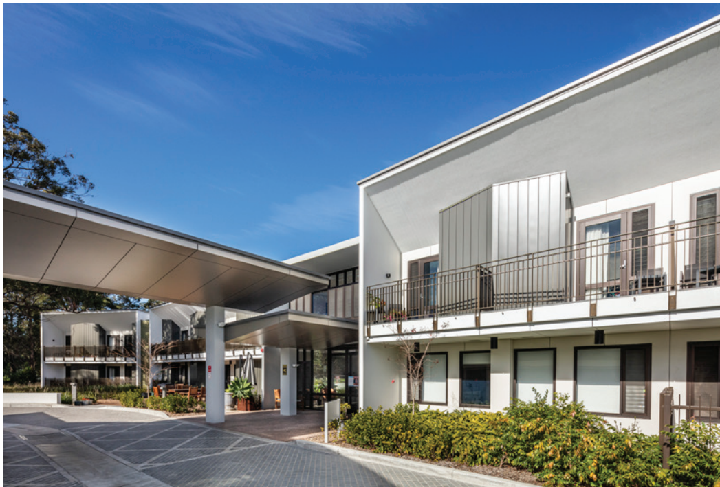
Fig 6.6.A Entry point is identifiable with generous and well-protected roof cover roof cover
