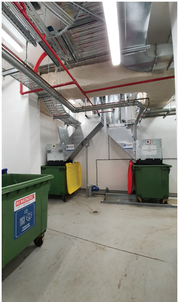
Fig 6.19.A Recycling in basement back-of-house
