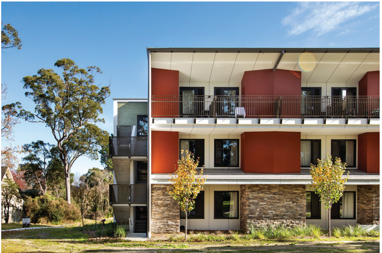
Fig 6.4.A Residential care facility with texture, shadows, recessive elements and colour
