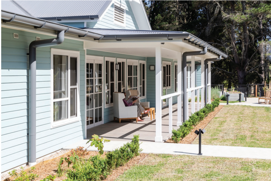
Fig 5.3.G Verandahs offer shade and protected access to the external environment to entice residents outdoor as well as providing familiarity in the Australian context
