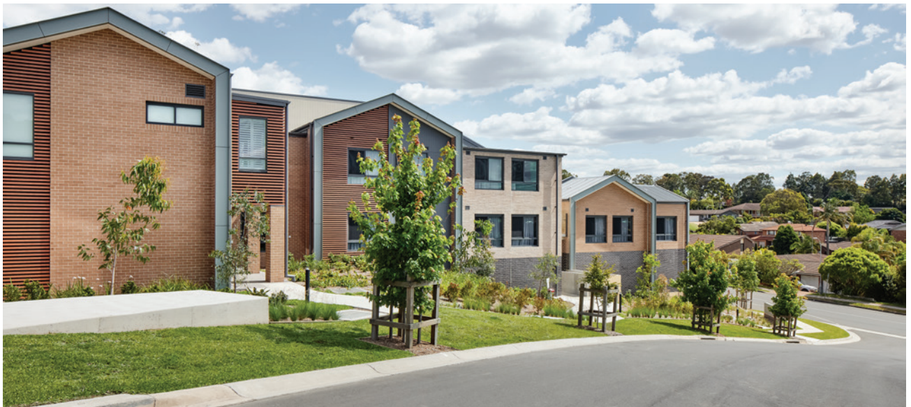
Fig 3.1.A New residential care facility integrates sympathetically with neighbourhood character
