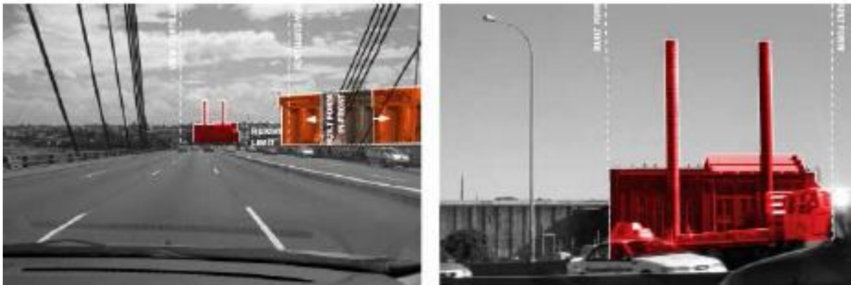
Viewshed from Anzac Bridge as defined in the Heritage Impact Statement (p.80) showing that the view of the existing built elements and the chimneys in particular must be retained. The report notes that “The over-station development will block the northern half Boiler House east elevation and completely block the east elevation of the Coal Handling Shed from Anzac Bridge approach”
