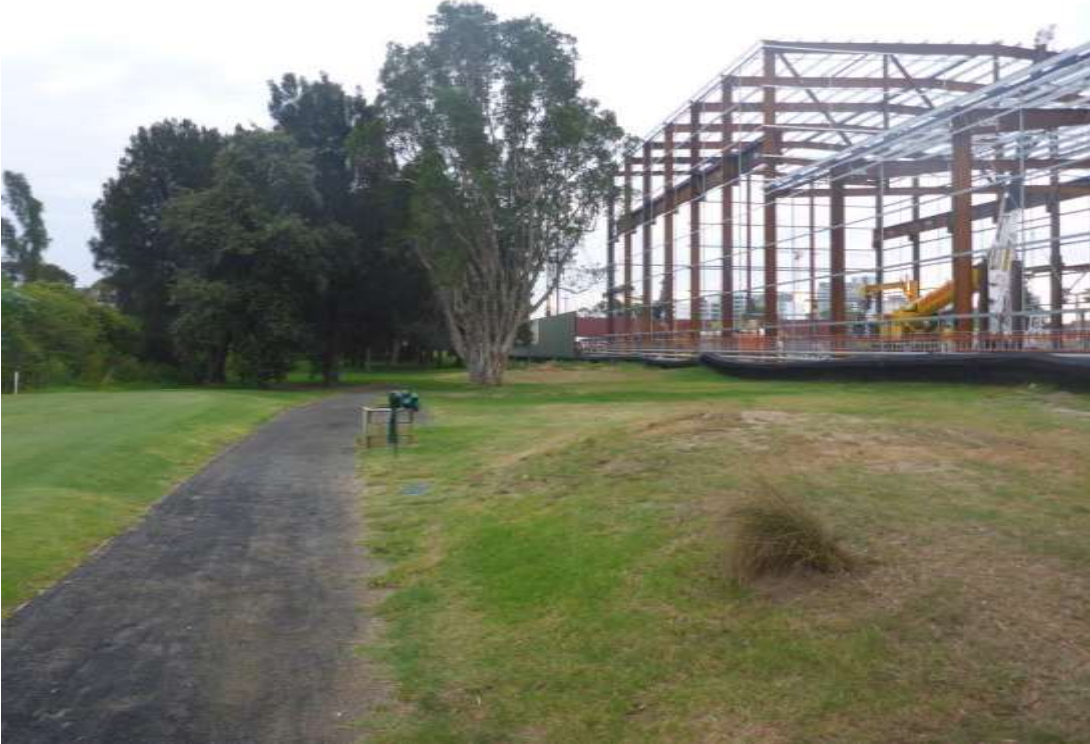
Plate 10 Area adjacent to M5 works, view north-west.
