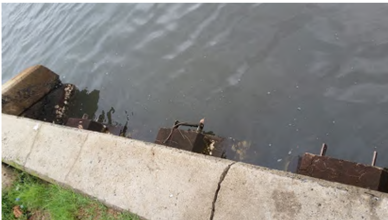
Figure 24: Existing headwall and flap gates at discharge point to the Cooks River north of Marsh Street
