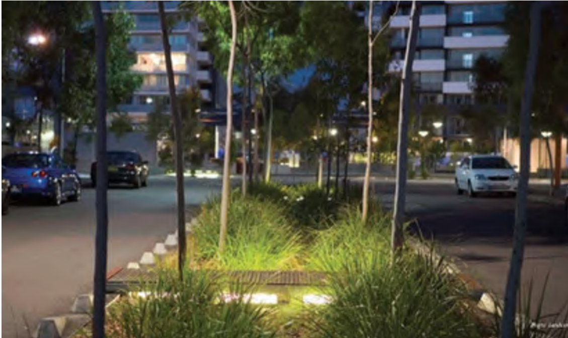
Figure 25: Example central median bioretention swale with broken kerb in Zetland (source: Water by Design, 2009)
