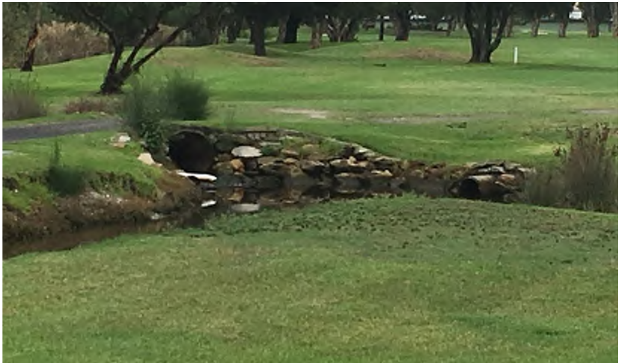
Figure 22: Golf course landscaping incorporating swales culverts (photograph taken on 17/03/2017)
