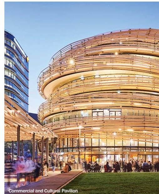
Commercial and Cultural Pavilion
