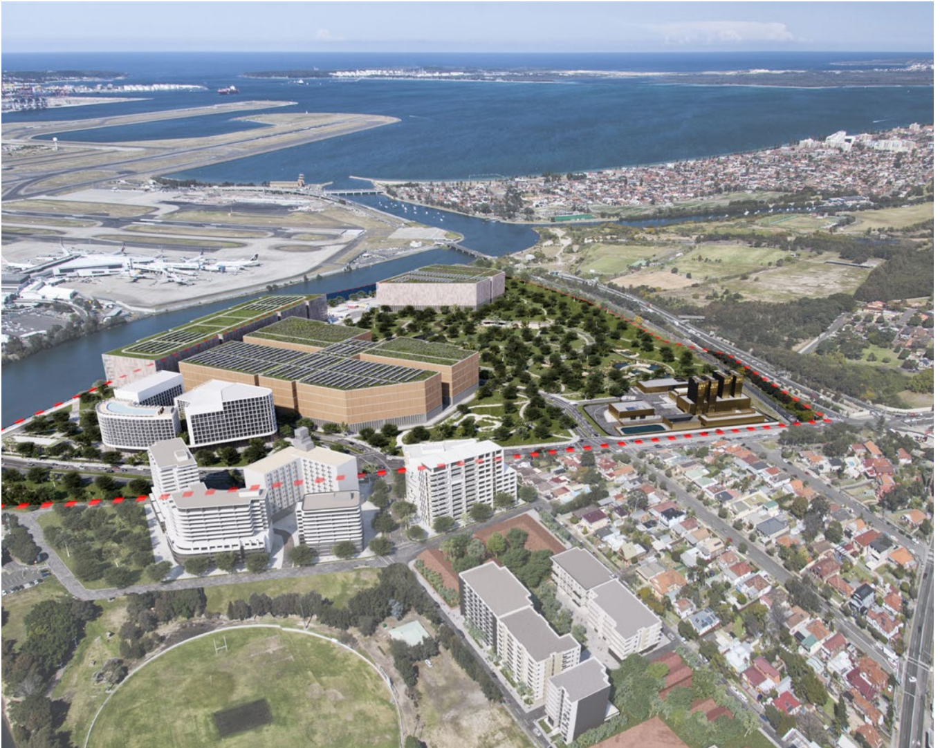
Figure 1: Cooks Cove indicative reference scheme – as viewed towards Sydney Airport and Botany Bay
