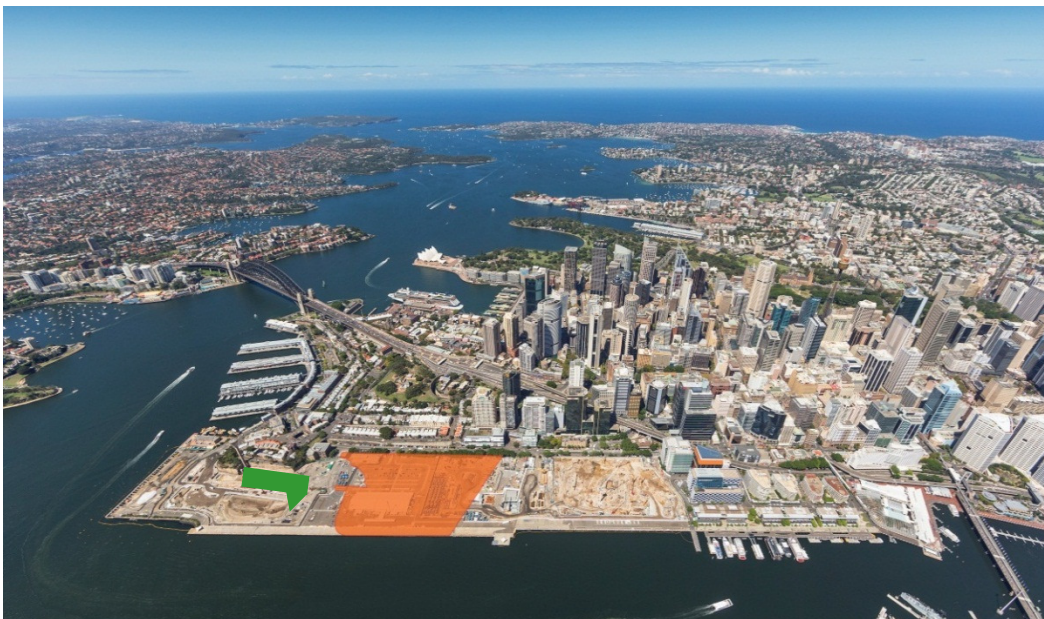
Figure 3: Aerial showing Central Barangaroo and Headland Park Cultural Facility Space
