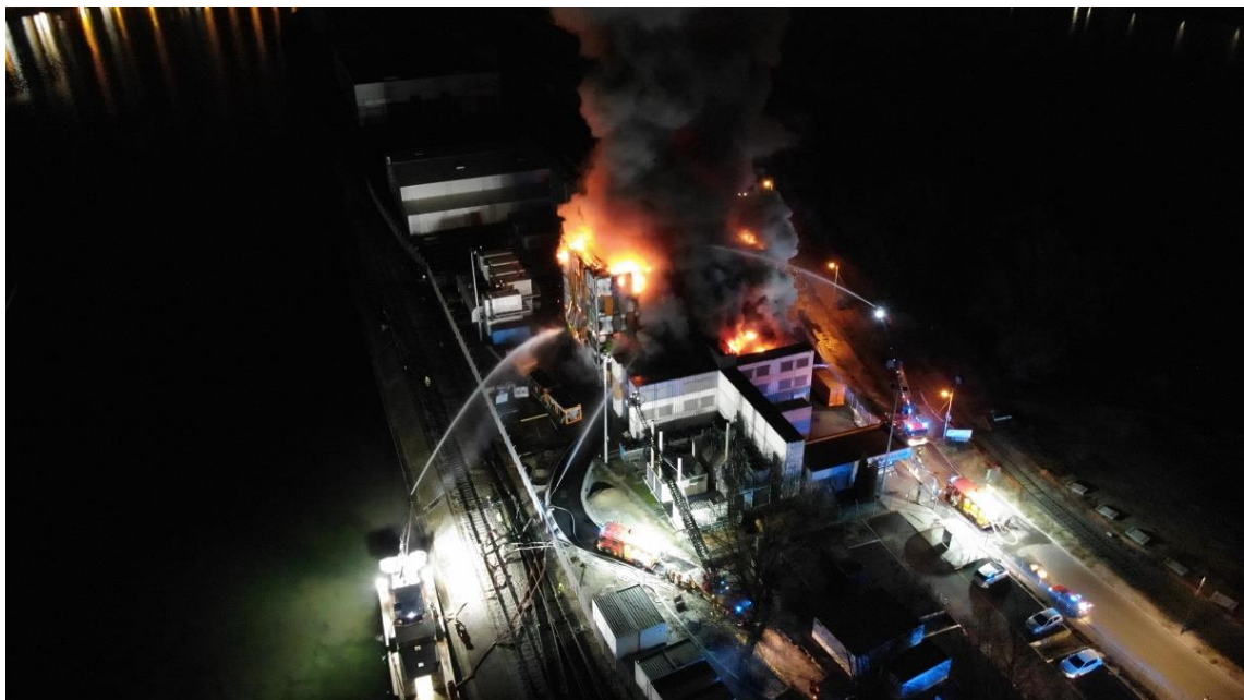
Figure 8.1: OVH data centre fire (March 2021)
