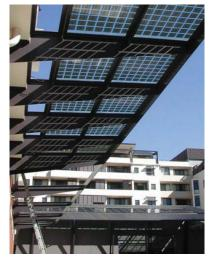
Figure 8C.1-3: Photovoltaic cells integrated into the awning design.
