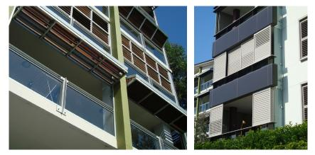
Figure 23.4-3: Louvres and sliding panels as an integrated facade element.
