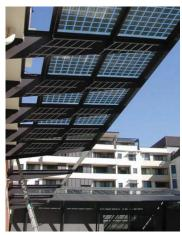
Figure 8C.9-3: Photovoltaic cells integrated into the awning design.
