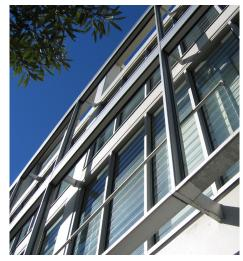
Figure 8C1-2: Retractable shading devices to the windows for solar access control.
