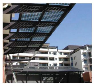
Figure 23.2-1: Photovoltaic cells integrated into the awning design.
