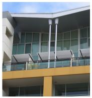
Figure 8C.9-4: Drainage pipes integrated with the overall facade design.
