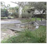
Figure 24C.6 -2 A local raingarden connected to the overflow of a rainwater tank improves water quality and reduces runoff to the adjoining bushland.
