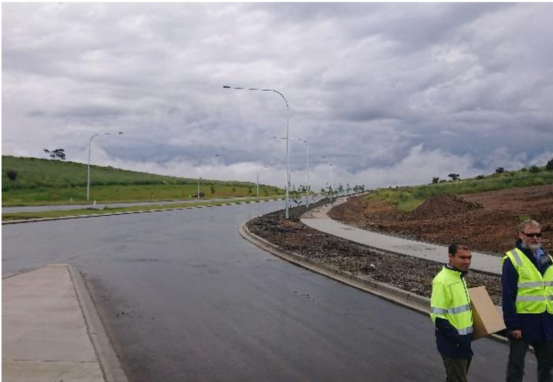
Figure 2-7 | Image 3 - Looking north from the site of the Innovation Hub
