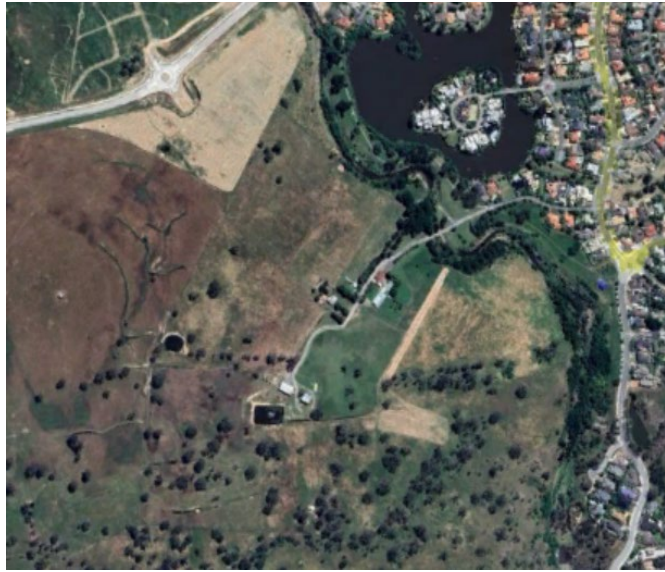
Photograph 10.14 Private property (east) (Google Earth 2022)
