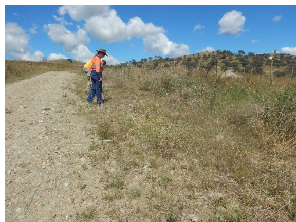
Figure 8.23 Assessing scours along dirt tracks in SU8
