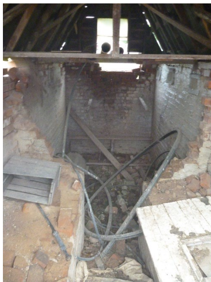
Photograph 10.7: Internal view of semi-underground dairy (ERM 2022)
