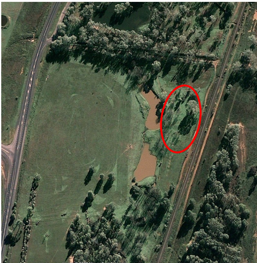
Photograph 11.4: Historical aerial c~2010 showing the demolition of former structures at Ettamogah Vineyard Ruins
