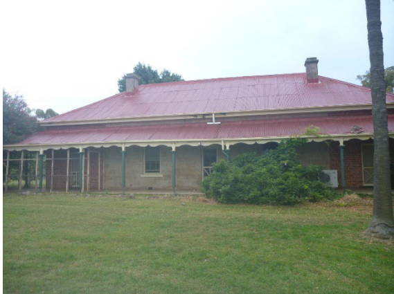
Photograph 10.1: View of front of main homestead (ERM 2022)
