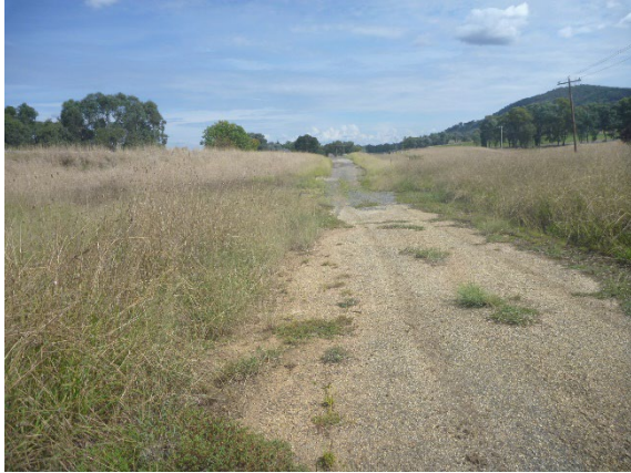
Photograph 10.14: View of remnant road surface towards continuation of Wagga Road
