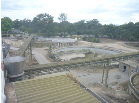
Photograph 8.13: View south towards Eight Mile Creek showing substantial earthworks associated with existing paper mill (ERM 2022)
