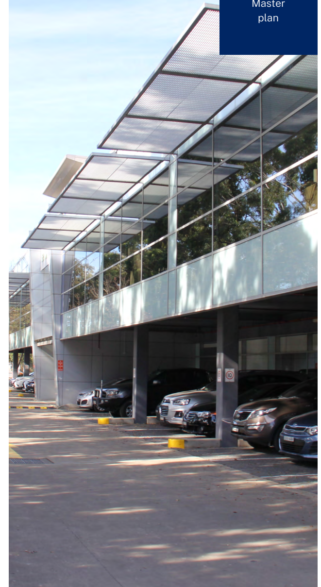
Commercial buildings in Camellia–Rosehill
