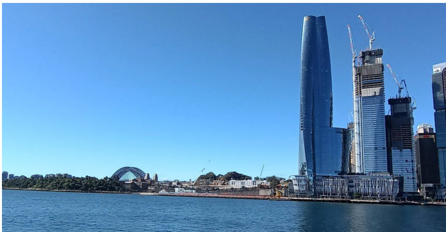
Figure 6: View of the subject site from Pyrmont
