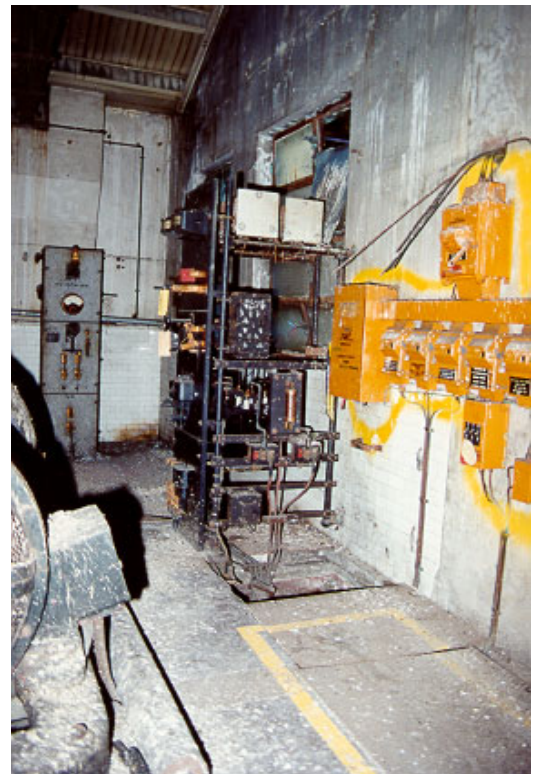
Figure 3.9 The former control room. Motor Generator Set 2 is located in the left side of this view. The motor generator Set 2 switchboard, one of the oldest in the power station, is located in the background on the right hand side. Other switchboards also part of the Power Reticulation System are located on the left hand side.
