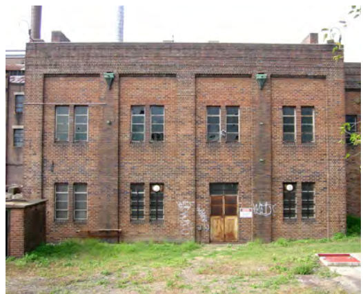
Figure 2.1.2.5 Control Room from the west (Design 5 - Architects)
