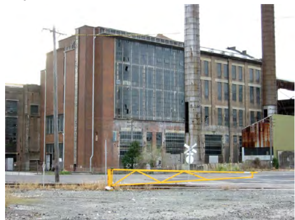
Figure 2.1.2.2 Boiler House #1 from the south east (Design 5 - Architects)
