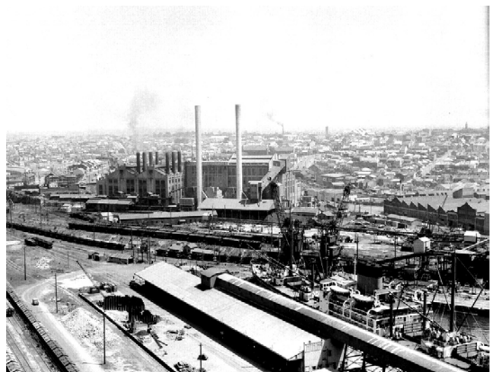
Figure 2.6.6.1 White Bay Power Station and the White Bay Hotel (left of picture) from the tops of the Glebe Island Wheat Silos about 1960. (Collection of Pacific Power)
