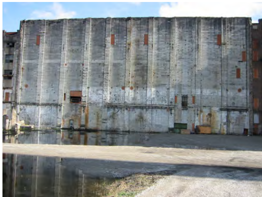
Figure 2.1.1.8 Site of Boiler House No. 2 (Design 5 - Architects)
