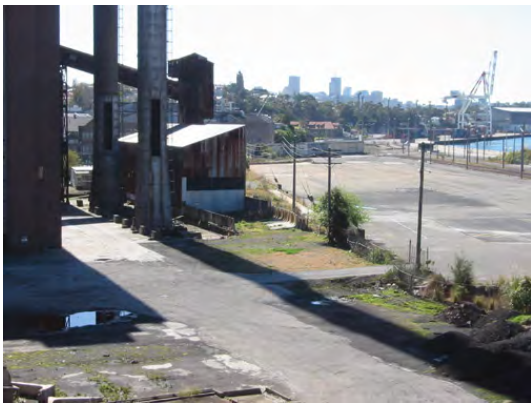
Figure 2.1.1.2 Coal Yard (Design 5 - Architects)
