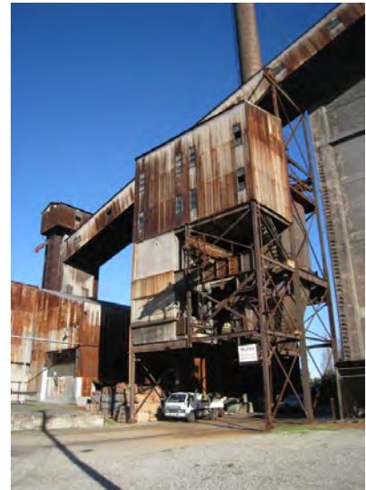
Figure 5.1.2.2.1 Coal Handling Shed and Conveyor (Design 5 - Architects)
