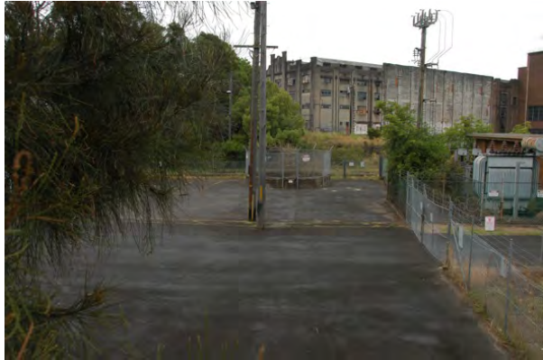
Figure 2.1.1.1 The southern Penstock in State Rail land (Design 5 - Architects)
