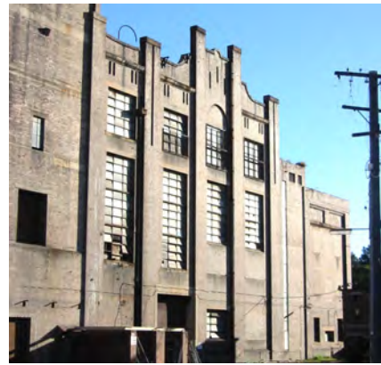
Figure 2.1.2.3 Turbine Hall from the north (Design 5 - Architects)
