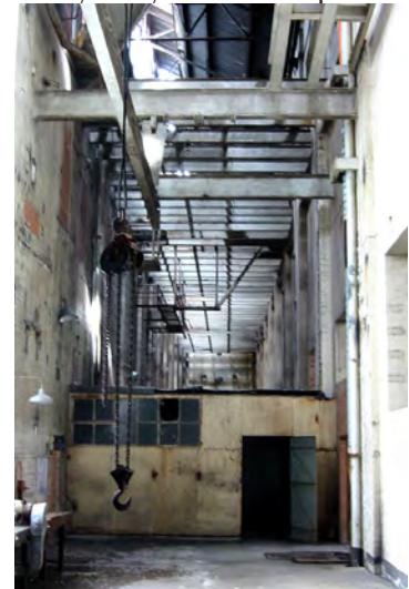
Figure 3.2.2.3 Pump House (Design 5 - Architects)
