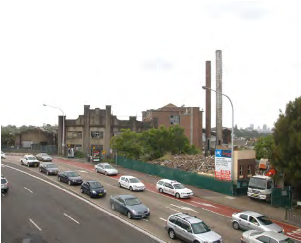
Figure 2.1.0.4 Southern Elevation, viewed from overpass (Design 5 - Architects)
