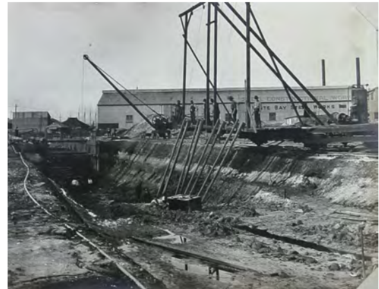
Figure 2.6.2.3 WBPS Site during Construction 1912 (courtesy PowerHouse Museum archive)
