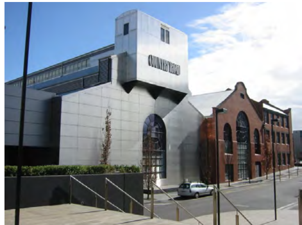
Figure 2.7.3.2 Former Richmond Power Station
