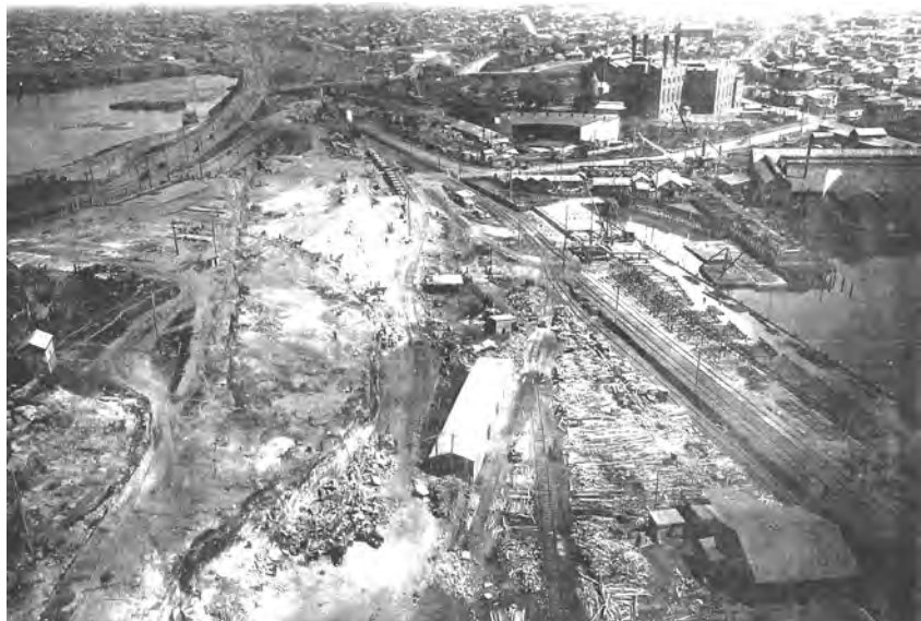
Figure 2.6.1.6 View of the quarrying of Glebe Island for the Wheat Silos - but interestingly showing White Bay Power Station at the completion of Stage 1. The first boiler house is complete and half of the Turbine Hall and Switch House. Note the road to the right of the Power Station which appears in the Parish map of 1886 (amended up to 1899). The shed by the wharf must be standing on Sydney Harbour Trust land. The White Bay Hotel can be seen as a solitary building at the southern end of the Power Station site.
