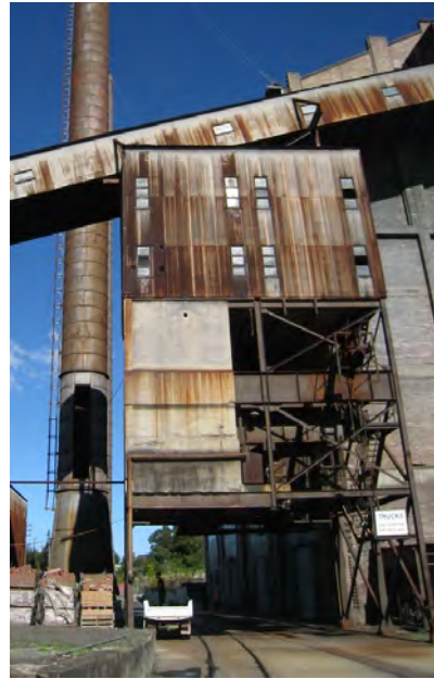
Figure 2.1.1.7 Ash Handling Unit (Design 5 - Architects)
