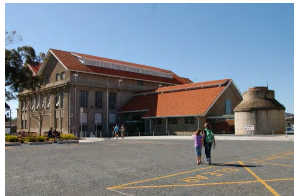
Figure 2.7.3.1 Canberra Glass Works (Design 5 – Architects, 2010)
