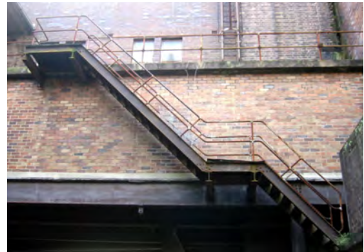
Figure 5.3.7.1 Walkways and Handrails (Design 5 - Architects)
