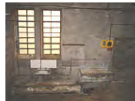
1948 Switch House ground level south end
