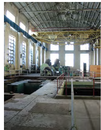
Figure 5.1.8.1 Turbine Hall Interior (Design 5 - Architects)
