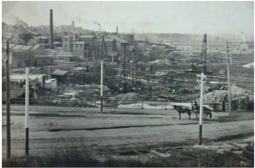
Figure 2.6.1.5 Early photograph of work commencing on the site of the White Bay Power Station. (courtesy of PowerHouse Museum archive)
