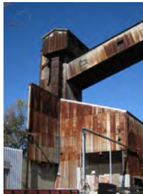
Coal Handling Tower
