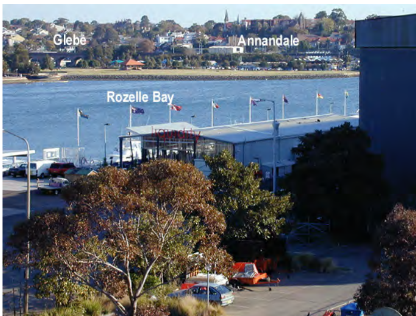
Figure 5.7.4.5 Rozelle Bay viewed from the north (Source unknown)
