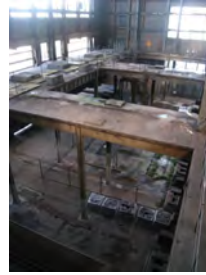
Boiler House floor - spaces formerly occupied by Boilers 2, 3 and 4
