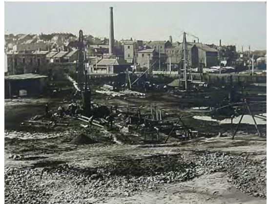
Figure 2.6.2.1 WBPS Site during Construction 1912 (courtesy PowerHouse Museum archive)
