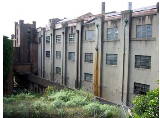
Figure 2.1.2.4 Switch House from the west (Design 5 - Architects)
