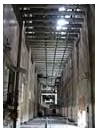
Pump House south end
