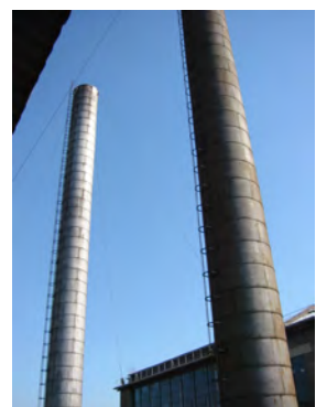
Figure 5.1.6.1 Chimneys (Design 5 - Architects)
