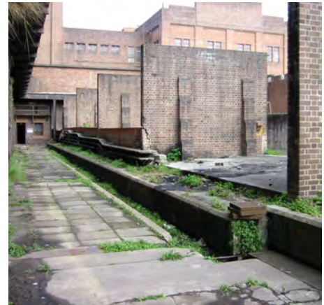
Figure 5.1.11.2 Transformer Yard (Design 5 - Architects)
