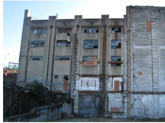
Figure 2.1.1.19 Admin & Staff Accommodation from the east (Design 5 - Architects)
