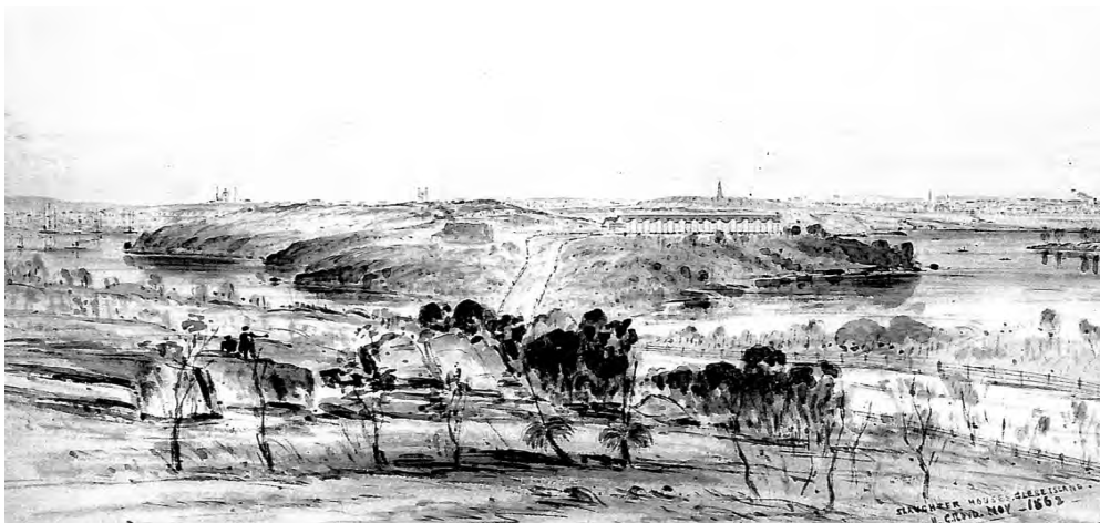
Figure 2.6.1.1 Watercolour drawing entitled 'Slaughterhouses. Glebe Island. H.G.Lloyd 1863' The White Bay Power Station site would be to the left of the road leading towards Glebe Island.
