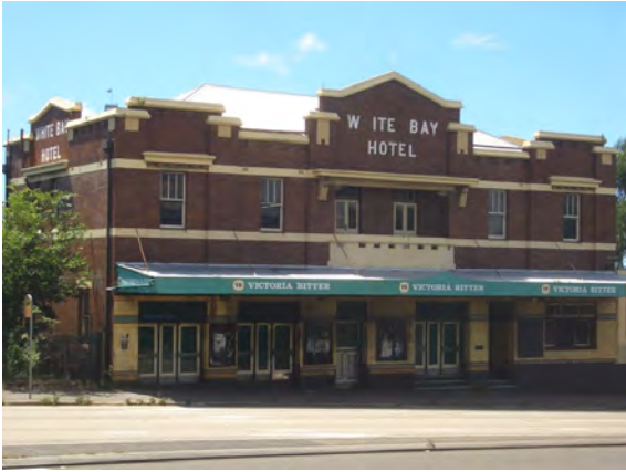
Figure 2.6.9.5 White Bay Hotel front elevation, 26 January 2008 (Photographer: J Bar, Available through Wikimedia Commons, file: White Bay Hotel.jpg)
