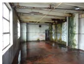
Former locker room level 2, Admin Building
