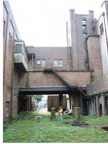
Figure 2.1.1.13 South Transformer Yard looking north (Design 5 - Architects)
