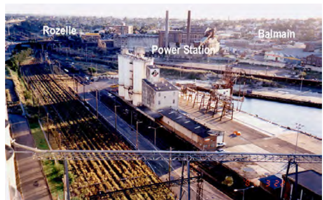
Figure 5.7.4.2 The power station viewed from on top of the Glebe Island grain silos (Source unknown)
