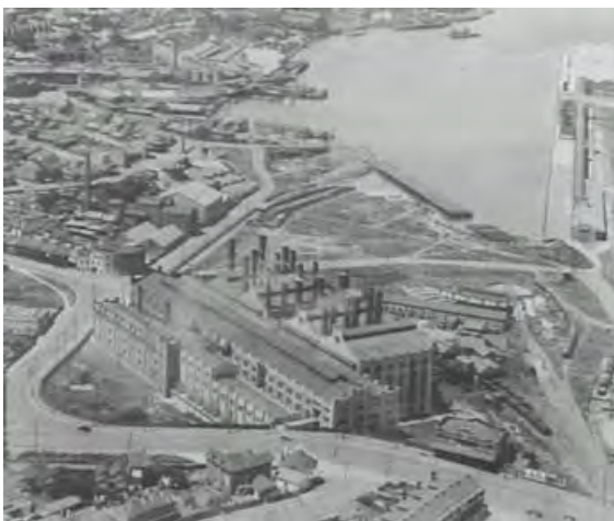
Figure 2.6.9.3 Aerial, c 1930 of the White Bay Power Station including White Bay Hotel in the bottom right corner.
