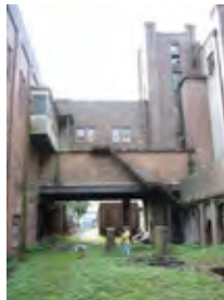
South-west Transformer Yard
