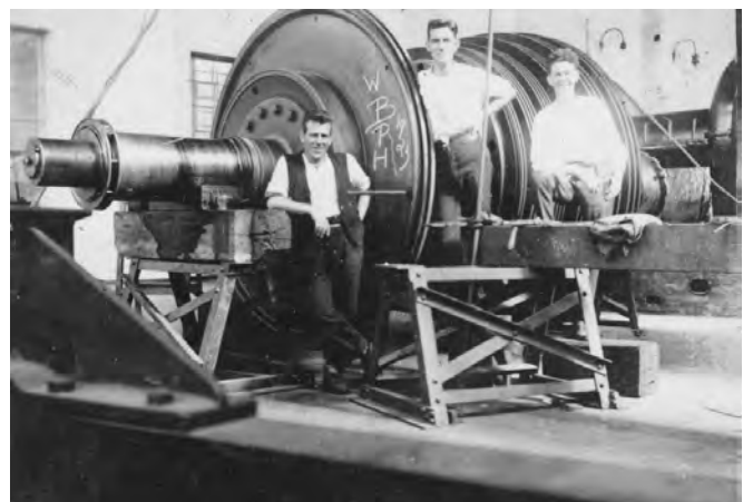
Figure 2.6.4.4 White Bay Power Station 1923. Installation of turbine rotor during the 2nd phase of development. (courtesy PowerHouse Museum archive)
