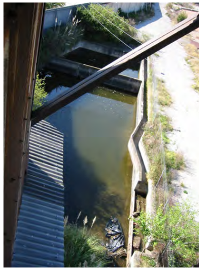
Figure 2.1.1.3 Coal wash pit (Design 5 - Architects)
