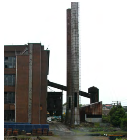
Figure 3.2.1.4 View north from railway cutting (Design 5 - Architects)
