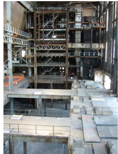
Figure 2.5.1 Interior of Boiler House (Design 5 - Architects)
