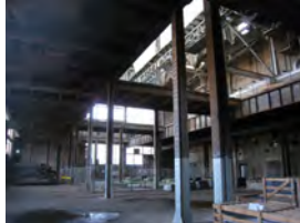
Boiler House – spaces formerly occupied by Boilers 2, 3 and 4
