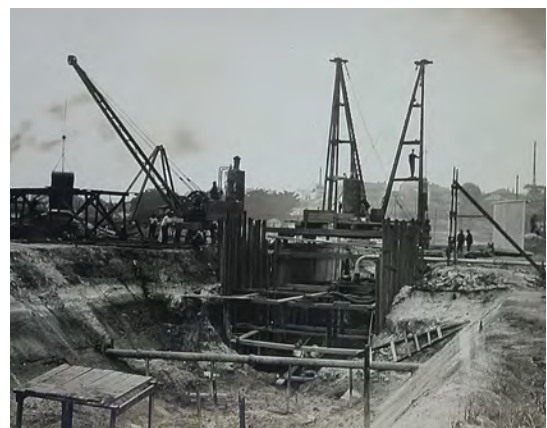
Figure 2.6.2.2 WBPS Site during Construction 1912 (courtesy PowerHouse Museum archive)
