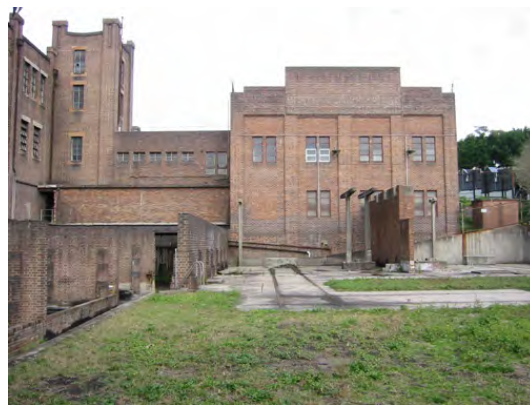
Figure 2.1.1.14 North West Yard looking towards 1948 Control Room (Design 5 - Architects)
