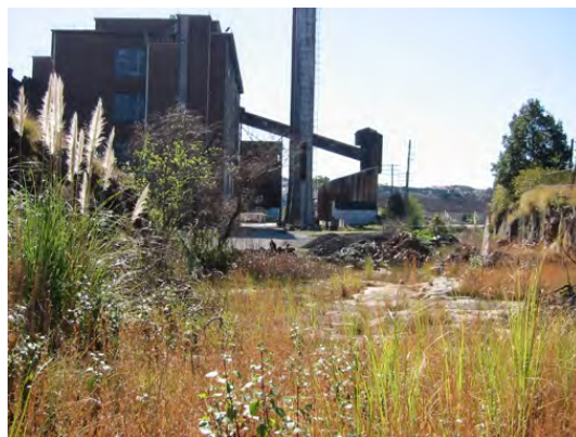
Figure 2.1.1.5 View north from railway cutting (Design 5 - Architects)
