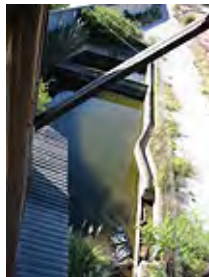
Coal Wash tank
