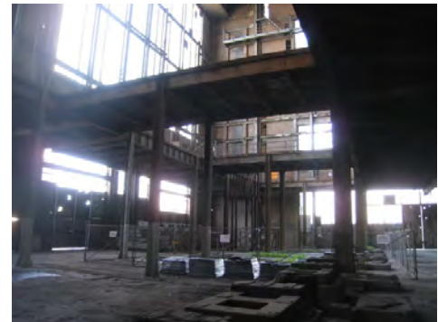
Figure 5.1.7.1 Boiler House Void (Design 5 - Architects)
