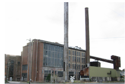
Boiler House and Stacks (Design 5 - Architects)
