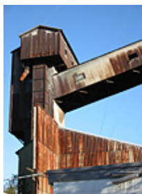
Coal Handling Tower
