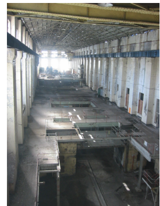
Turbine Hall (Design 5 - Architects)
