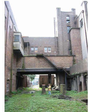
SW Transformer Yard (Design 5 - Architects)
