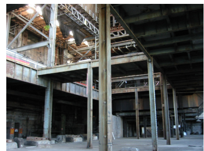
Boiler House (Design 5 - Architects)
