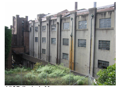
1927 Switch House (Design 5 - Architects)
