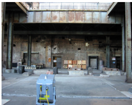
Added raised concrete plinth in 1958 Boiler House
