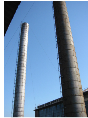
Chimney Stacks (Design 5 - Architects)
