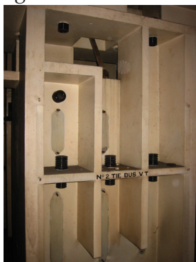
Bus Bar Enclosures (Design 5 - Architects)
