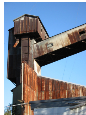
Coal Elevator (Design 5 - Architects)
