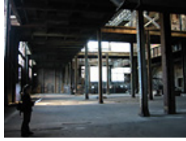
Boiler House – spaces formerly occupied by Boilers 2, 3 and 4
