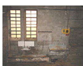
1948 Switch House ground level
