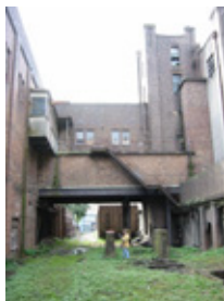
South-west Transformer Yard
