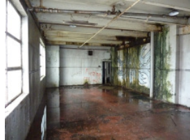
Former locker room level 2, Admin Building
