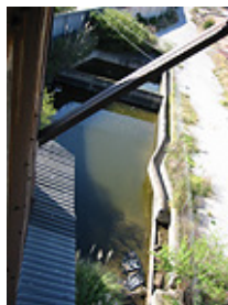
Coal Wash tank
