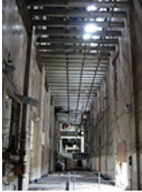
Pump House south end
