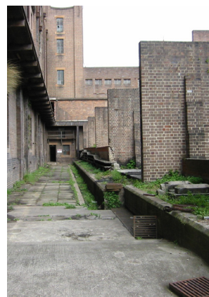
NW Transformer Yard (Design 5 - Architects)
