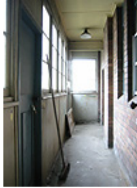
1948 Switch House corridor top level
