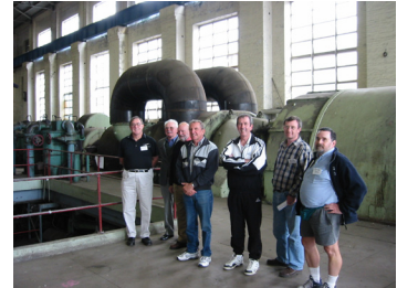
No. 1 Turbine and former Employees (Design 5 - Architects)
