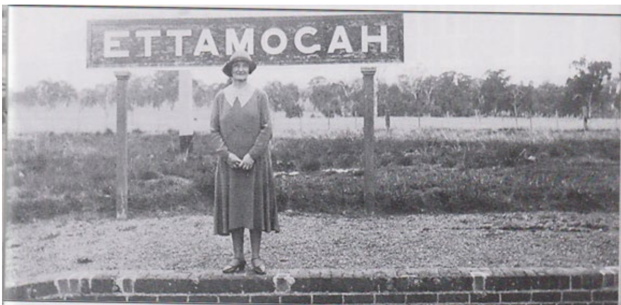
Photograph 7.5 Ettamogah Railway Station, circa 1930s
