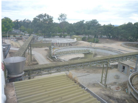
Photograph 8.13: View south towards Eight Mile Creek showing substantial earthworks associated with existing paper mill (ERM 2022)
