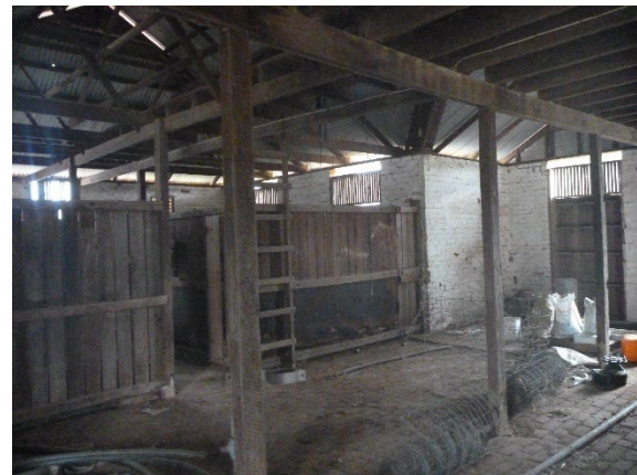
Photograph 10.4: Internal view of stable showing timber supports and internal structures (ERM 2022)
