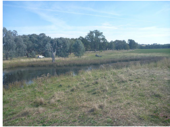
Photograph 8.22: Dam infrastructure associated with localised areas of exposure (ERM 2022)
