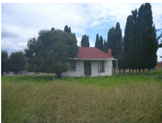
Photograph 10.5: View of front of worker's cottage (ERM 2022)
