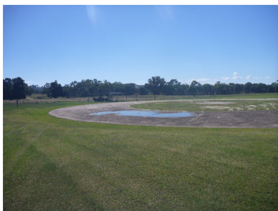
Photograph 8.7: Concrete pad and shade structures associated with the Aeroclub (ERM 2022)
